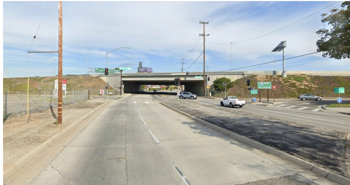
Existing Main St
