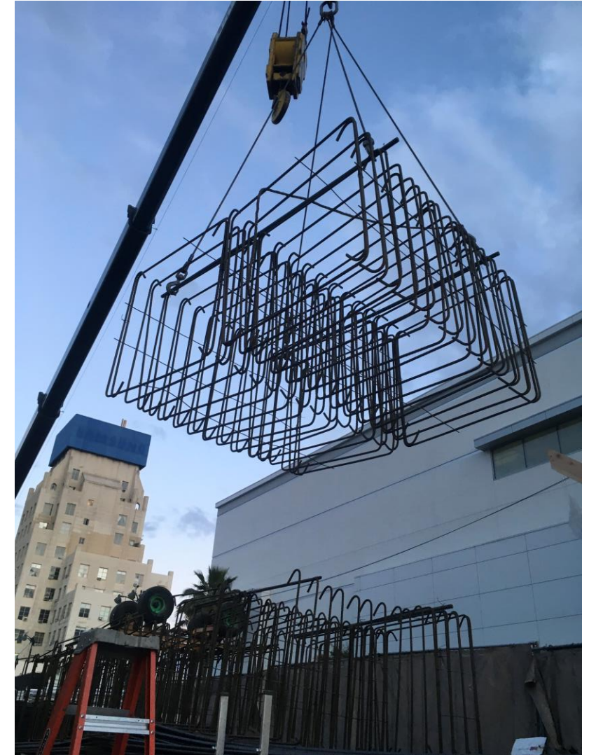
Structural Rebar – Wilshire/La Brea
