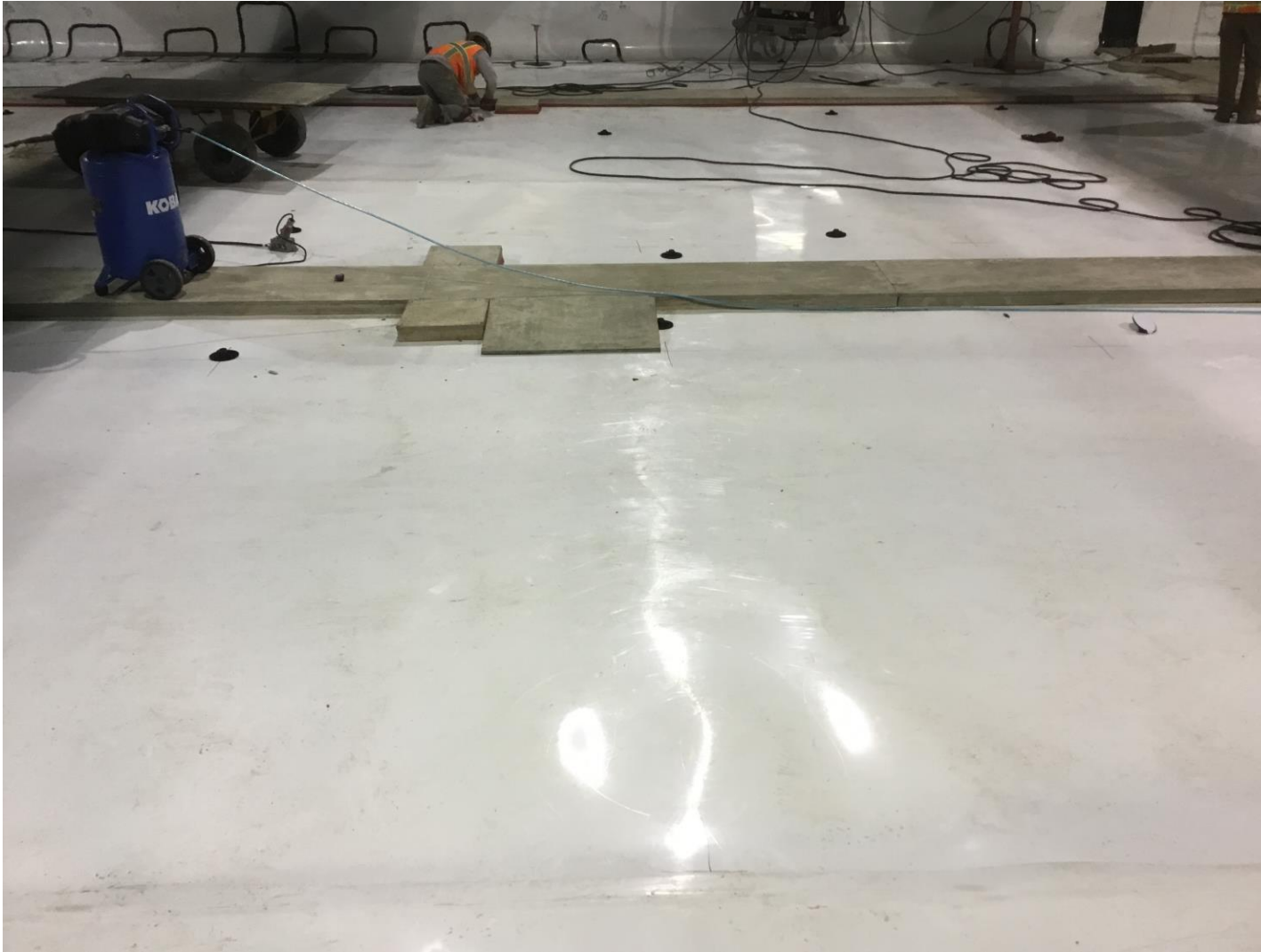
HDPE Placement – Wilshire/Fairfax
