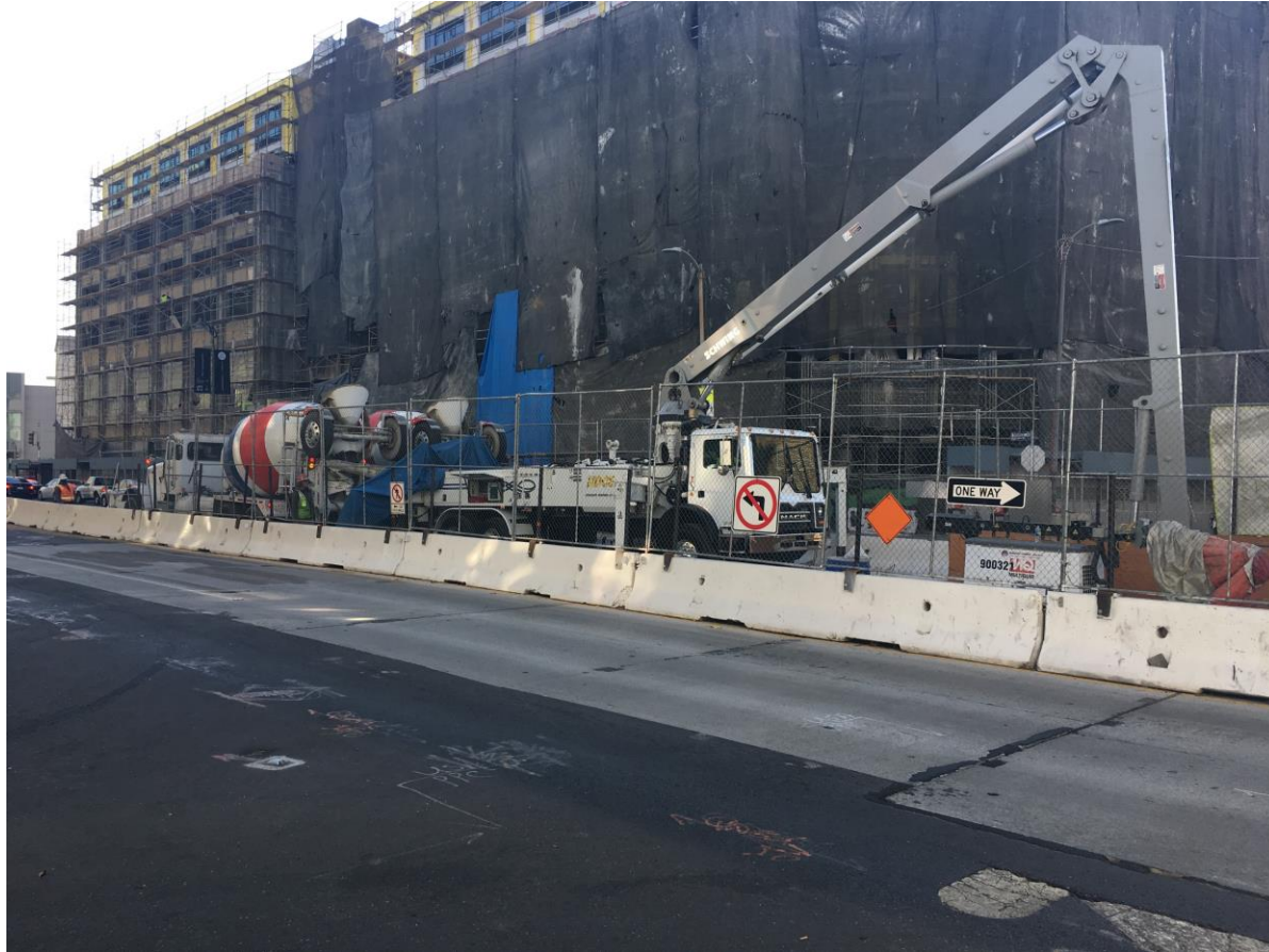
Center Muck Shaft – Wilshire/La Brea
