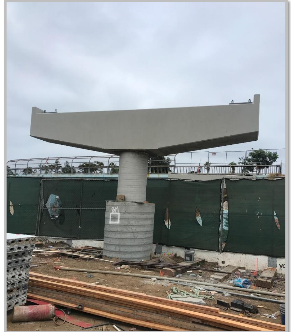
Pedestrian bridge support cap completed, facing North. (August 2026)
