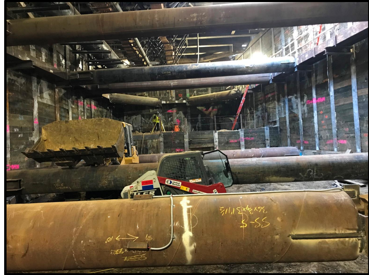
Excavation support system installed, facing East. (August 2026)
