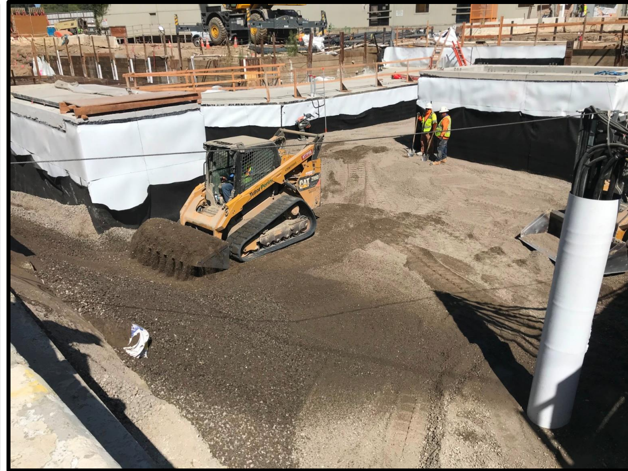
Backfilling operations above the main entrance roof, facing Northwest. (August 2026)
