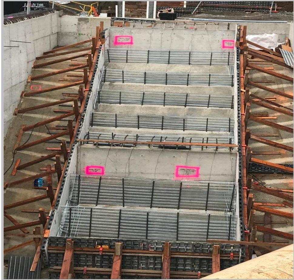
Formwork and rebar installation for stairs at main entrance, facing West. (September 2026)
