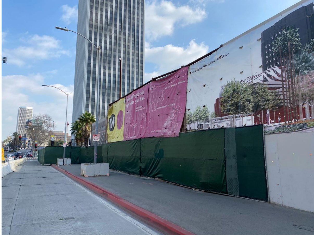
Wilshire/Fairfax Appendage Work
