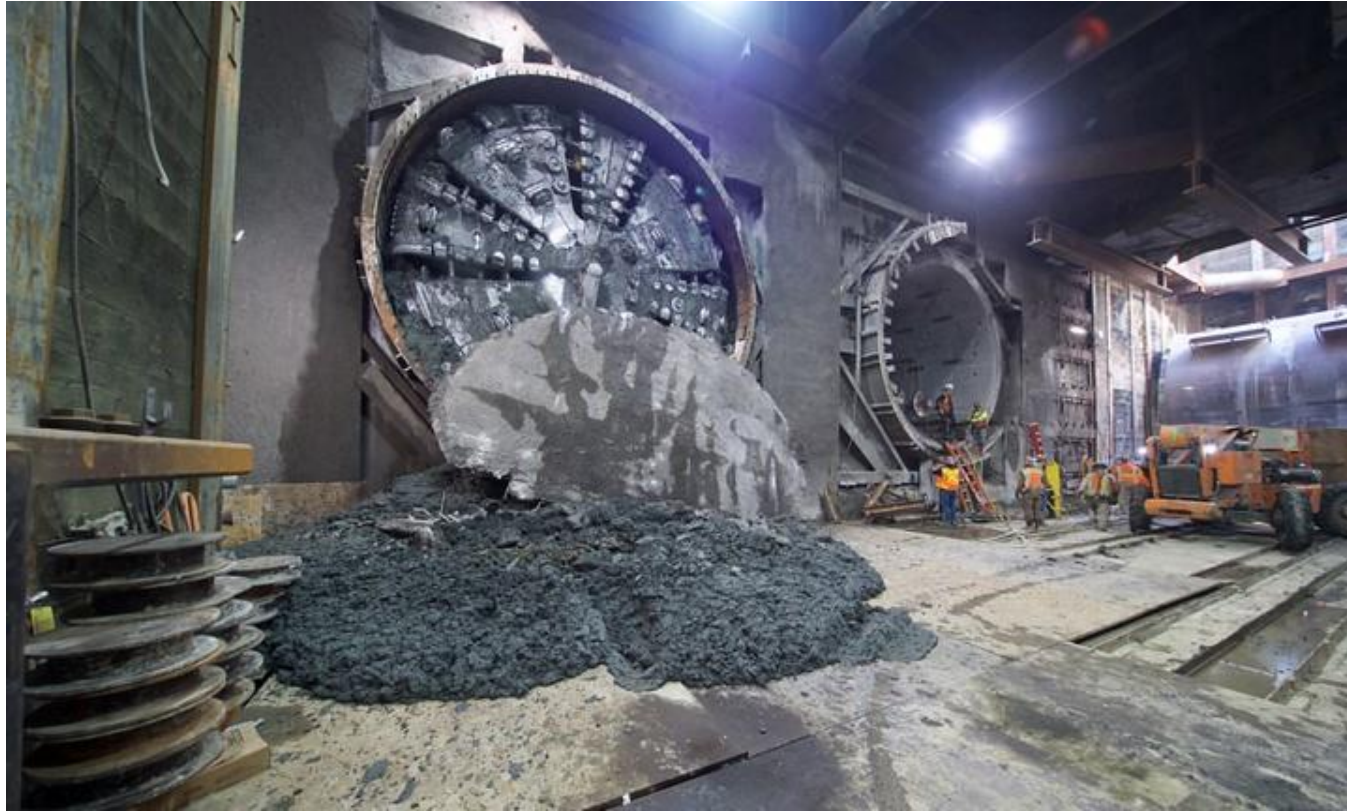
TBM Breakthrough
