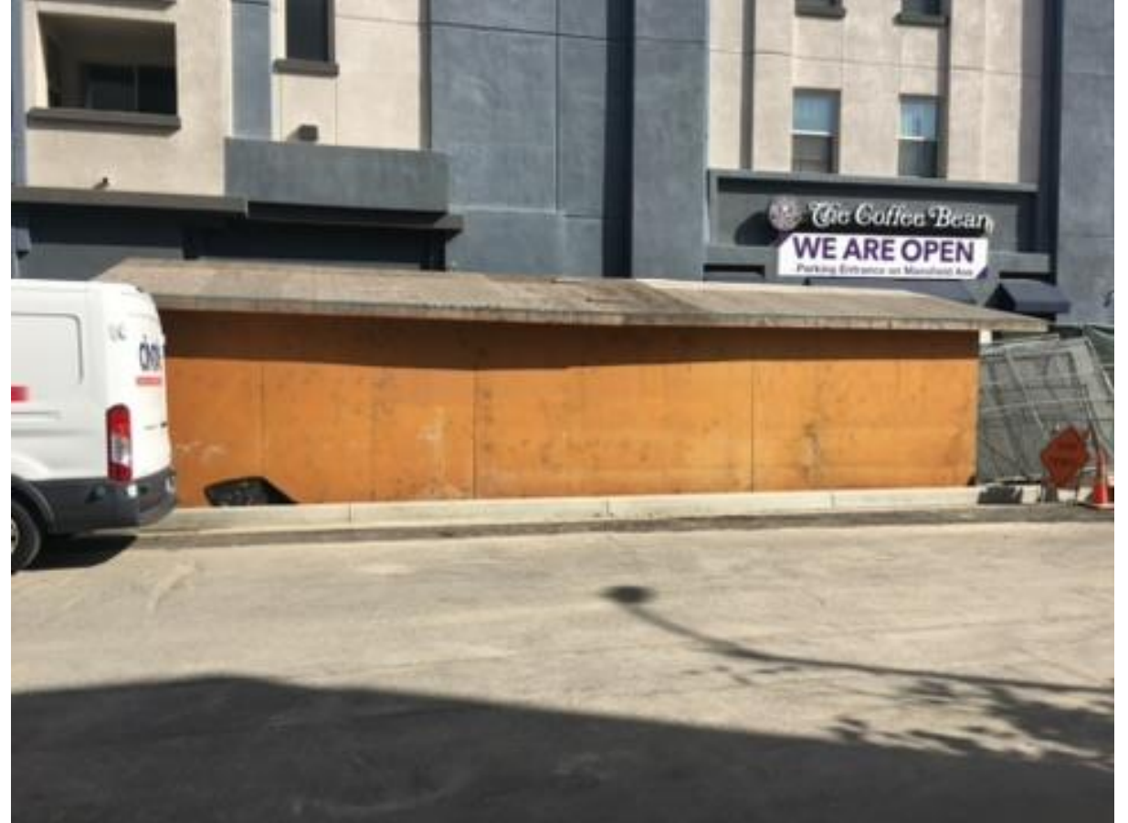
Wilshire/La Brea Appendage Work
