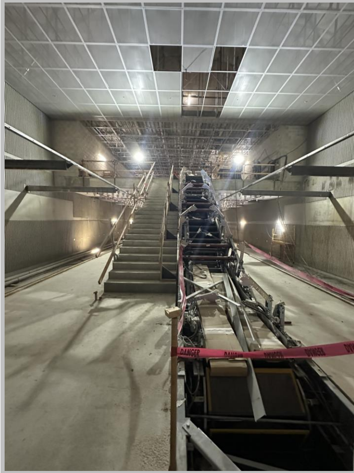
Escalators frame safety guards and brackets installed, facing West. (July 2026)
