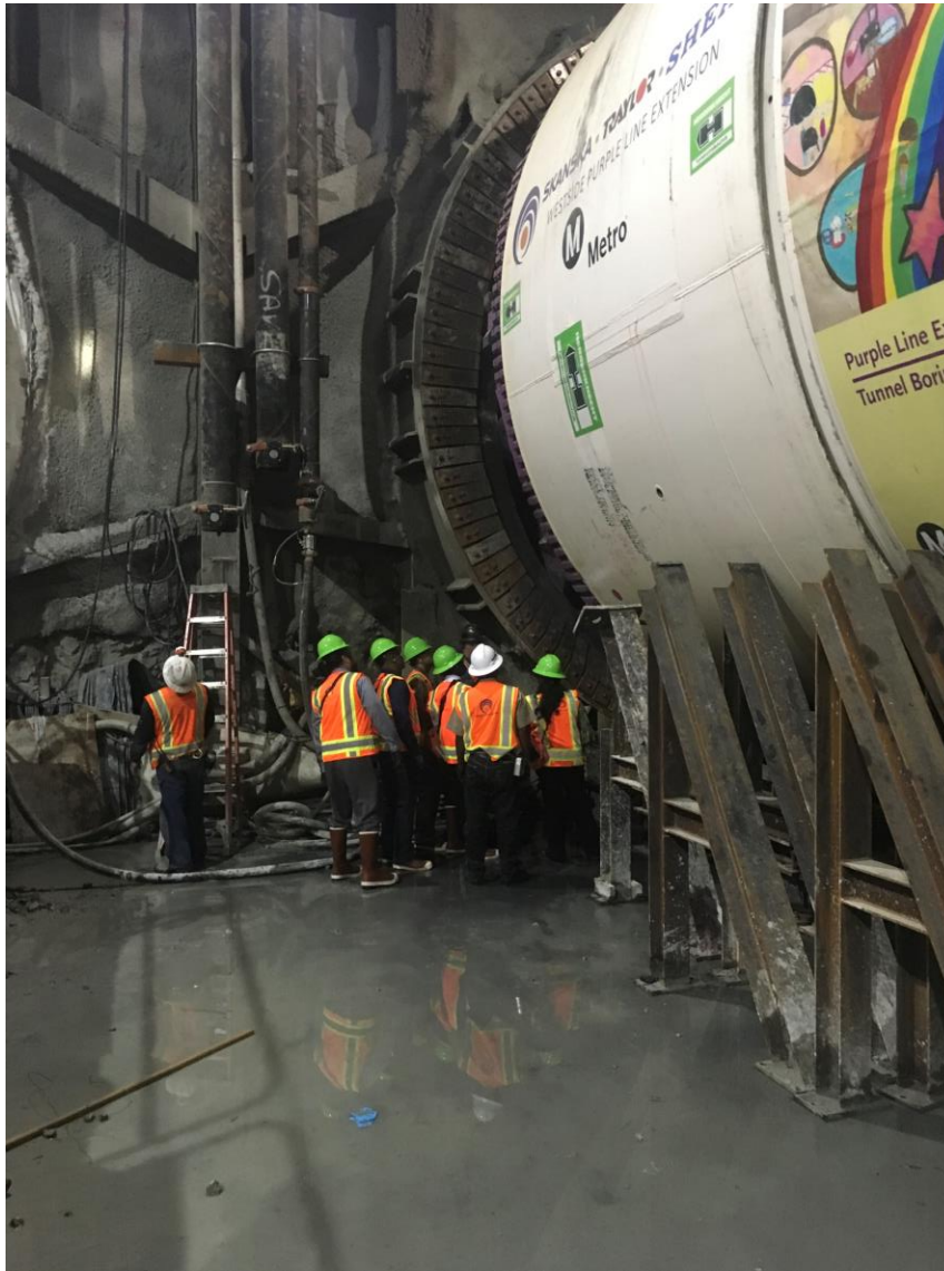
TBM – Facing West
