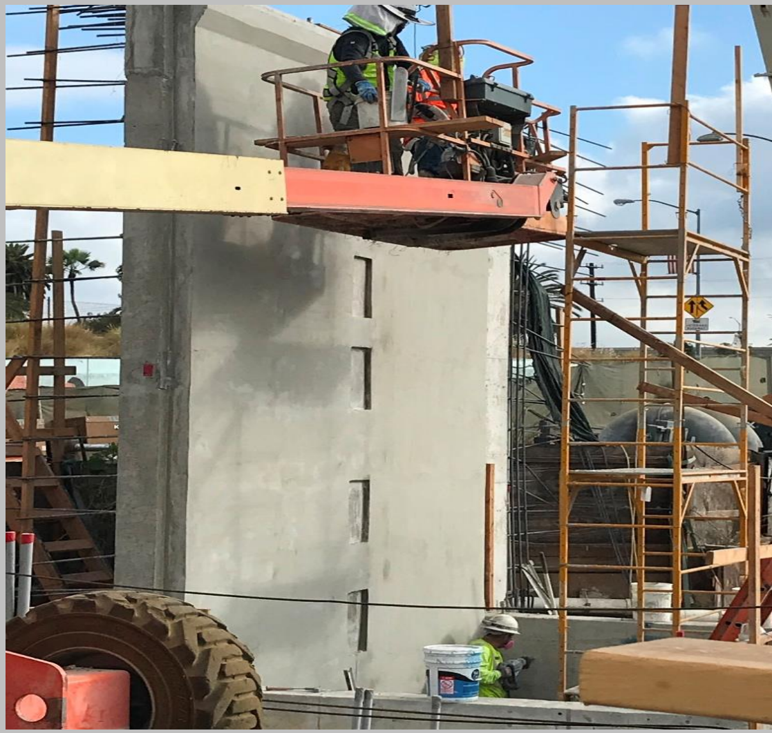
Finishing work for pedestrian bridge wall section. (September 2026)
