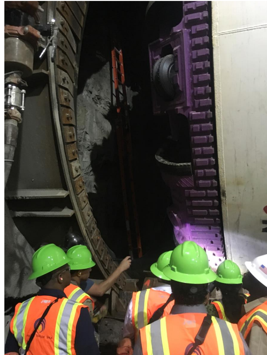
TBM – Prior to Boring
