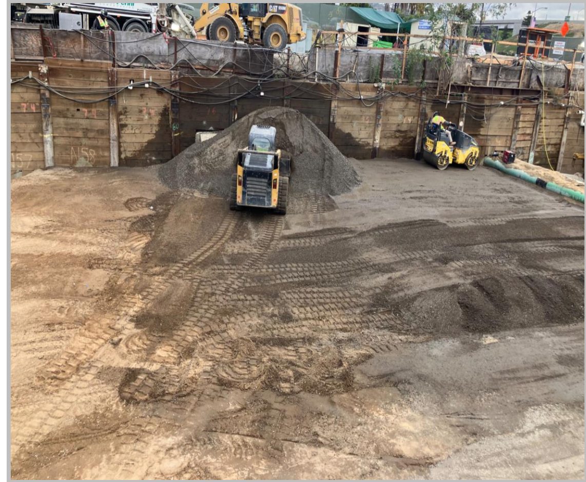
Main station box backfill
