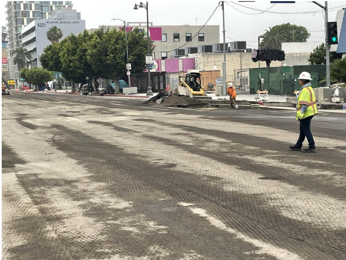
Wilshire/Fairfax Final Pave Work
