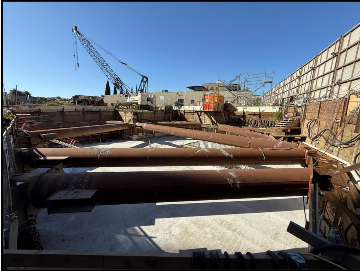
Post concrete pour for the main entrance roof, facing West. (February 2026)
