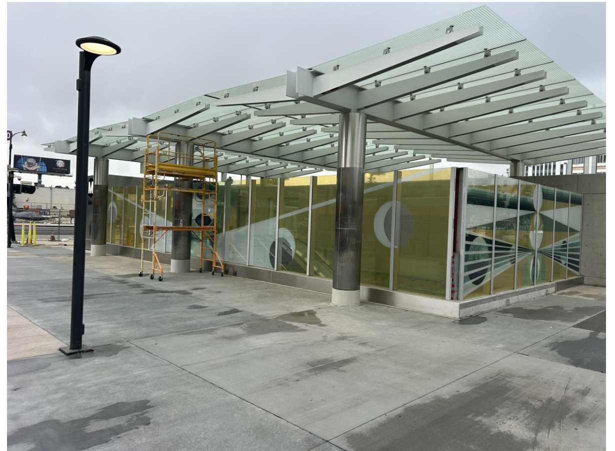
Wilshire/La Brea Entrance Portal Construction
