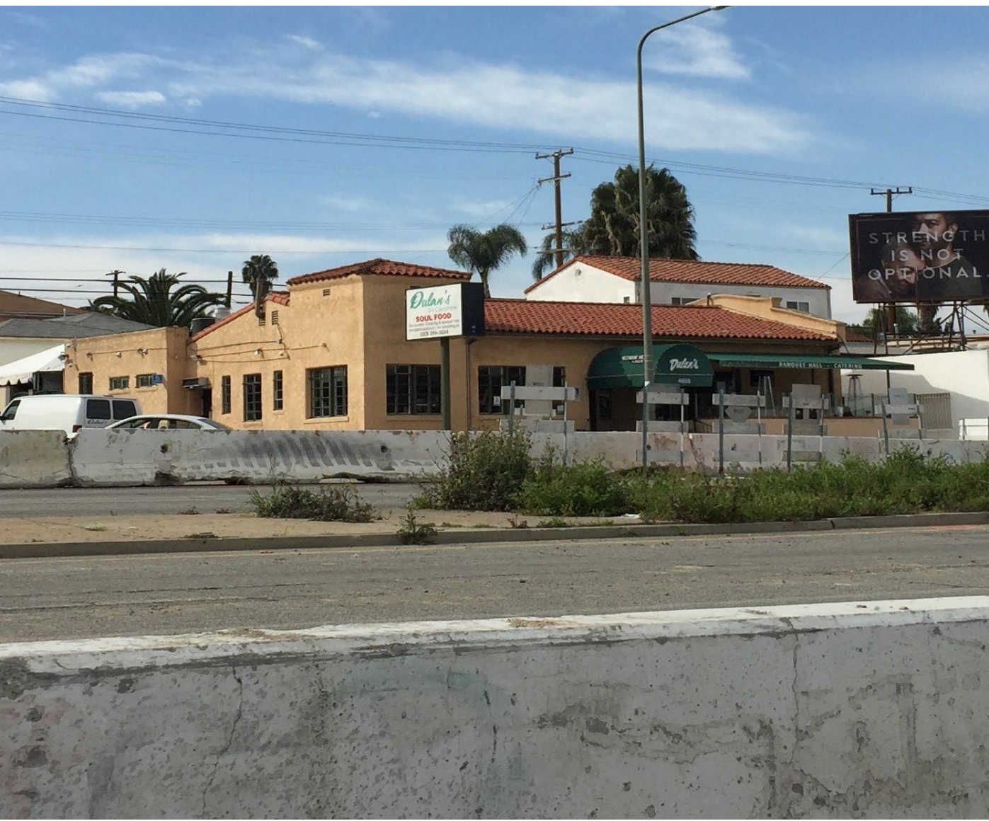
Construction located across the street from Dulan's Restaurant.
