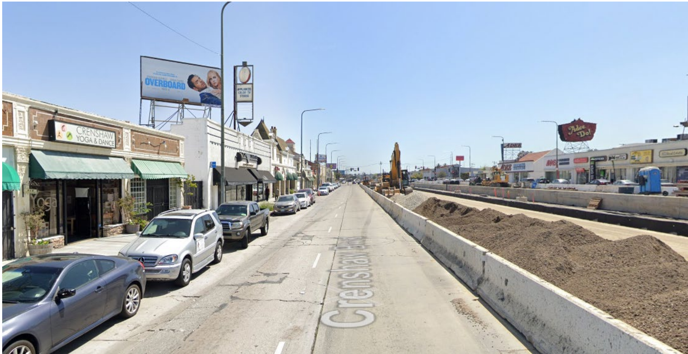
Construction located across the street from Crenshaw Yoga & Dance.
