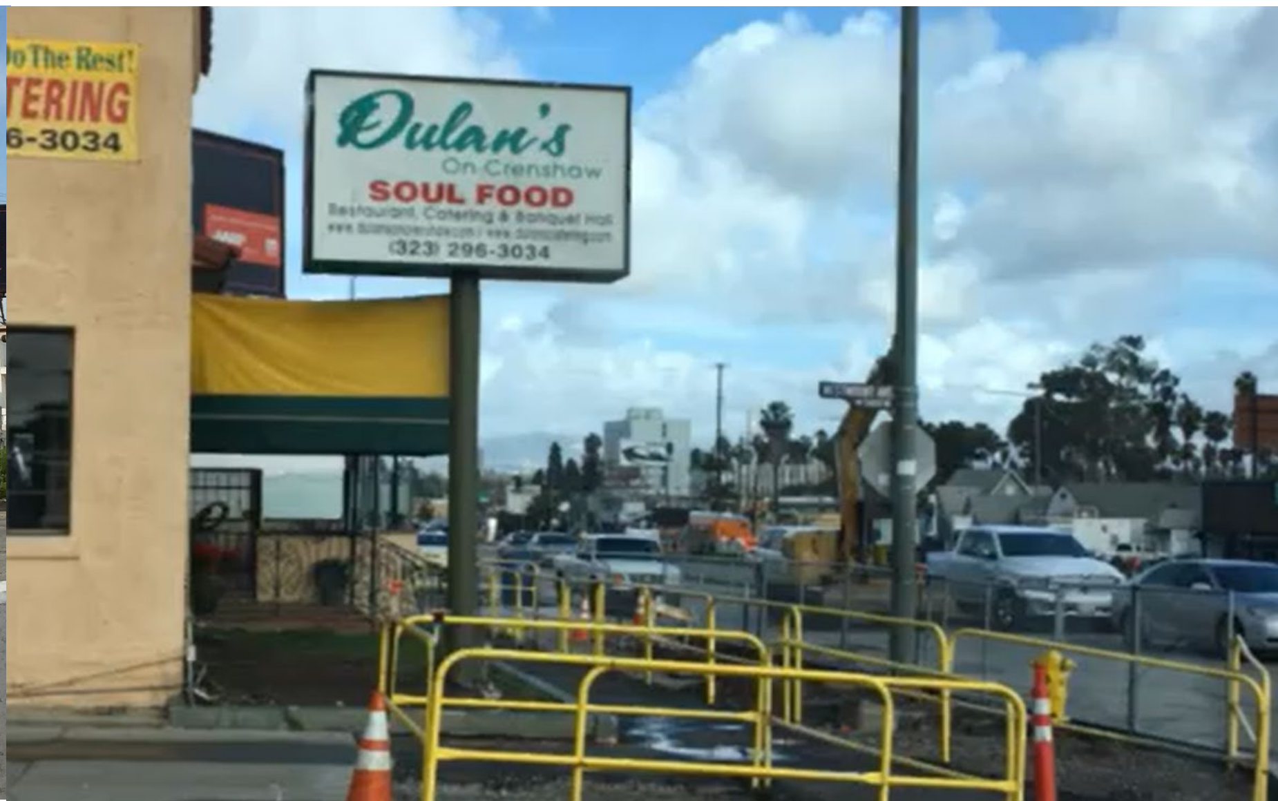
Construction located next to and across the street from Dulan's Restaurant.
