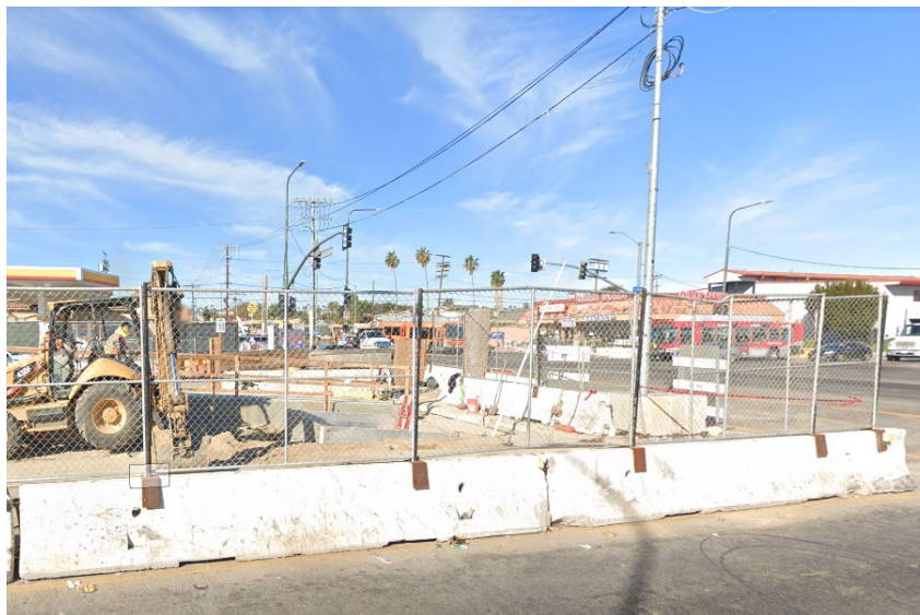
Construction activity at Crenshaw Boulevard/Slauson Avenue
