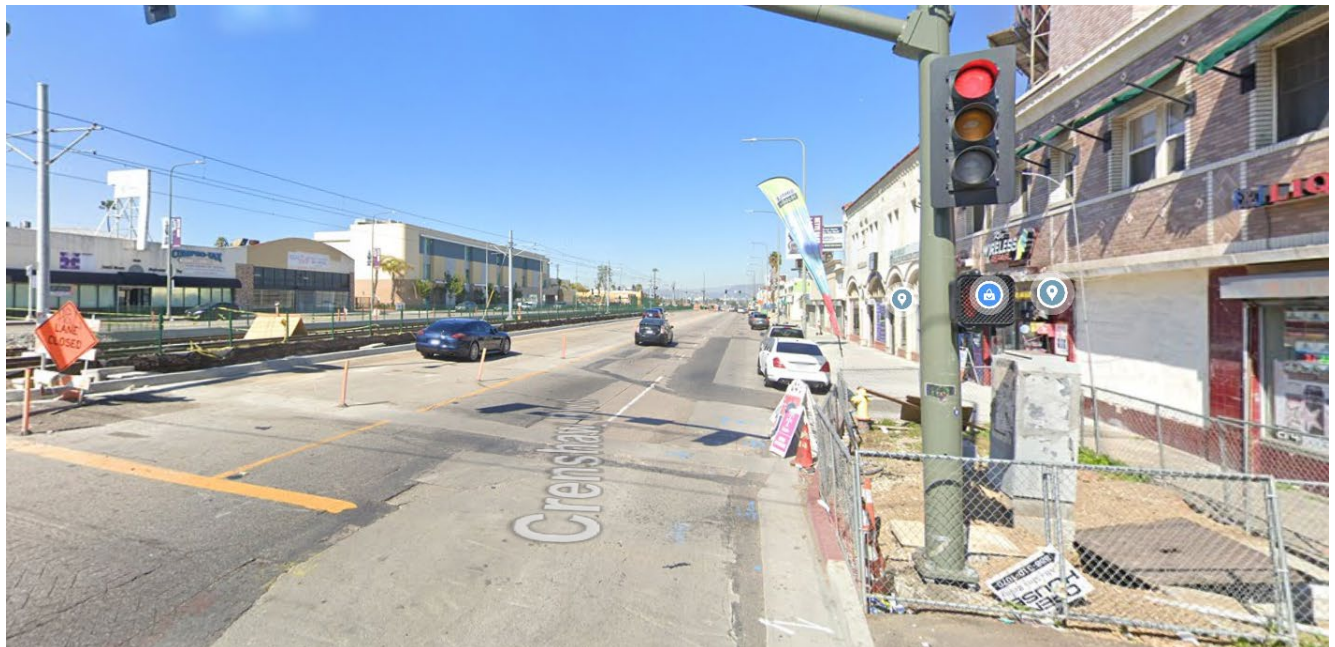
Crenshaw Blvd. and 54 th St. construction activity.
