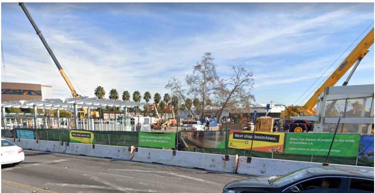
Station Construction at Crenshaw Blvd. and Exposition Blvd.
