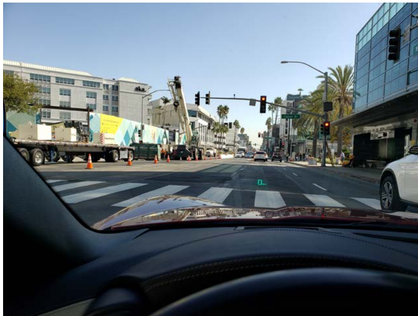
Construction at N. Canon Drive and Wilshire Blvd. in Beverly Hills (Purple Line Extension Section 2)
