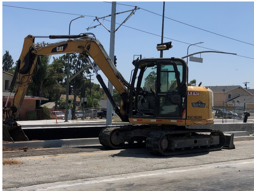
Construction on Crenshaw Blvd. at grade segment.
