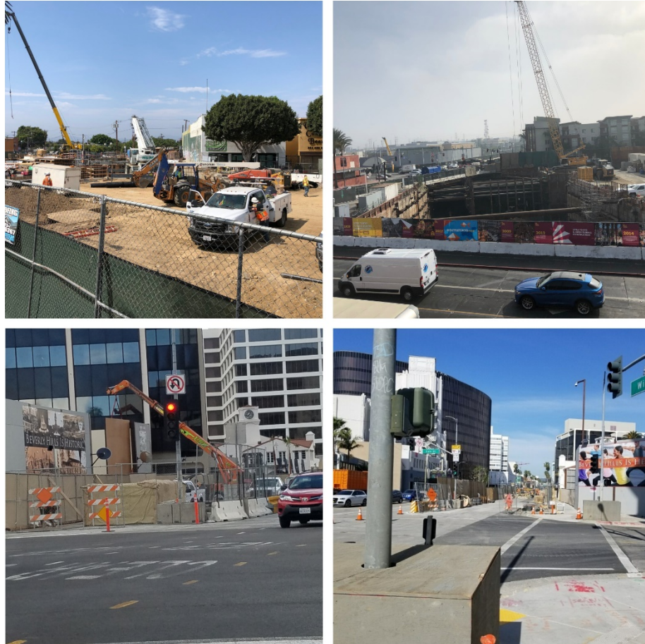
Construction activity in all four BIF areas: (clockwise from top left) Crenshaw/LAX, Little Tokyo Area of the Regional Connector, Purple Line Extension, Section 1, Purple Line Extension, Section 2
