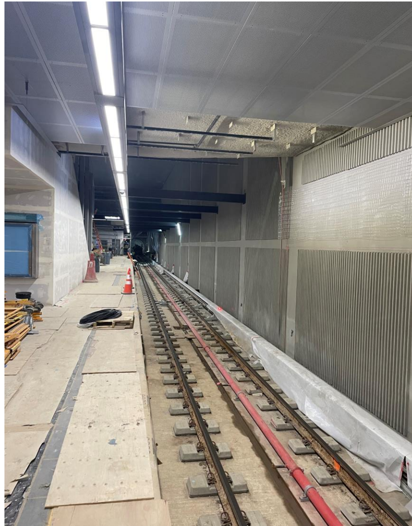
Trainway Looking West
