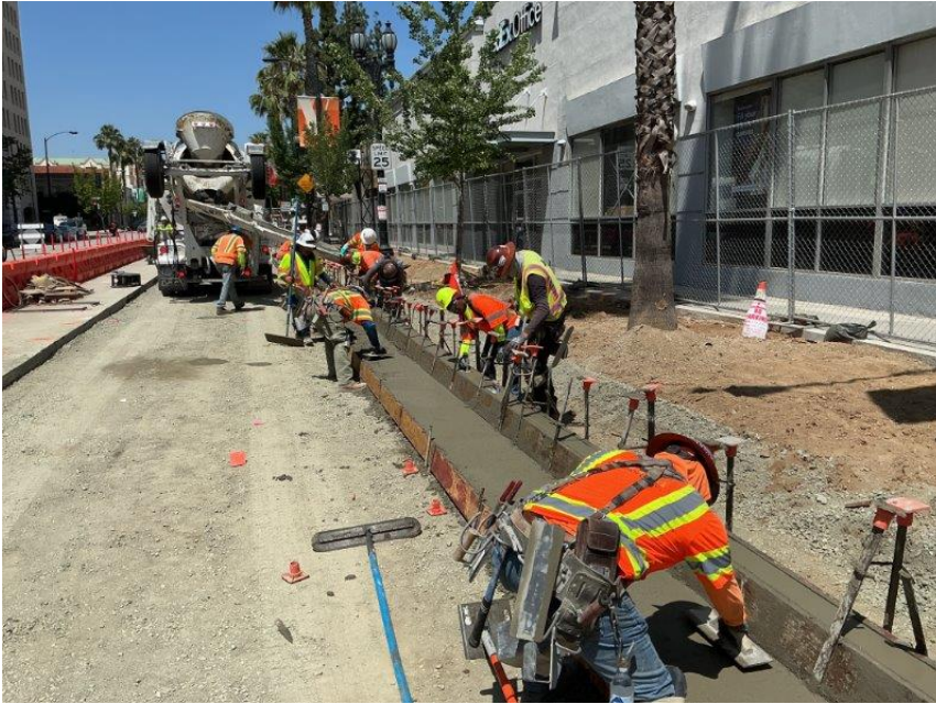
Concrete pours to form new curbs & gutters
