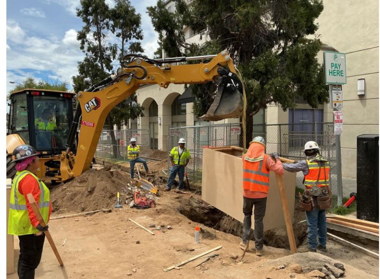
Installation of catch basins to support proper drainage
