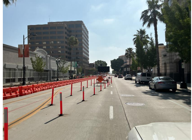
Cones and directional signs guide traffic through open lanes near work areas
