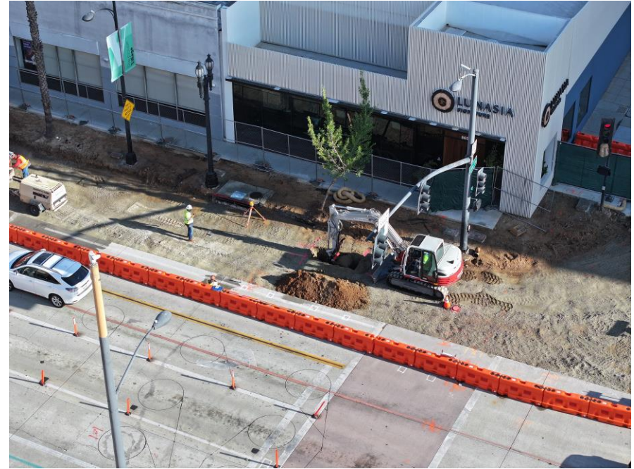
Construction at Colorado Bl/Lake Av intersection
