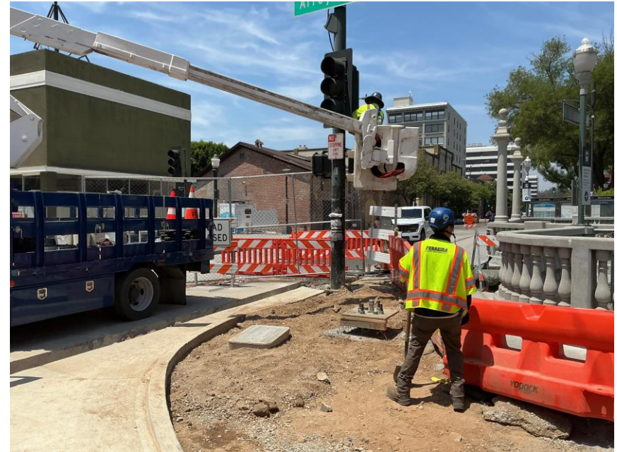
Traffic signal electrical work
