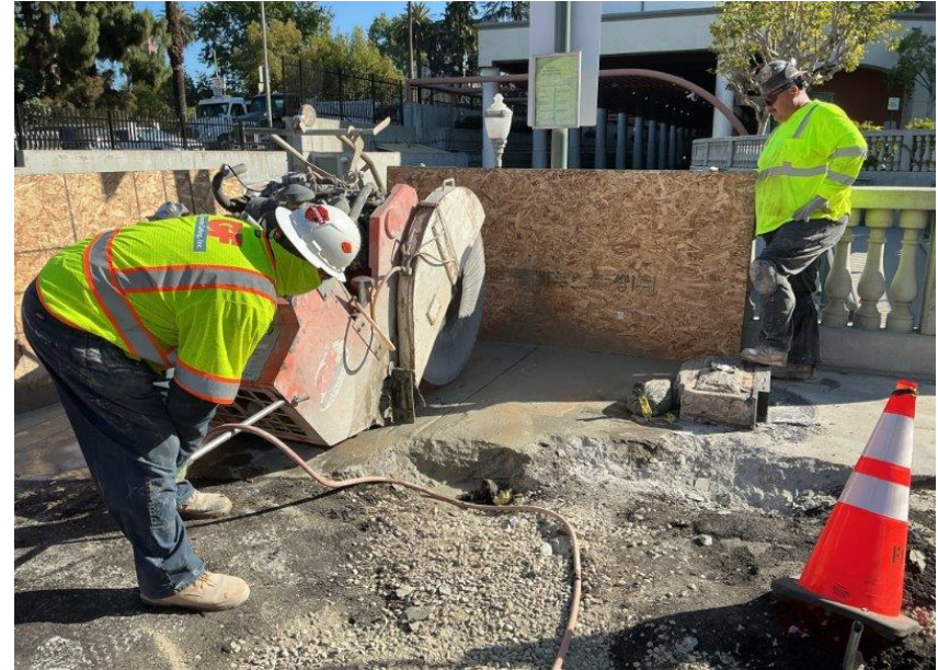
Saw cutting of sidewalks and roadways
