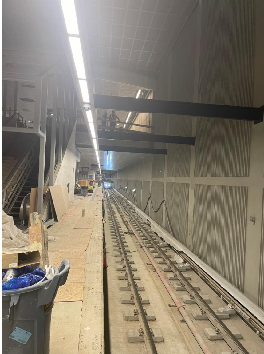
Station Track Level Looking West
