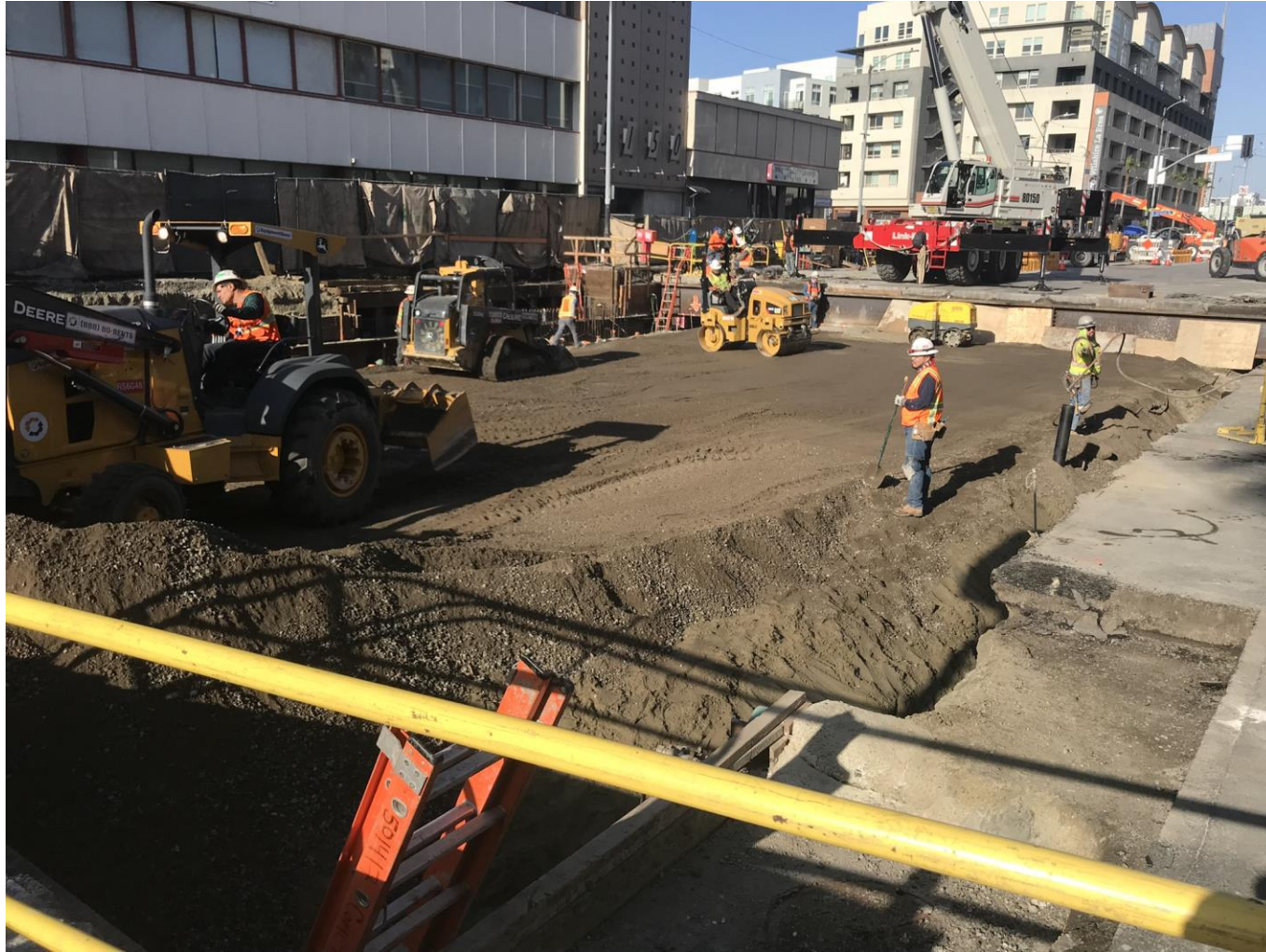
Wilshire/La Brea Decking Removal
