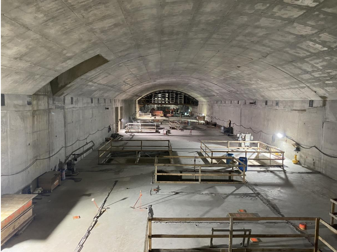
La Cienega Station Work - 2022
