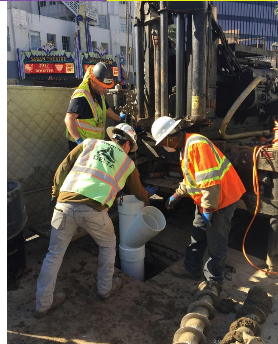
Example of instrumentation drilling
