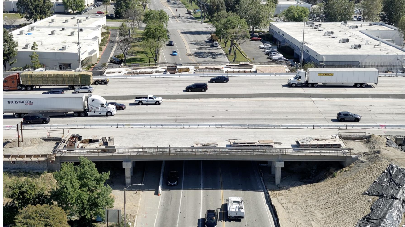
Rye Canyon Rd Bridge Segment – March 2026
