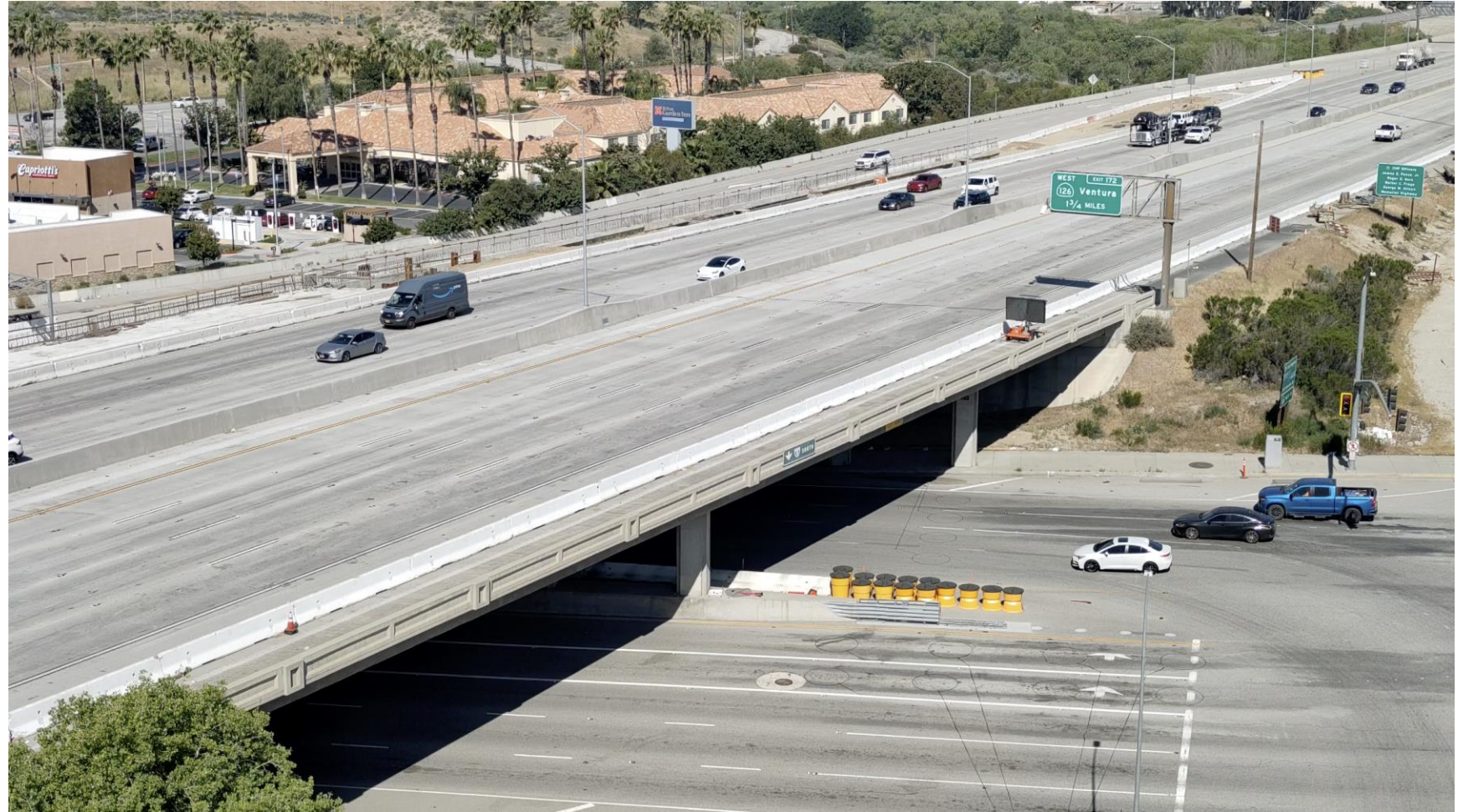
Magic Mountain Pkwy Bridge Segment – March 2026
