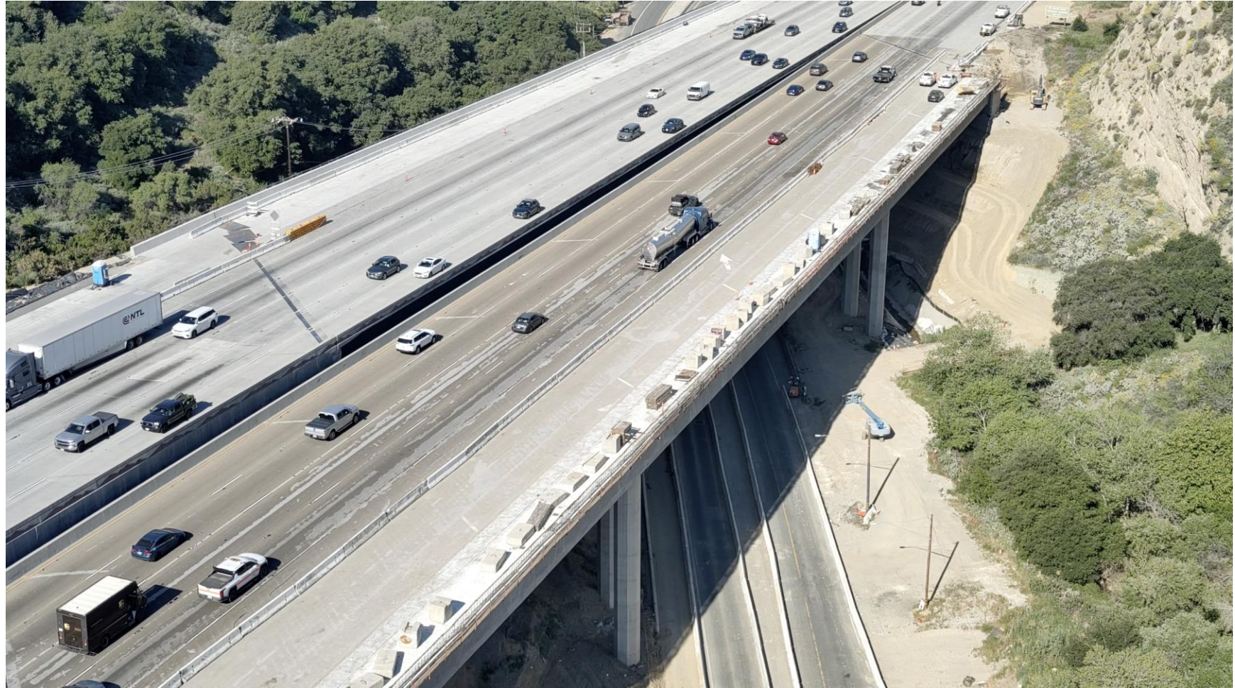
Gavin Canyon Bridge Segment – March 2026
