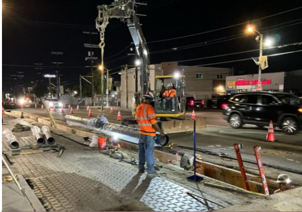
Utility work in Pacoima involving the installation of a water pipe
