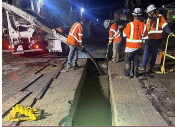
Work being performed to protect existing sewer lines in Panorama City
