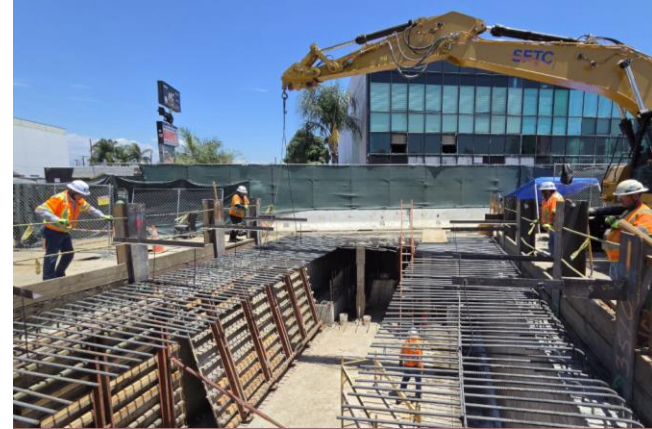
Work crews in Van Nuys conducting work for the Pacoima Wash box culvert reconstruction
