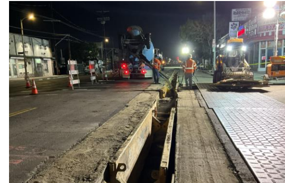
Crews backfill a trench before placing a steel plate so the roadway can reopen outside of work hours
