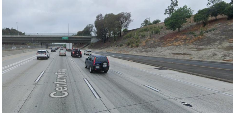
Typical I-105 retaining wall construction location
