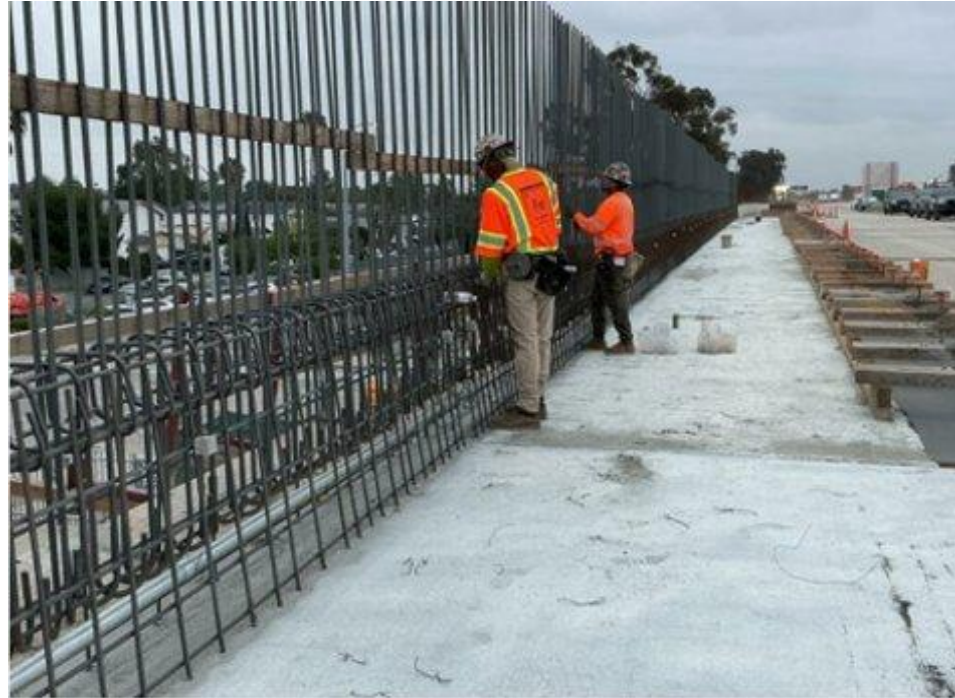
Avalon undercrossing wall rebar
