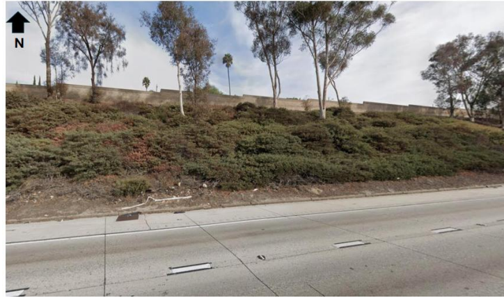
Typical I-105 retaining wall construction locations
