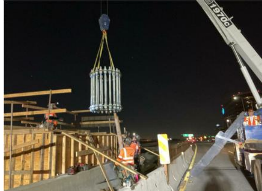
I-105 viaduct sign structure work near LAX
