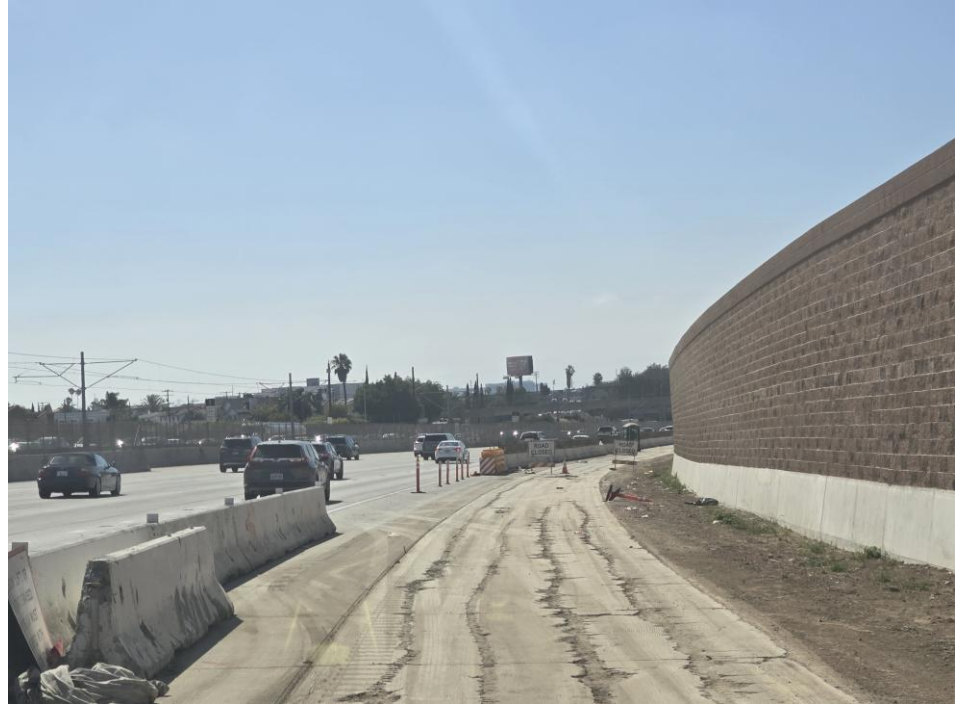
Newly reconstructed soundwall – south of Crenshaw BI
