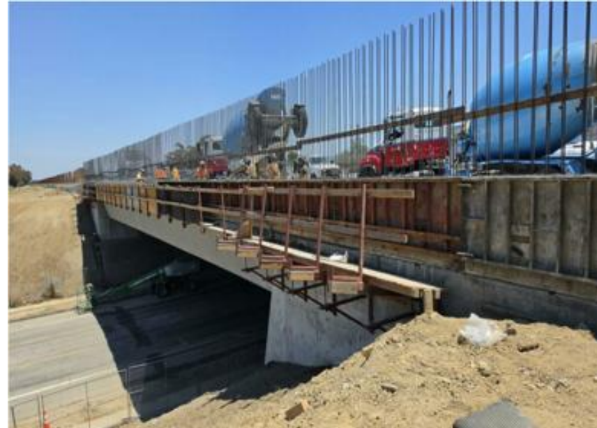
Westbound San Pedro undercrossing construction
