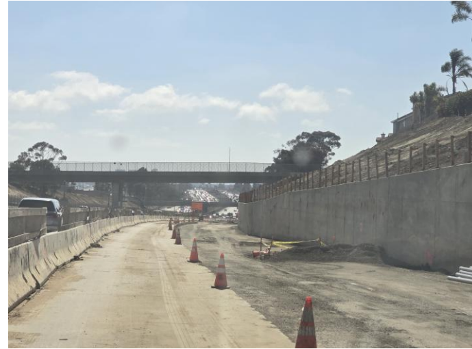
Retaining wall construction near Wilton Av
