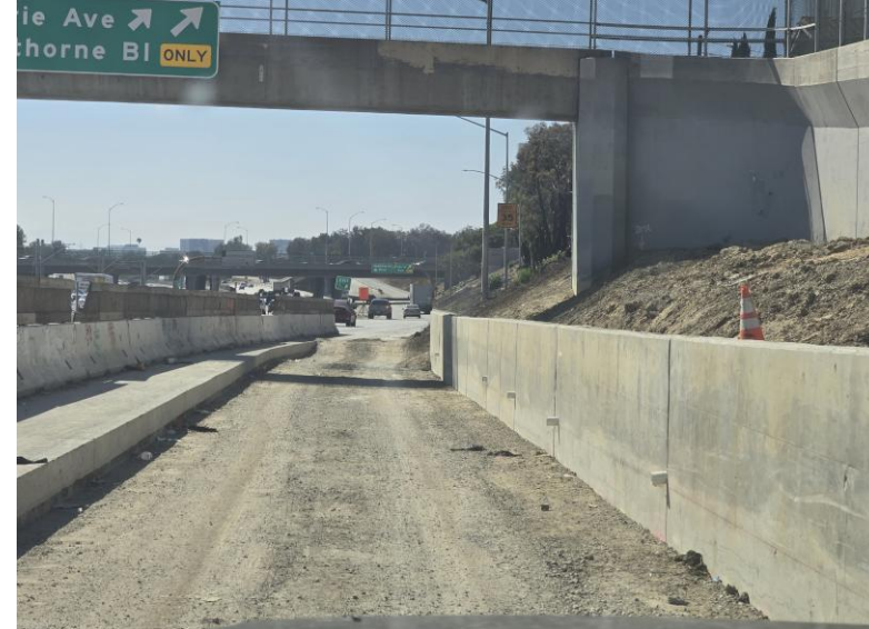
Retaining wall construction near WB Prairie off-ramp Av
