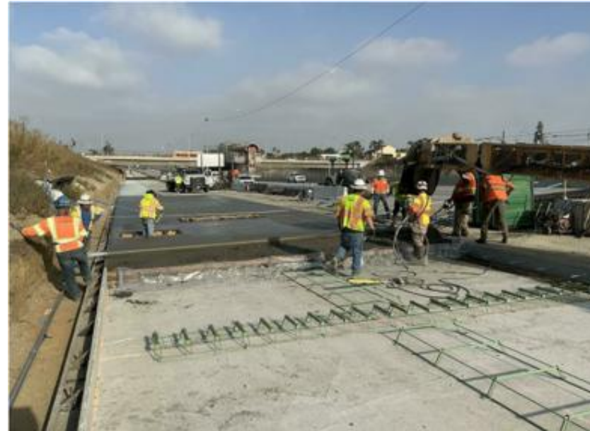
Roadway pavement construction near Vermont Av
