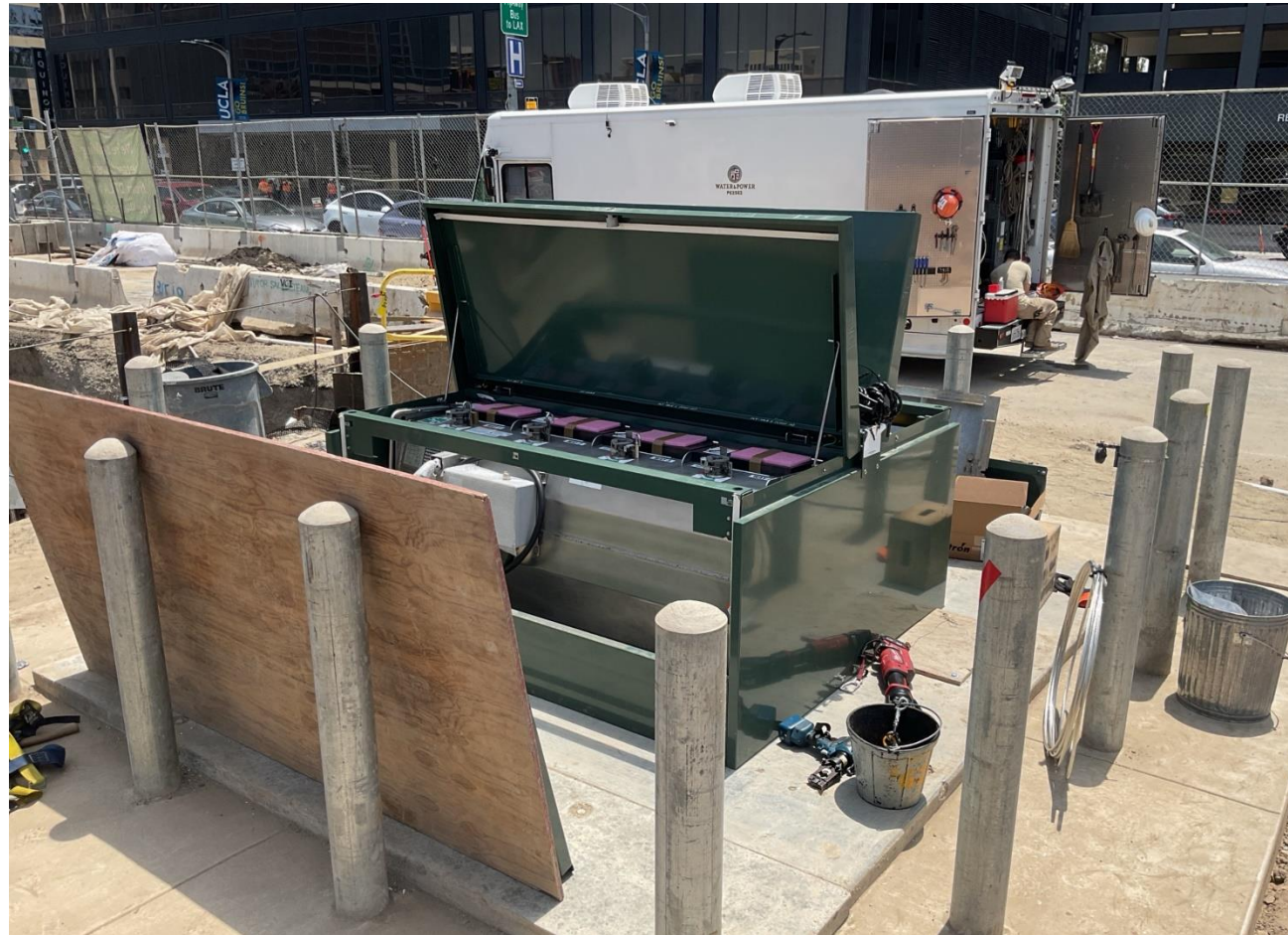
Vista Switchgear Installation on Surface Level
