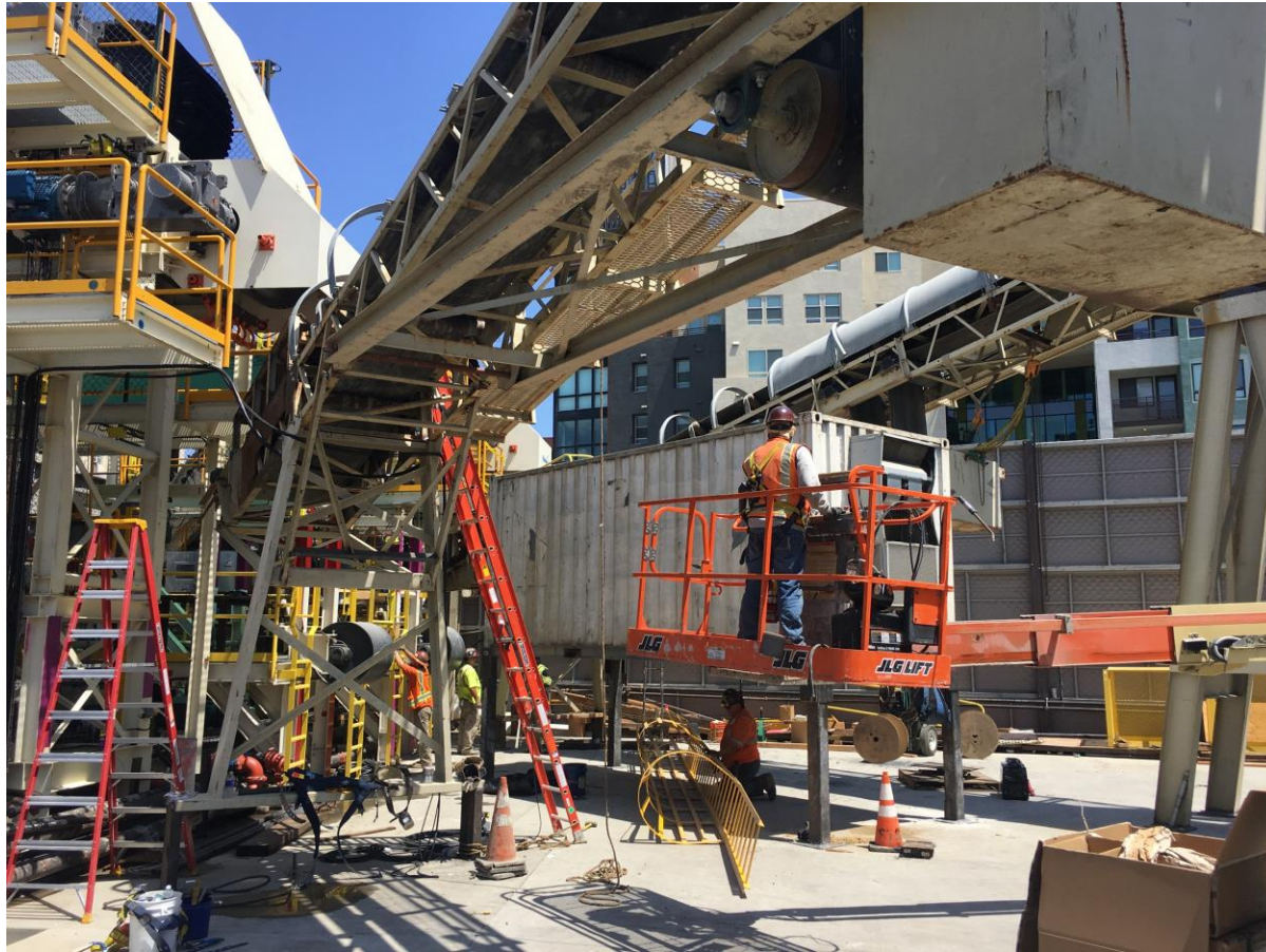
Muck Excavation from Tunnel – Wilshire/La Brea
