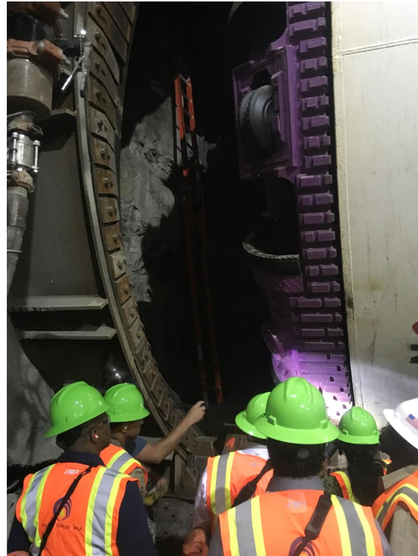
TBM – Prior to Boring
