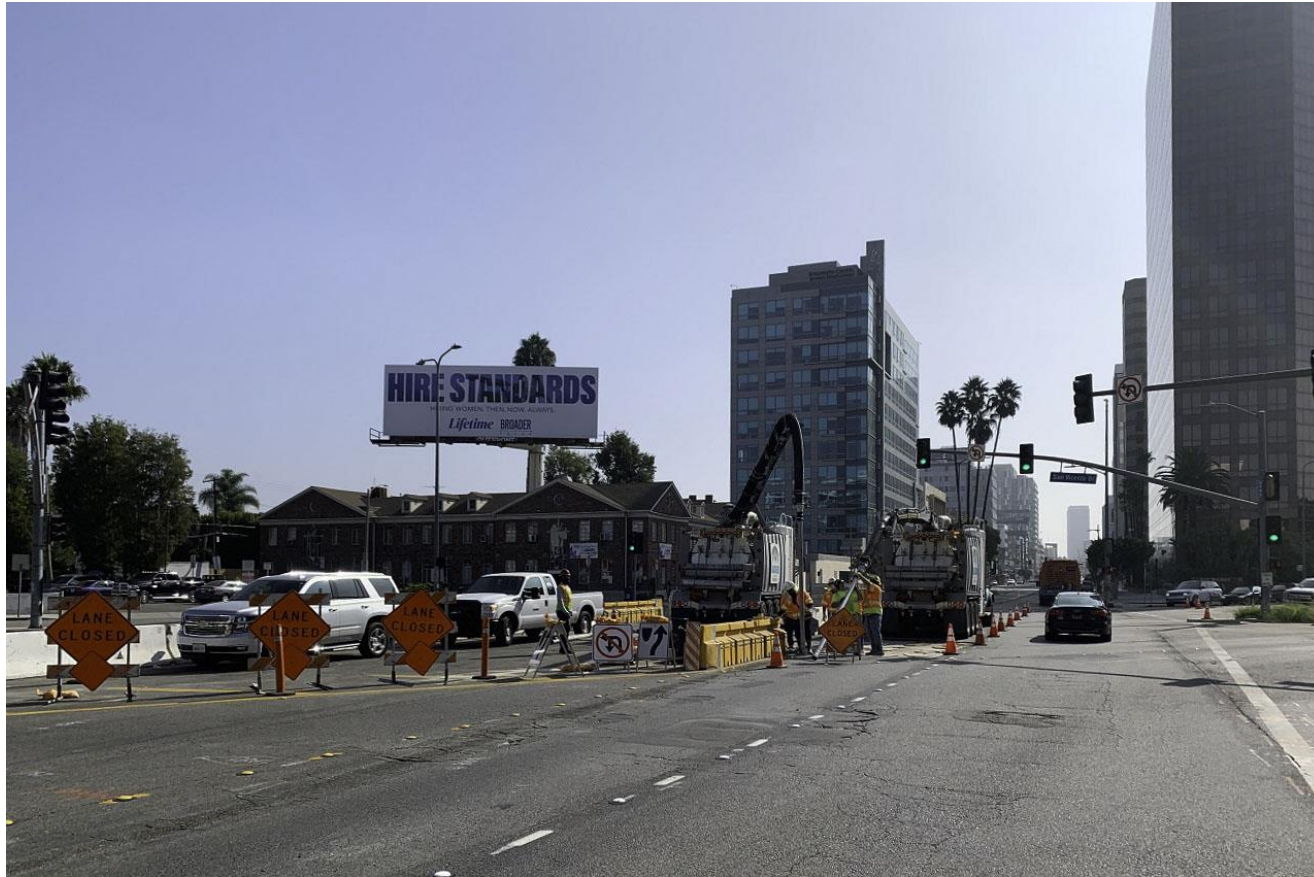
Wilshire/San Vicente Anomaly Work
