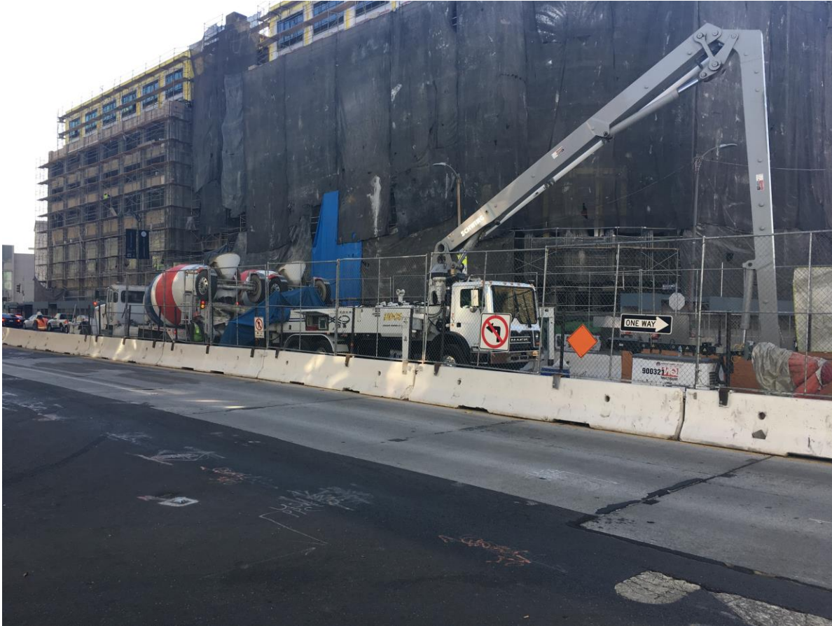
Center Muck Shaft – Wilshire/La Brea
