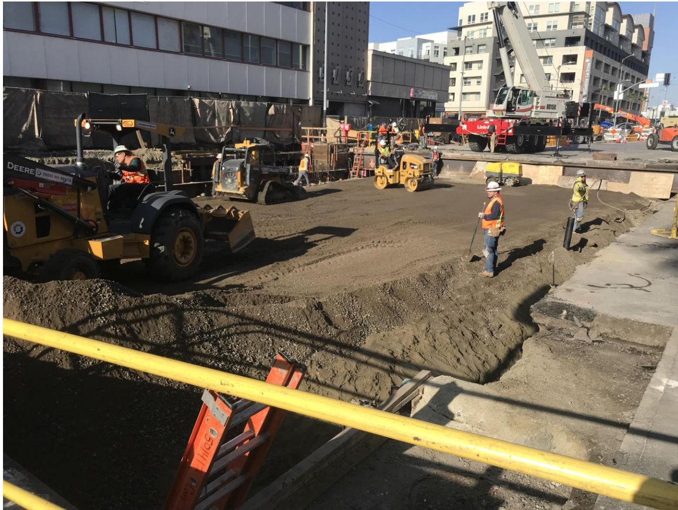
Wilshire/La Brea Decking Removal
