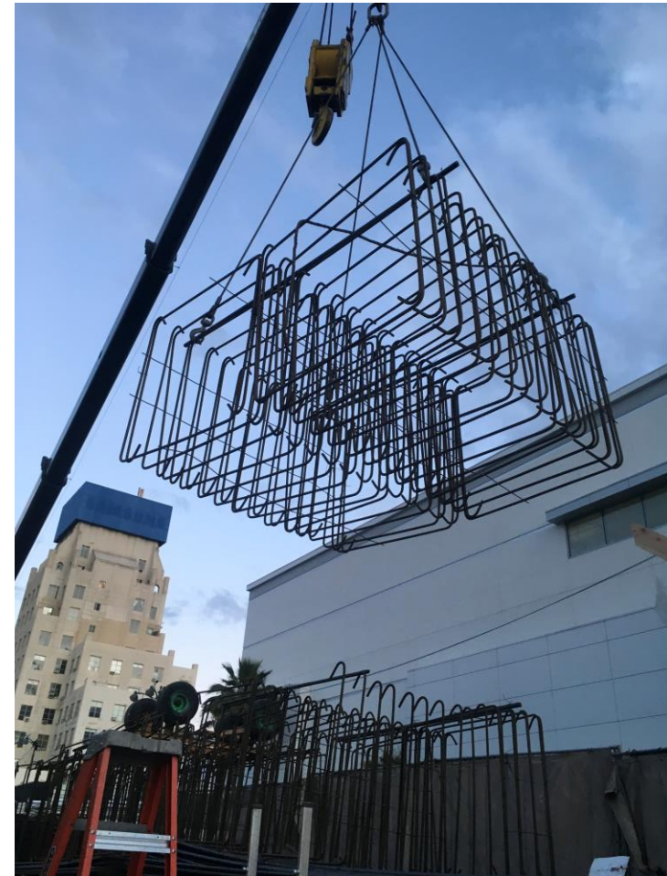
Structural Rebar – Wilshire/La Brea
