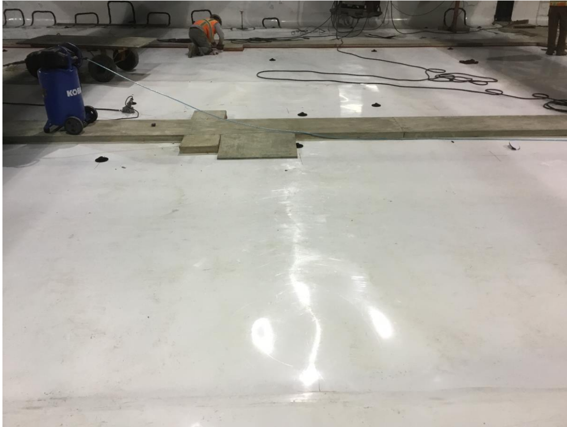
HDPE Placement – Wilshire/Fairfax
