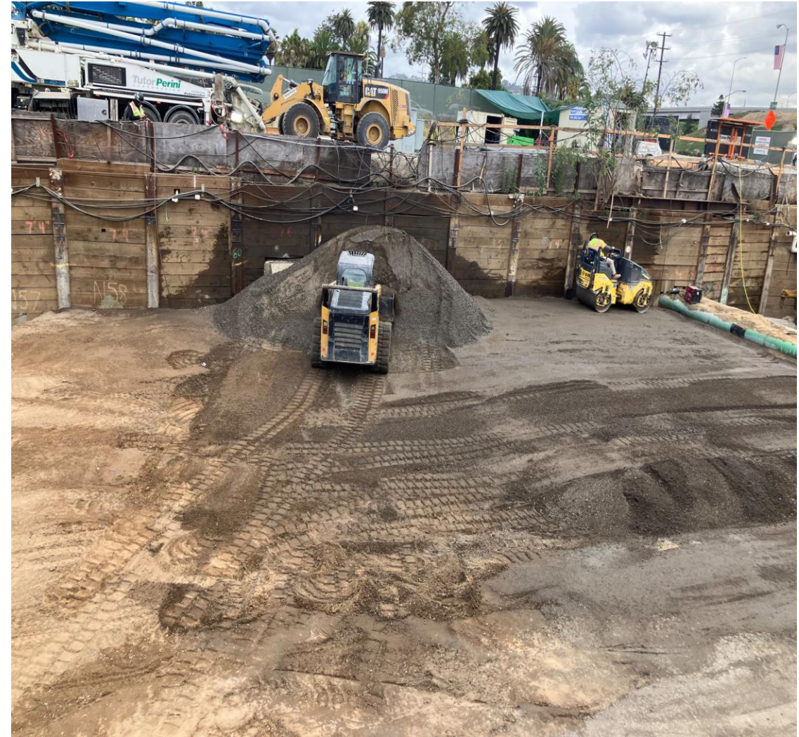
Main Station Backfill
