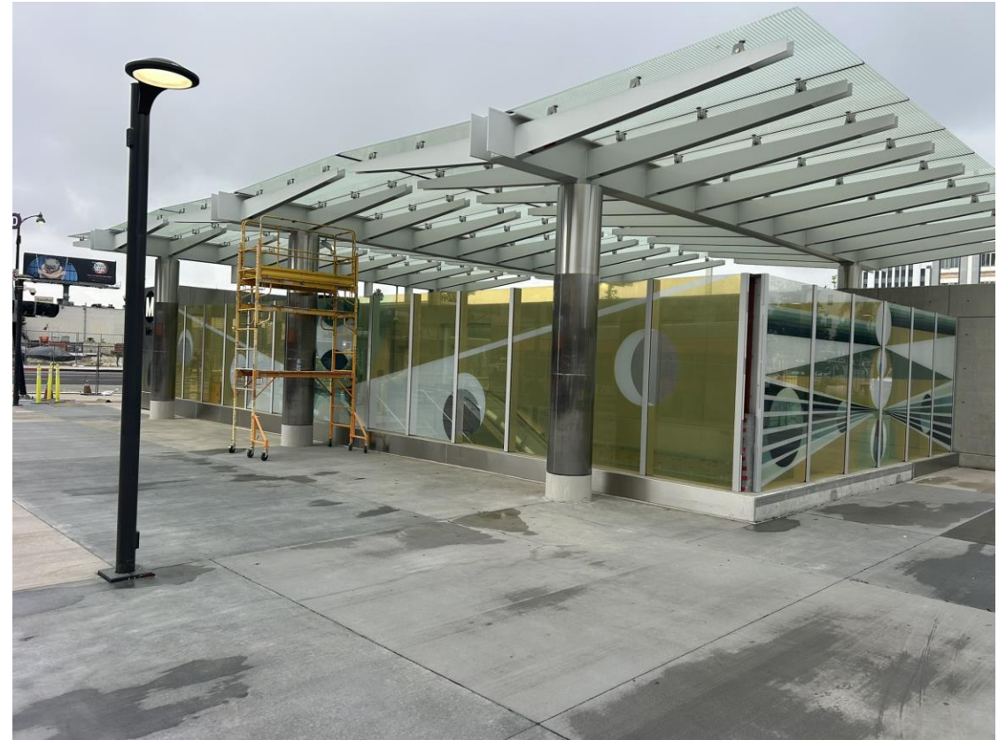
Wilshire/La Brea Entrance Portal Construction
