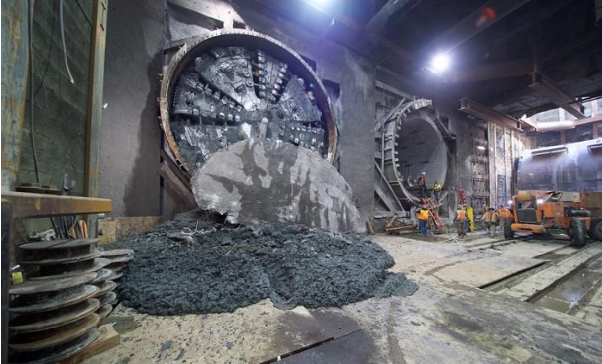
TBM Breakthrough
