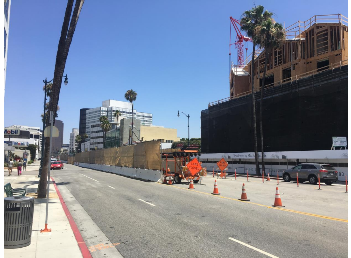
Cross Passage 26 – Wilshire/Stanley
