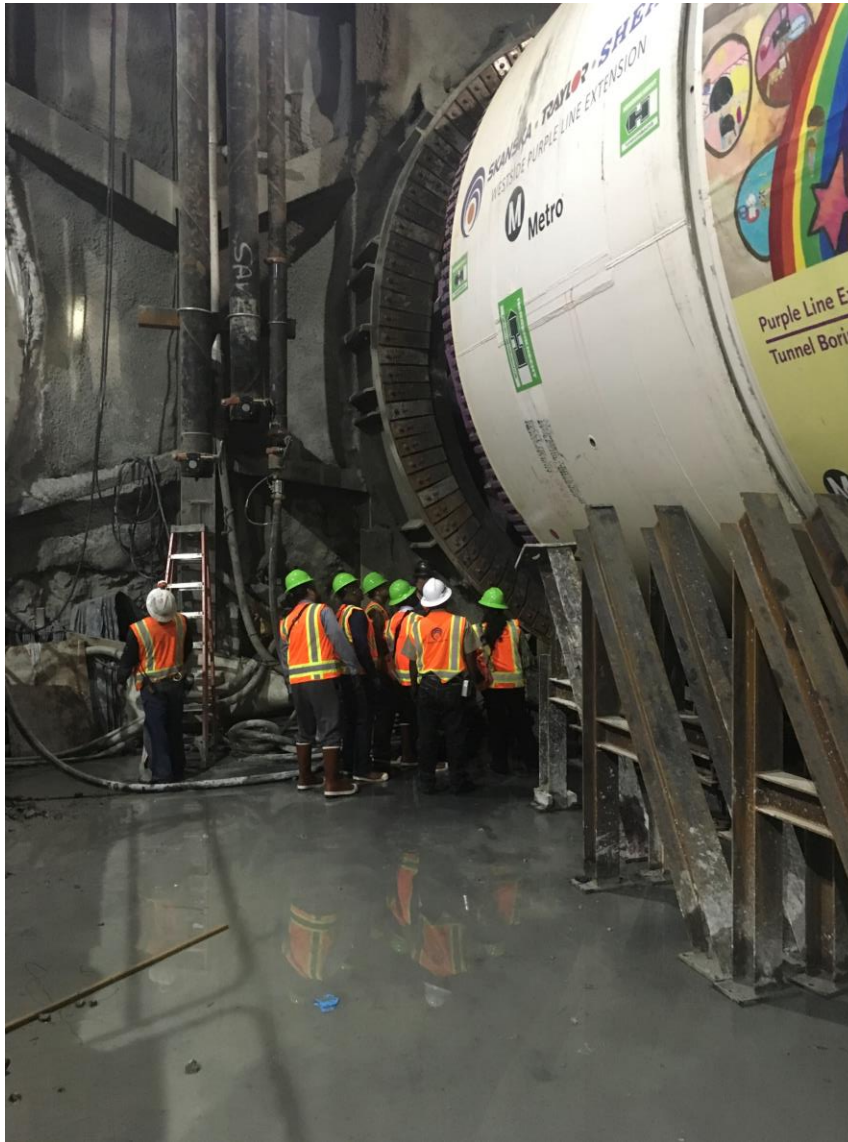
TBM – Facing West
