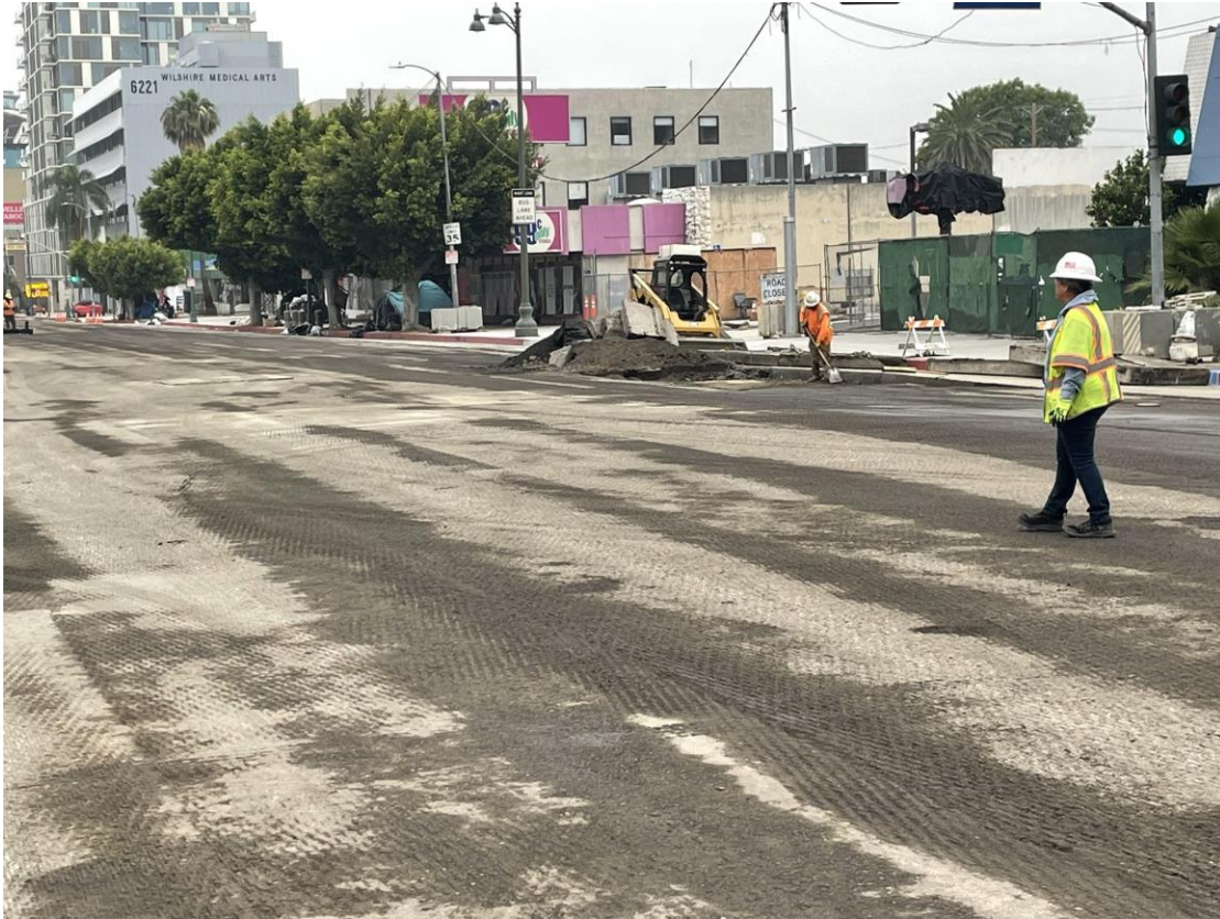
Wilshire/Fairfax Final Pave Work
