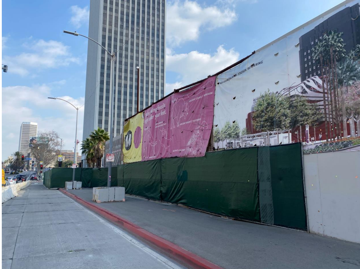
Wilshire/Fairfax Appendage Work
