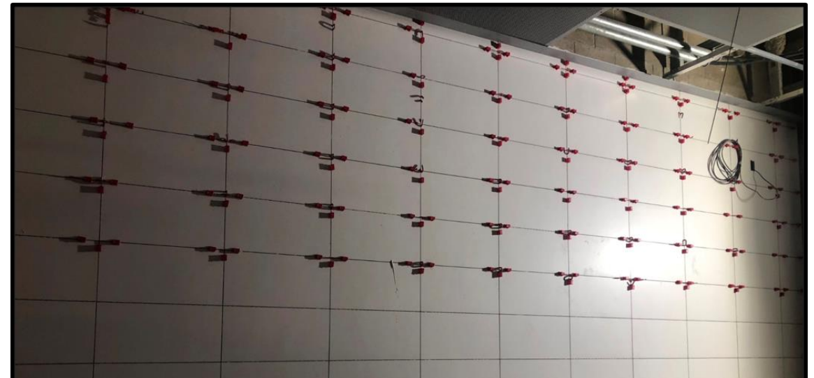
Porcelain tile installed in the Westwood/UCLA Station
