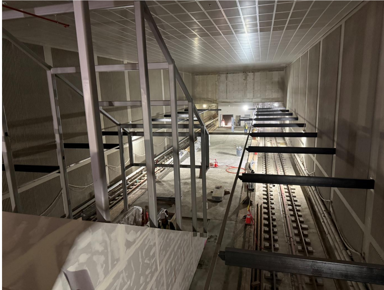
Station Concourse Looking East towards Track Platform Level
