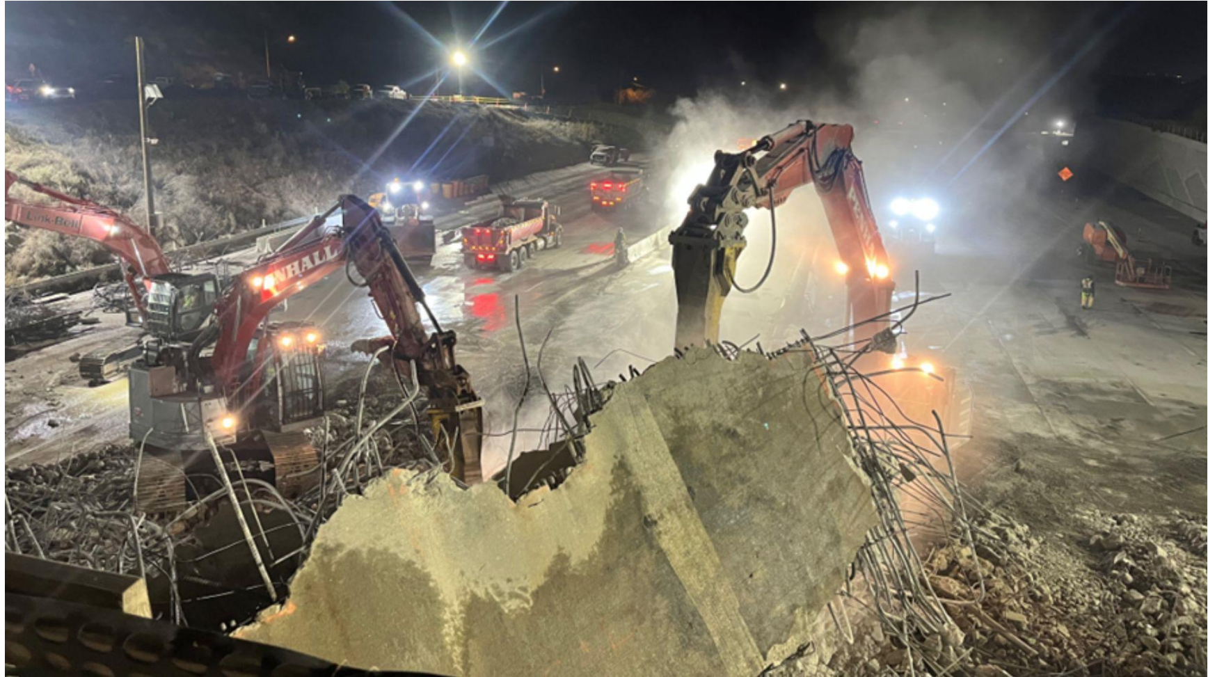
Weldon Canyon Rd Bridge Demolition, November 2023
