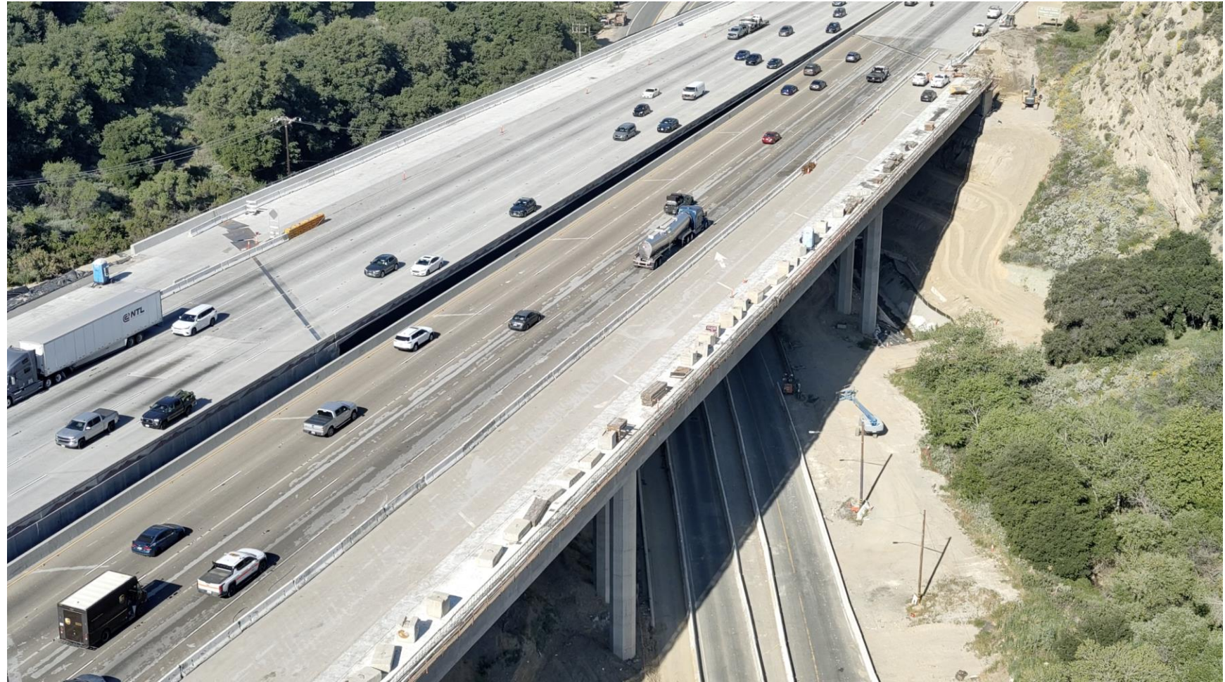
Gavin Canyon Bridge Segment – March 2026
