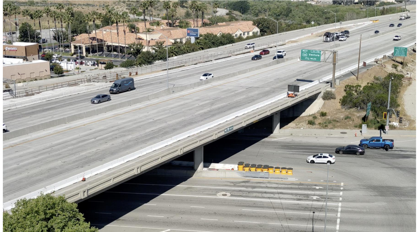
Magic Mountain Pkwy Bridge Segment – March 2026
