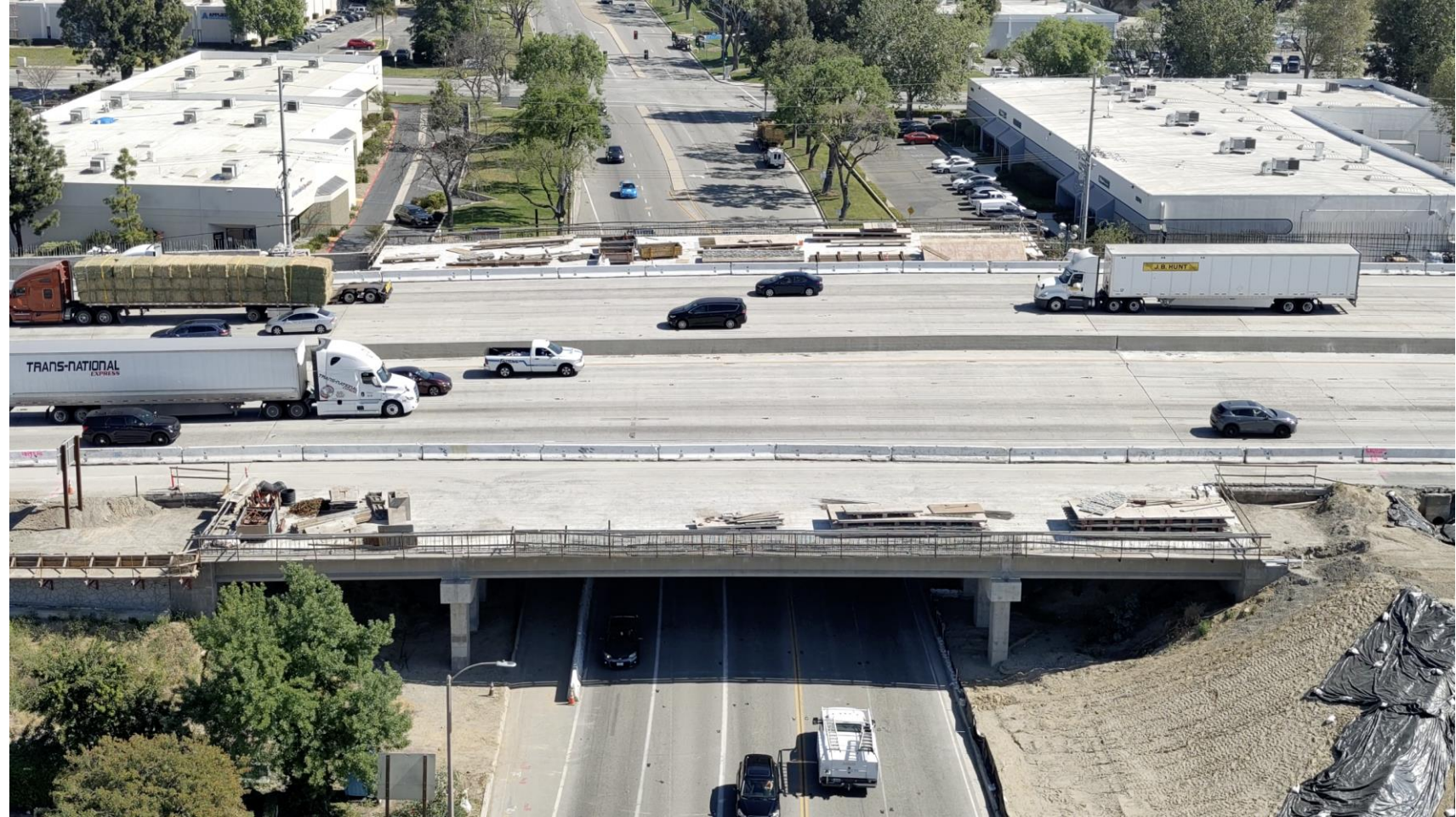
Rye Canyon Rd Bridge Segment – March 2026
