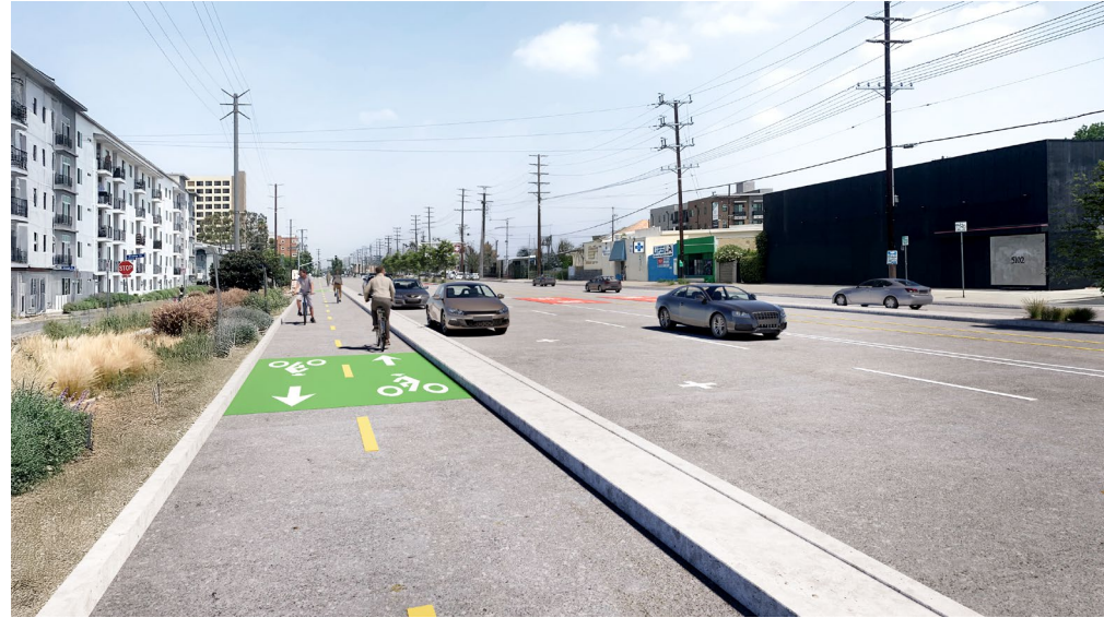
2-way cycle track on Vineland Av (looking north at Otsego St towards Magnolia Bl)
