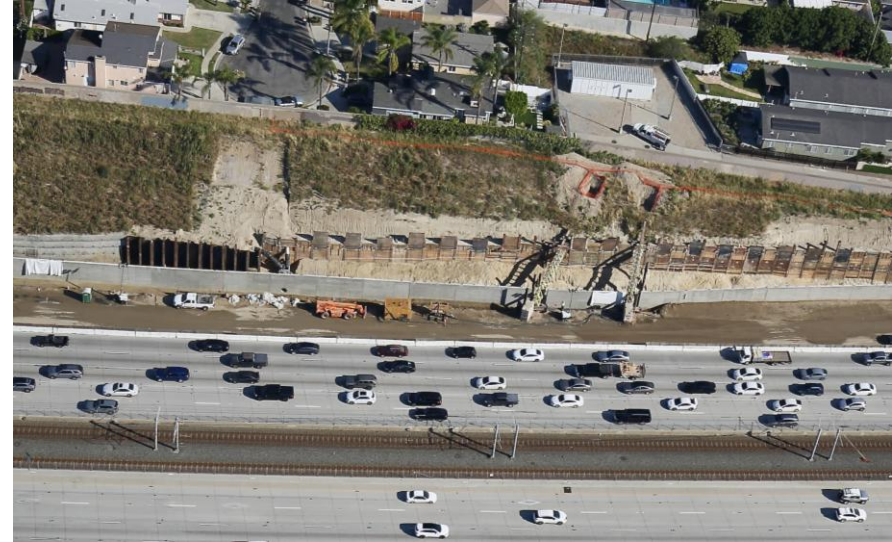
Retaining wall construction near Western Av
