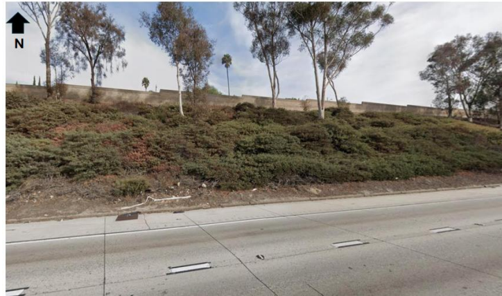
Typical I-105 retaining wall construction area
