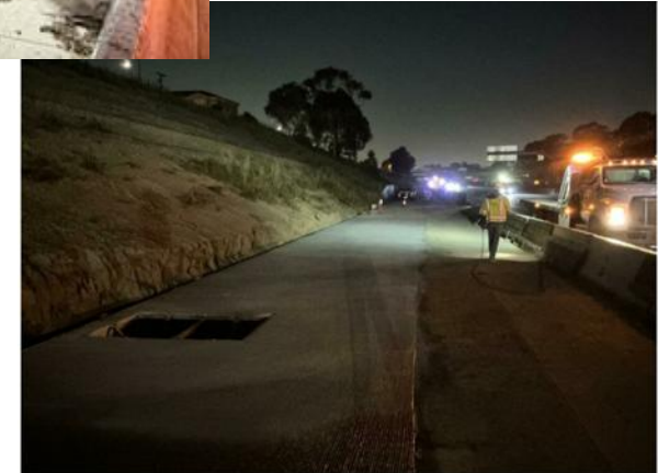
Roadway pavement construction
