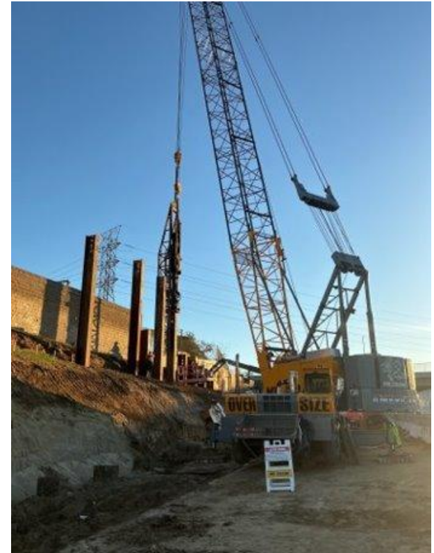
Shoring work activities for retaining wall construction
