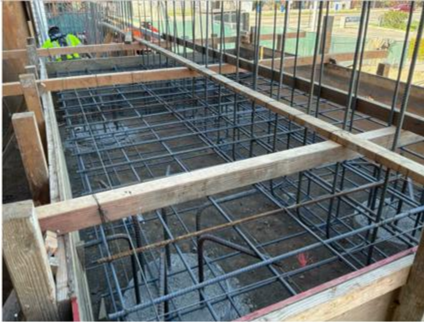
Westbound Avalon BI undercrossing abutment footing
