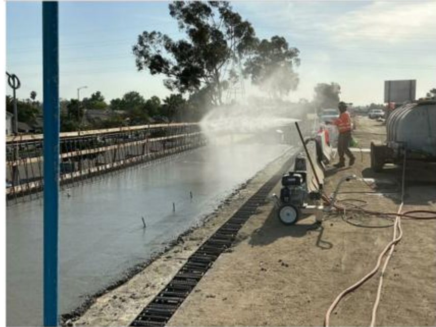
Westbound Avalon BI undercrossing concrete work
