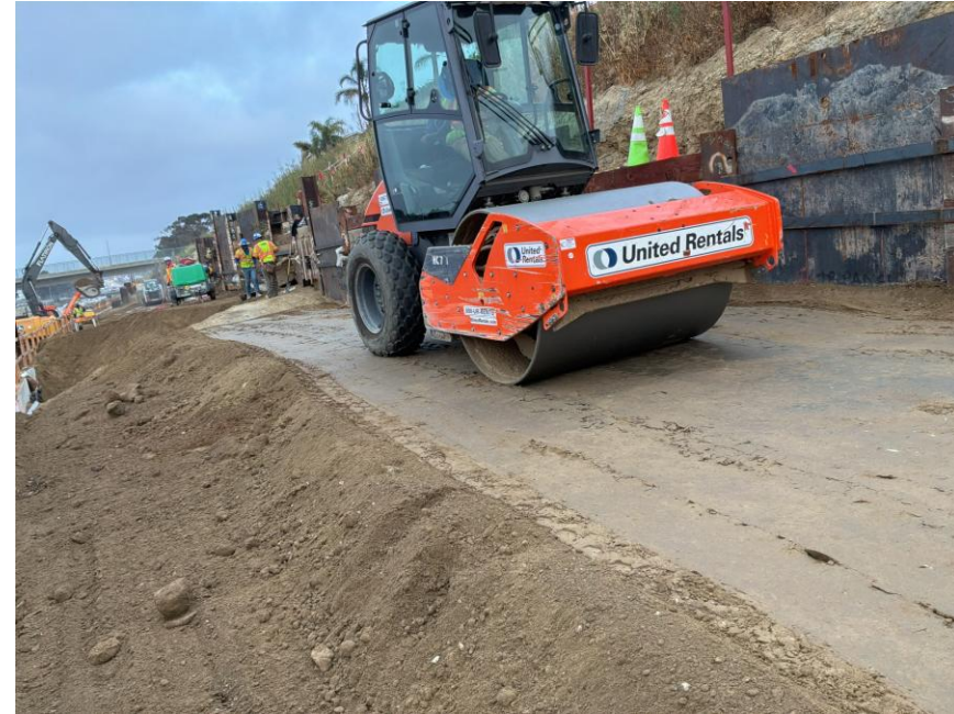
Soil compaction for retaining wall construction
