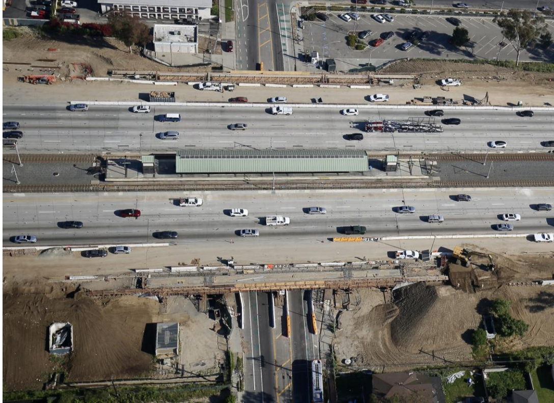
Avalon BI undercrossing construction
