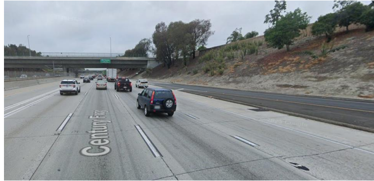
Typical I-105 retaining wall construction area
