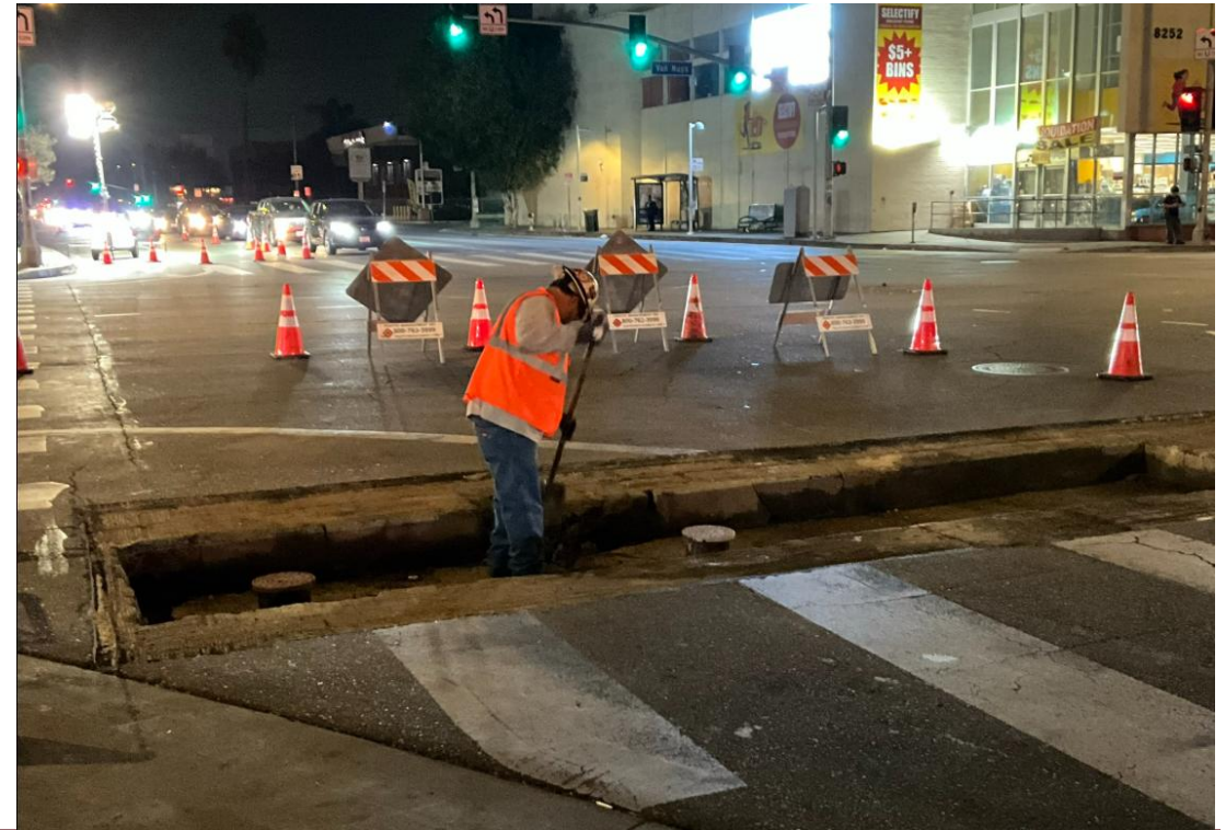
Trenching and excavation on Van Nuys Bl near Roscoe Bl for SoCalGas Work.
