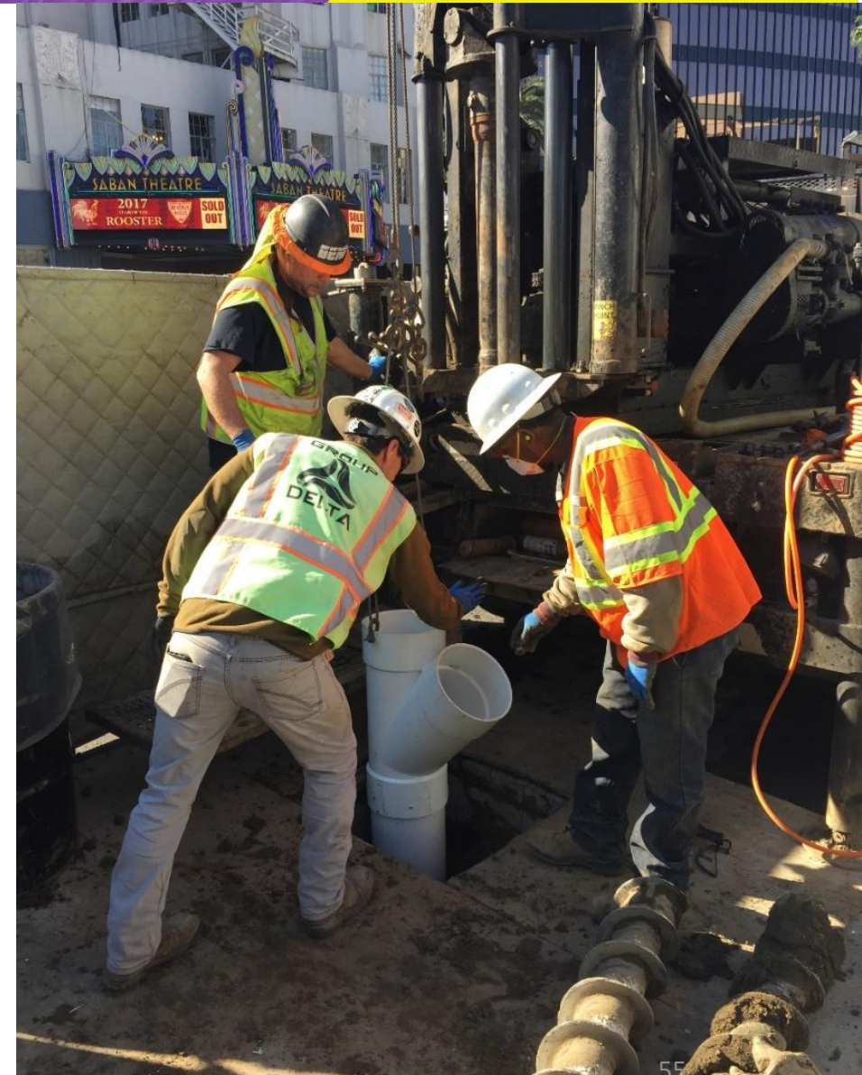
Example of instrumentation drilling
