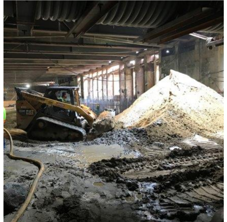
Main Station Box Backfill
