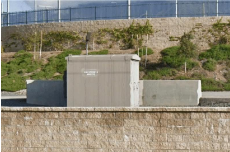
Figure 2.4-5. Typical Train Communications and Signaling Building
