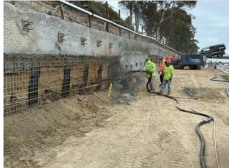
I-105 retaining wall construction
