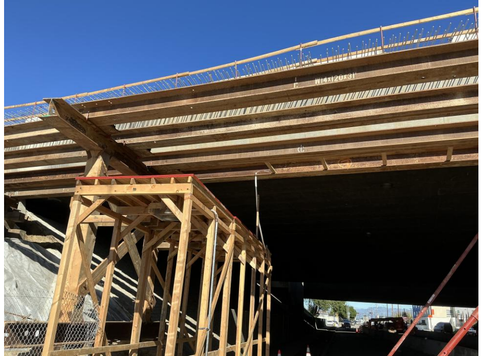
Main St falsework (bridge supports structures) installation
