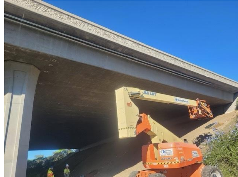
Electrical conduit installation at I-105 near Sundale Av
