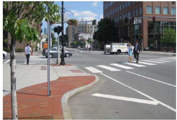
Curb extension and crosswalk
