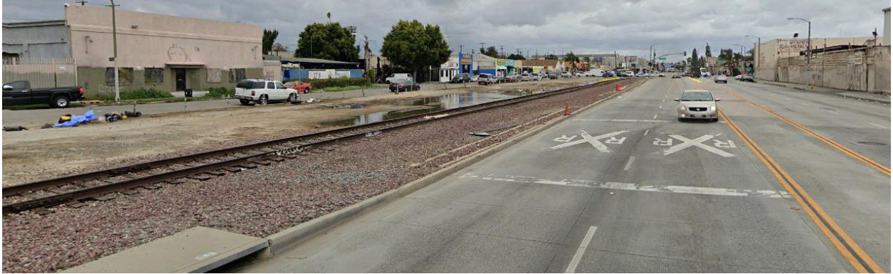
Metro-owned rail line along Slauson
