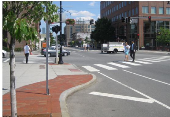
Curb extension and crosswalk
