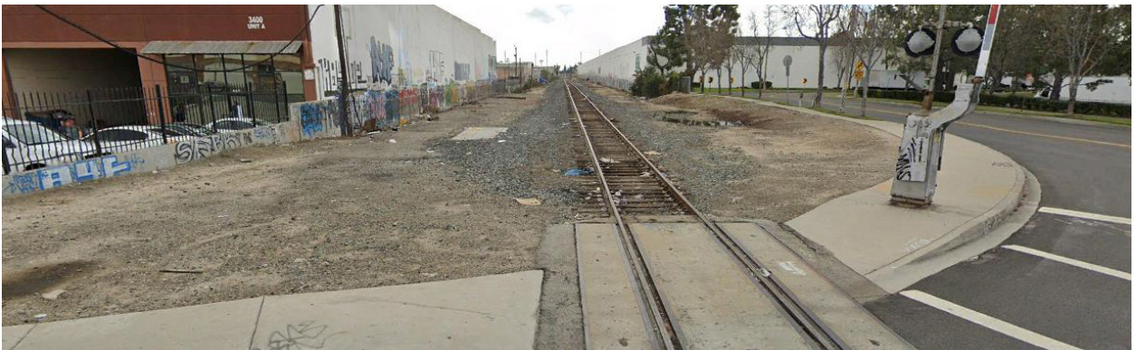
Rail line at Slauson and Downey looking south
