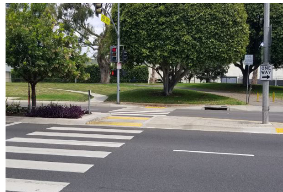
Median refuge island
