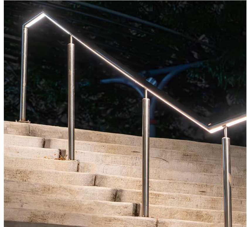
Installation of handrails with LED lighting (Grand Av Arts)
