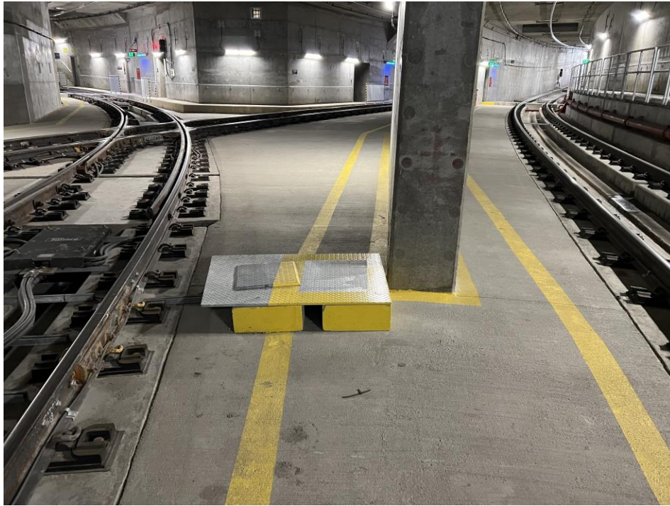
Installation of emergency walkway ramps at hazards
