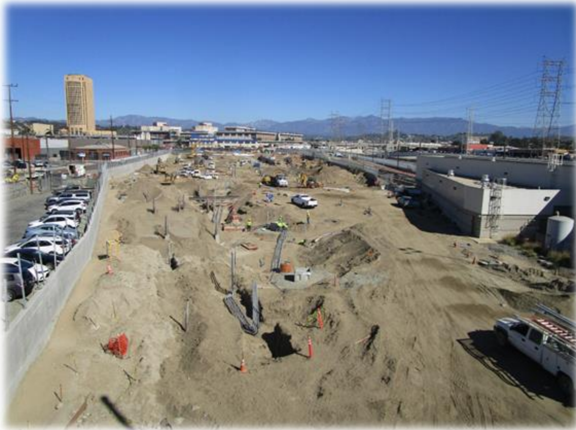
North Storage Yard- manholes & duct banks installation.
