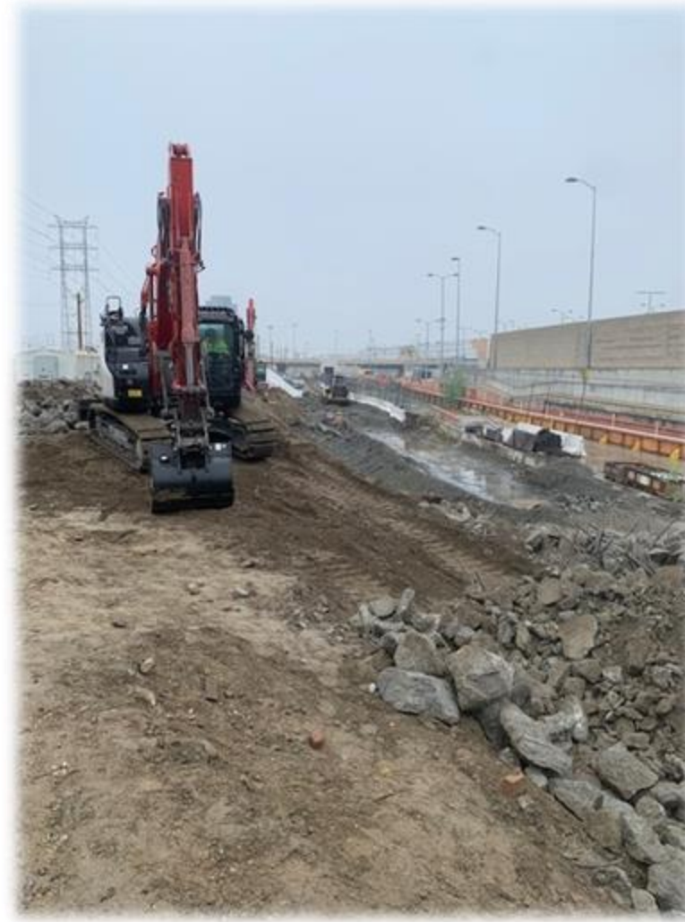
Demolition of Eastside portal retaining wall – looking in Southwest direction.
