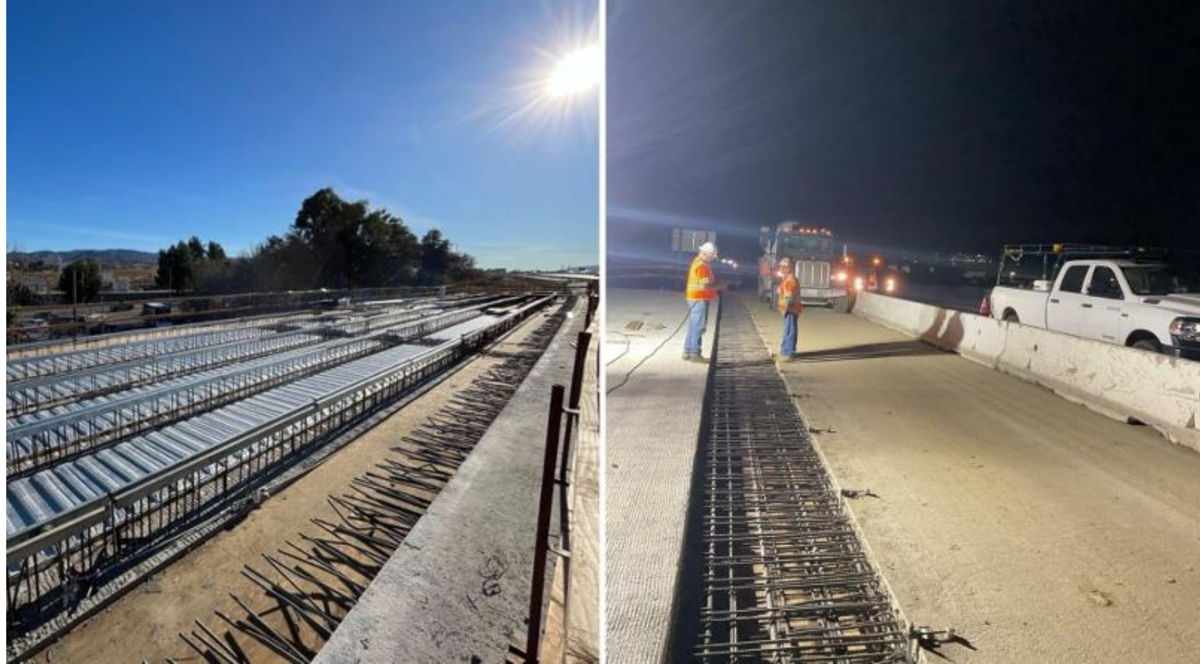
Rye Canyon Rd Bridge metal decking (left) – January 2025, concrete placement (right) – July 2025
