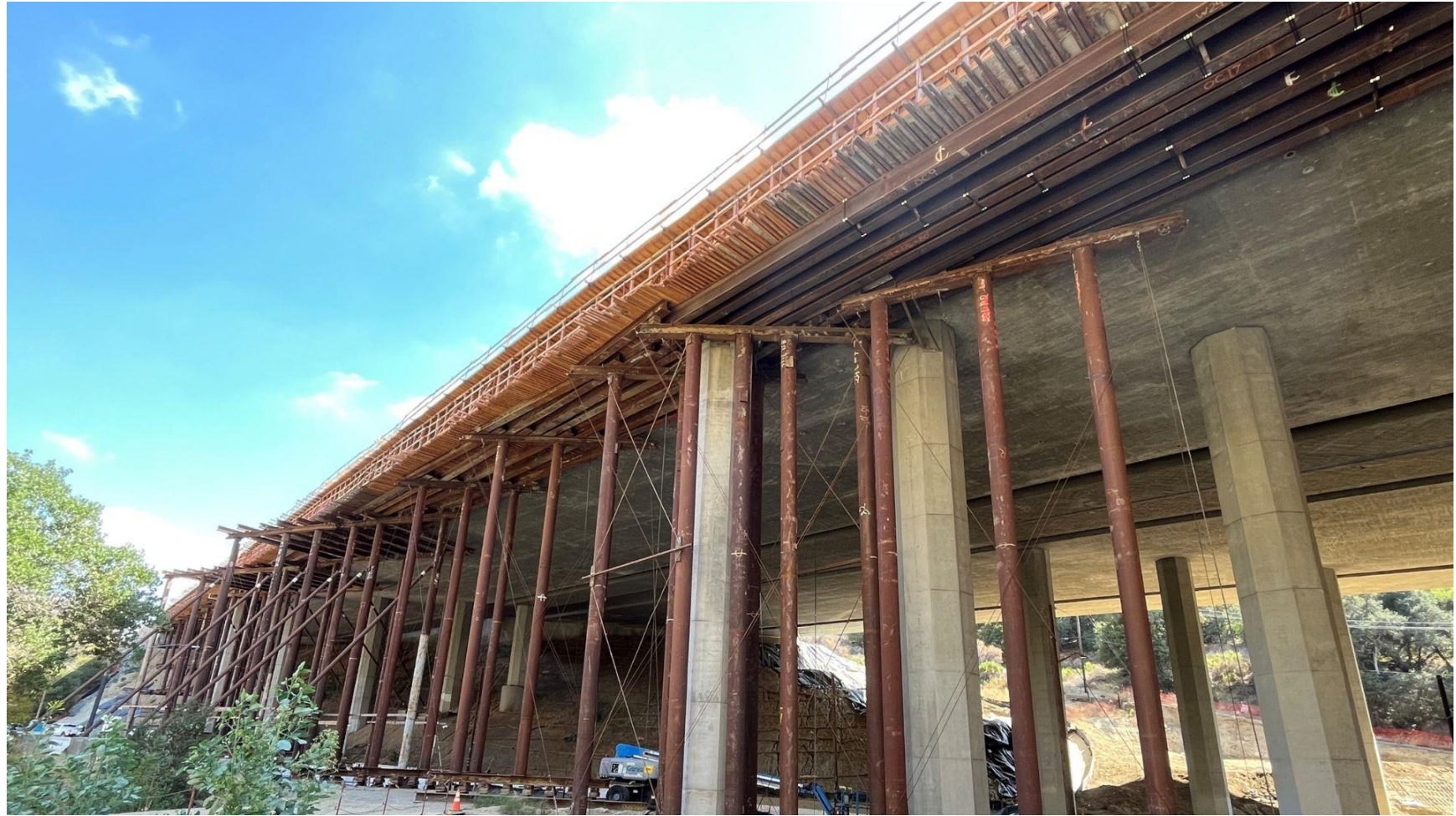
Gavin Canyon Bridge falsework construction – October 2025
