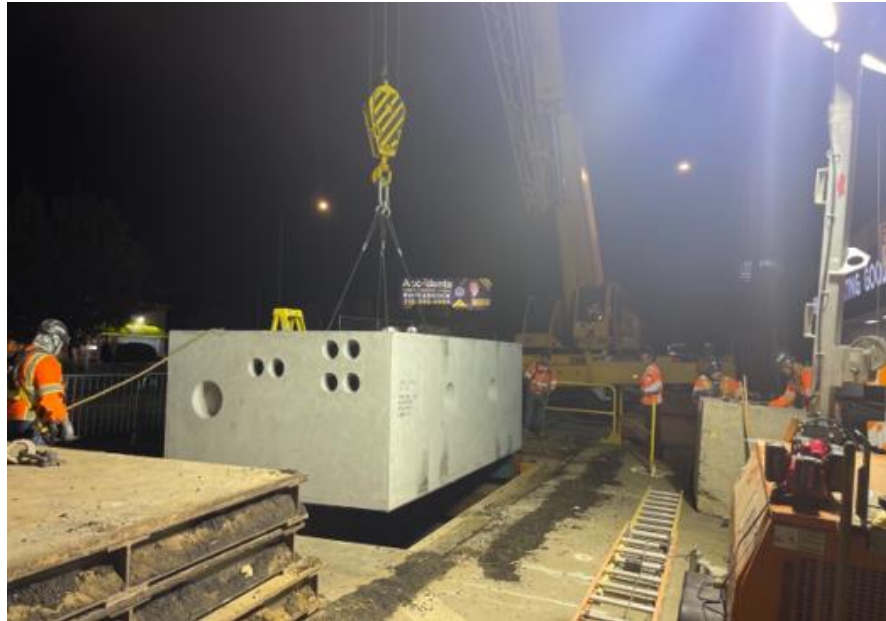
Vault installation on Van Nuys Bl and Wyandotte St
