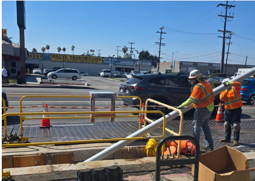
Conduit installation work at Van Nuys Bl and Keswick St
