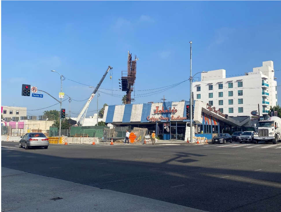
FIGURE 3.2-5. LU-3, PHOTO #3: WILSHIRE/FAIRFAX STATION ENTRANCE, NORTHWEST ENTRANCE (EXISTING VIEW, FACING NORTHWEST)
