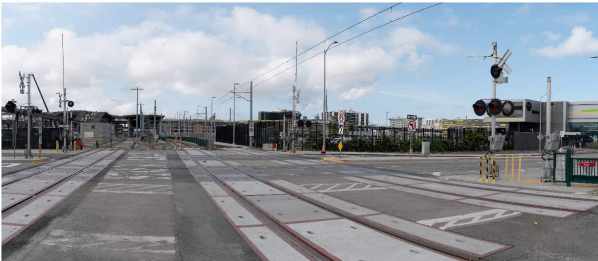
FIGURE 3.2-15. LU 13, PHOTO #13: MSF – EXPANSION OF DIVISION 16 YARD, BETWEEN ARBOR VITAE STREET ON THE NORTH AND 96 TH STREET ON THE SOUTH (EXISTING VIEW, FACING SOUTH)
