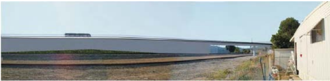
18b-3 With Retaining Wall and Embankment
