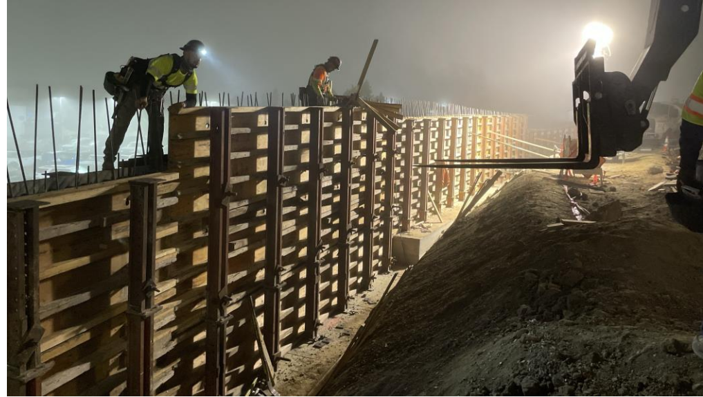
Retaining wall formation of South St SB off-ramp
