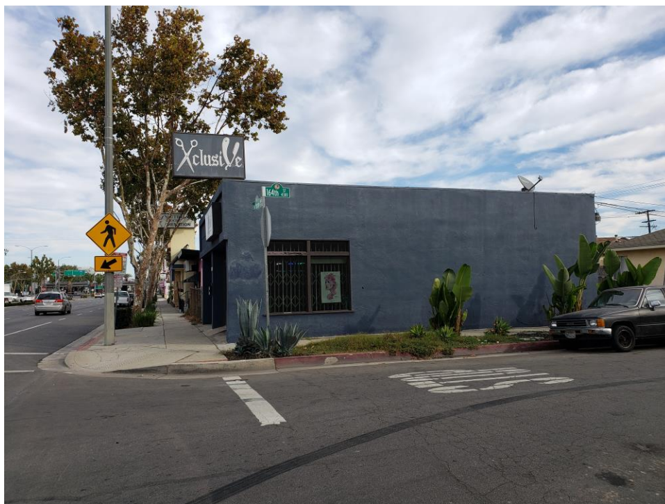
Photograph 2. South elevation, view to north, November 5, 2020
