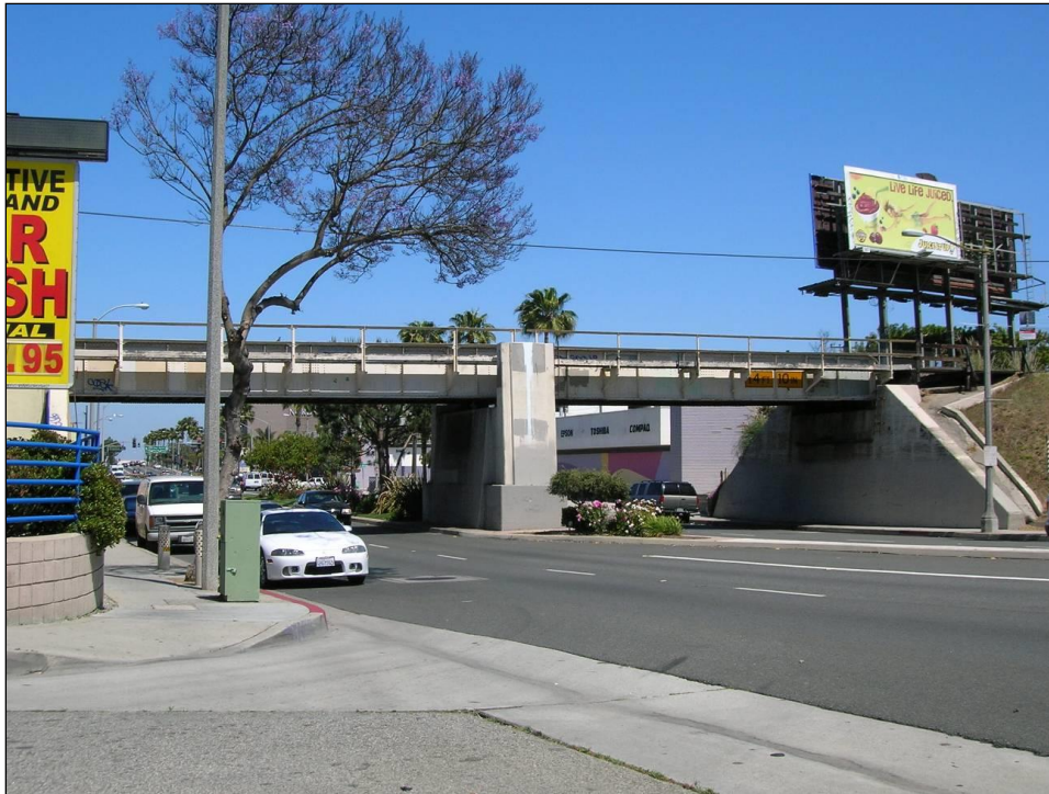
Photograph 4. Harbor Subdivision – Artesia Boulevard Bridge, view to east, AECOM 2010.
