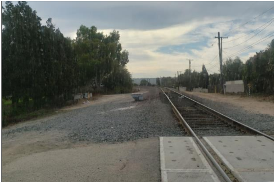
Photograph 2. Harbor Subdivision – Tracks through Lawndale, view to north, November 5, 2020.
