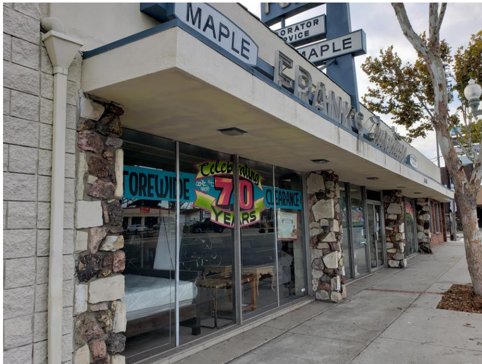
Photograph 2. Detail of west elevation façade, view to southeast, November 5, 2020
