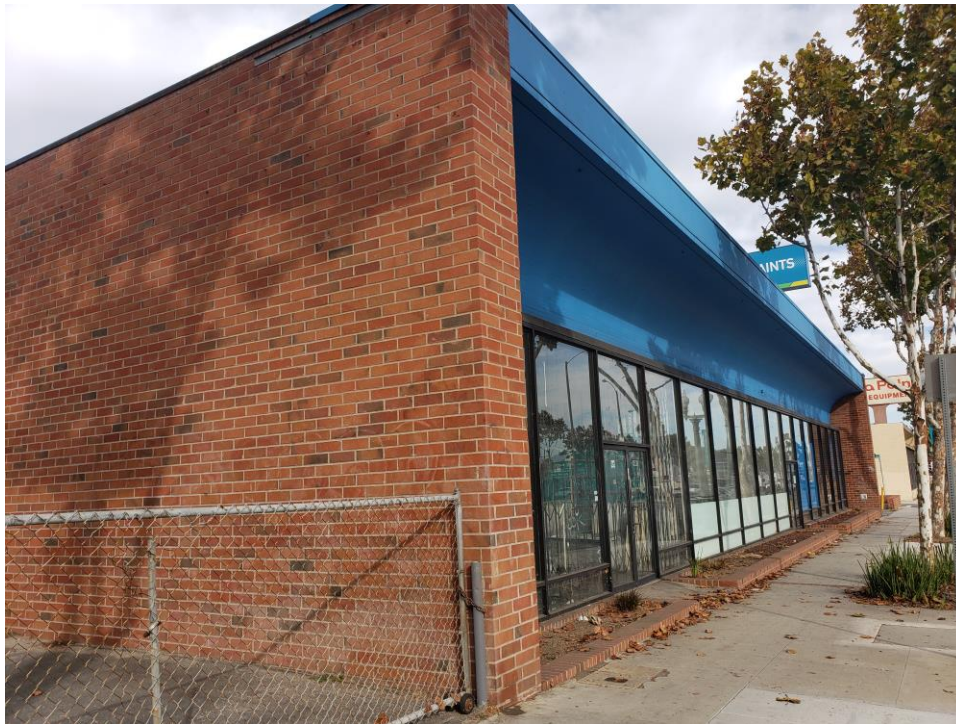
Photograph 2. South and east elevations, view to northwest, November 5, 2020
