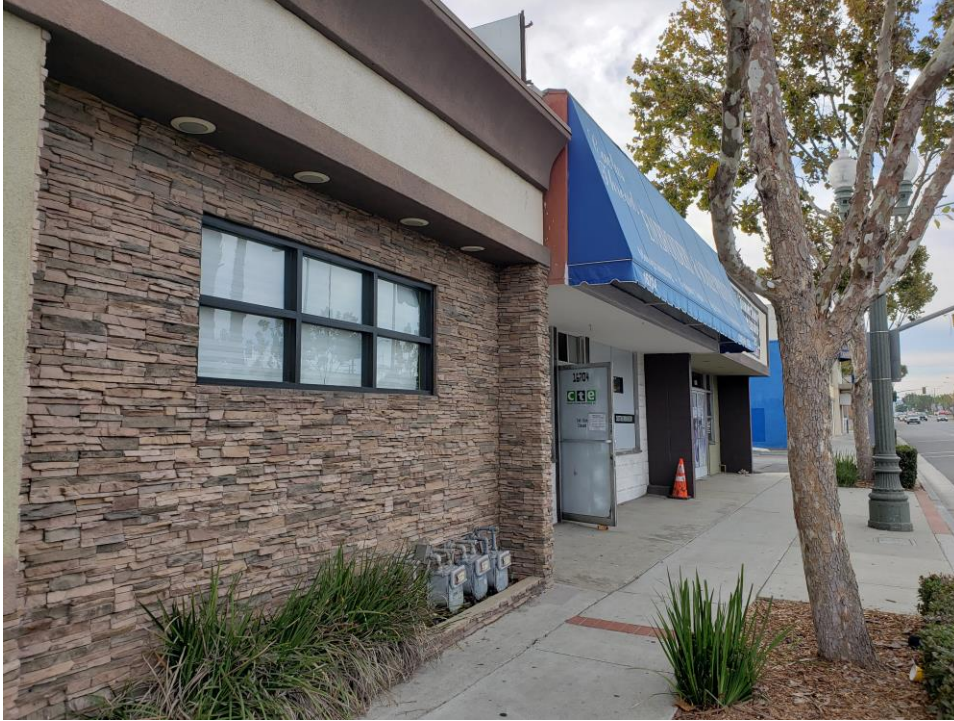
Photograph 2. Detail of façade, view to southeast, November 5, 2020
