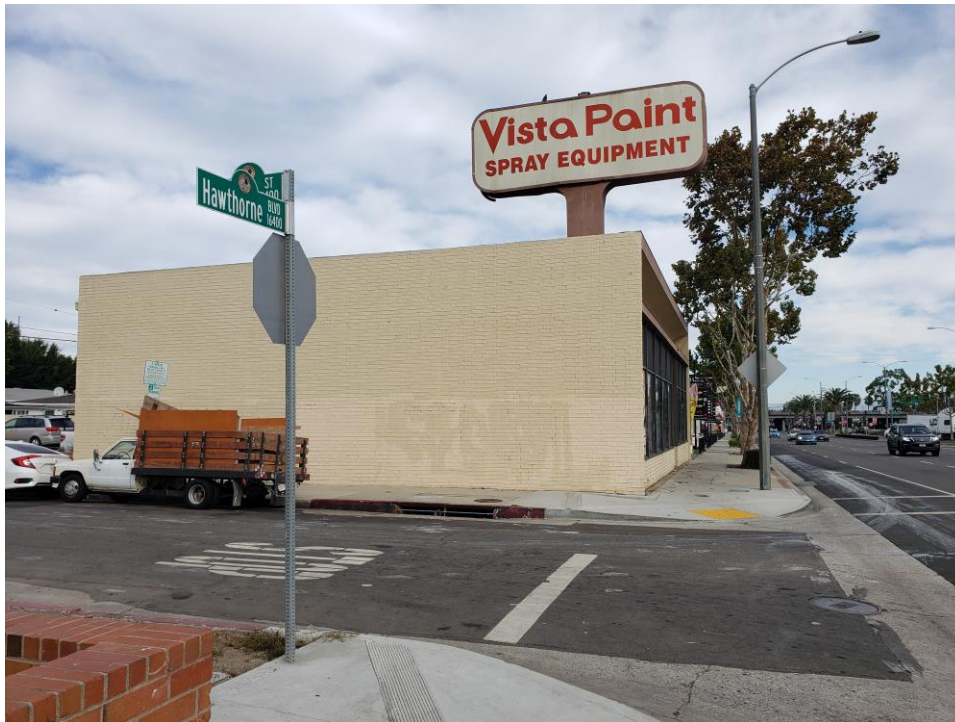
Photograph 2. South elevation, view to north, November 5, 2020
