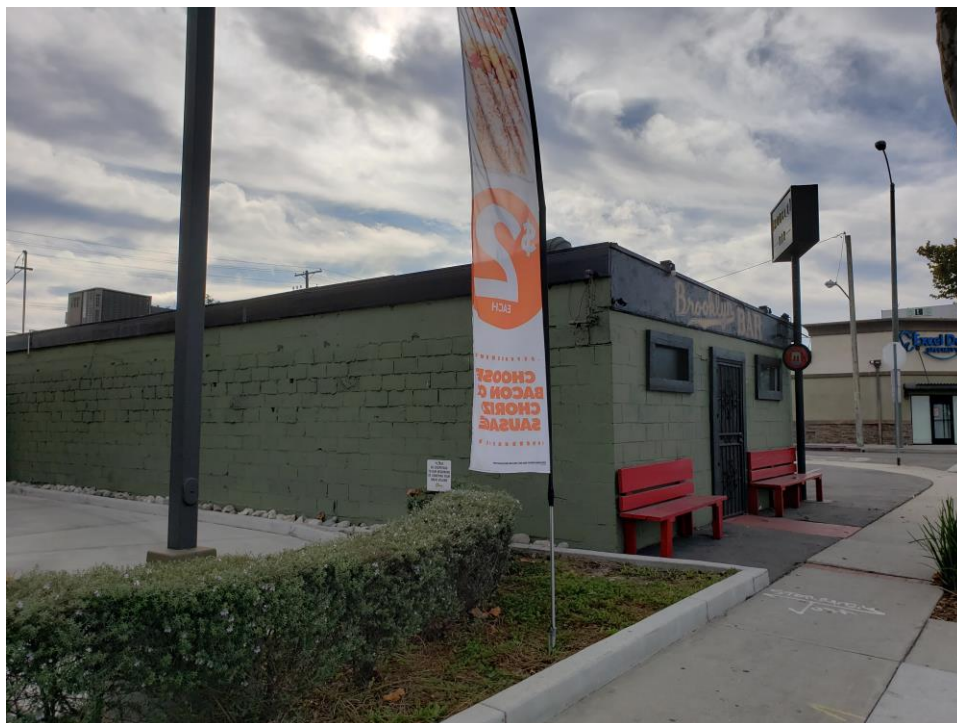
Photograph 2. North and west elevation, view to southeast, November 5, 2020
