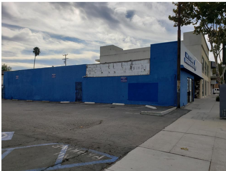
Photograph 2. North elevation and façade, view to south, November 5, 2020
