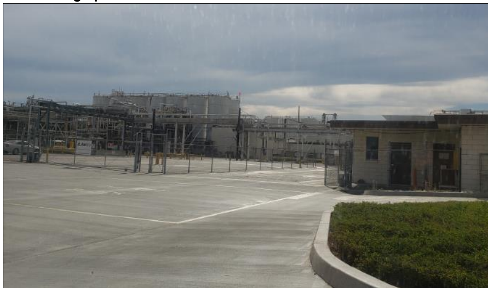
Photograph 1. Dow Chemical Plant, 305 Crenshaw Boulevard, Torrance, November 5, 2020.
