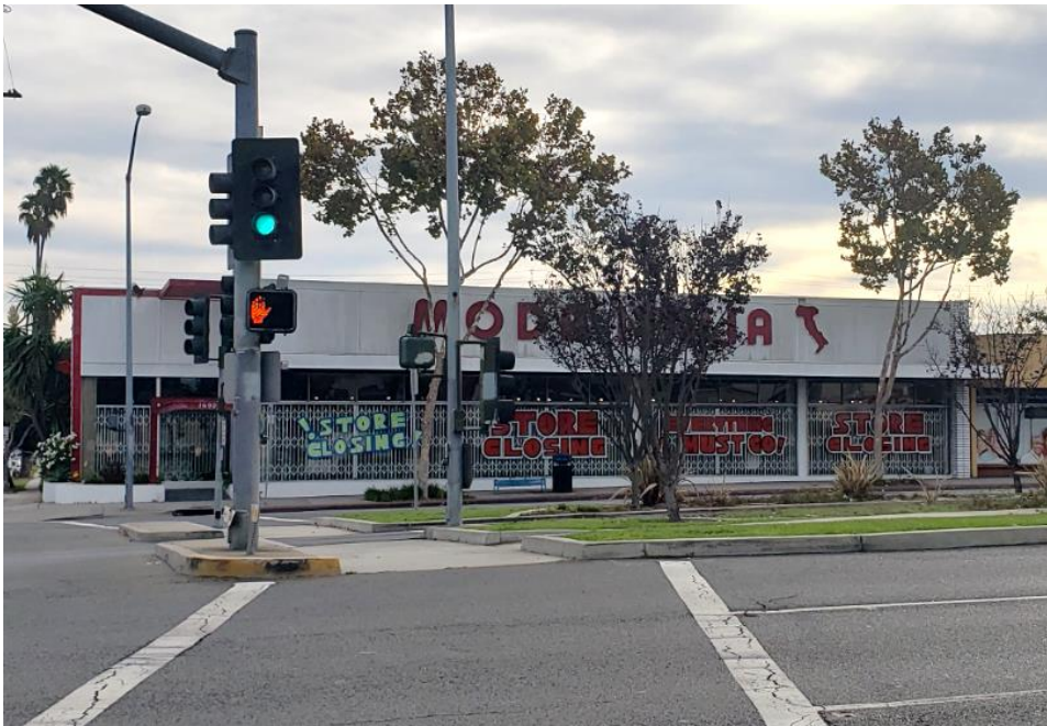
Photograph 2. West elevation, view to east, November 5, 2020
