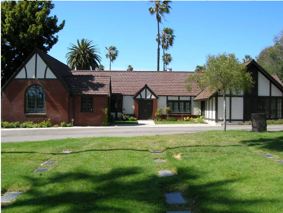
Photograph 3. Pacific Crest Cemetery – Chapel (c. 1934) and addition (c. 1960s), view to north, AECOM 2010
