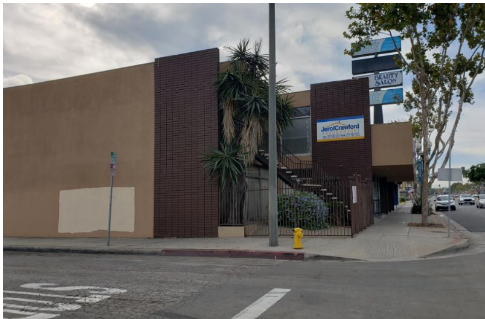
Photograph 2. North and west elevations, view to south, November 5, 2020
