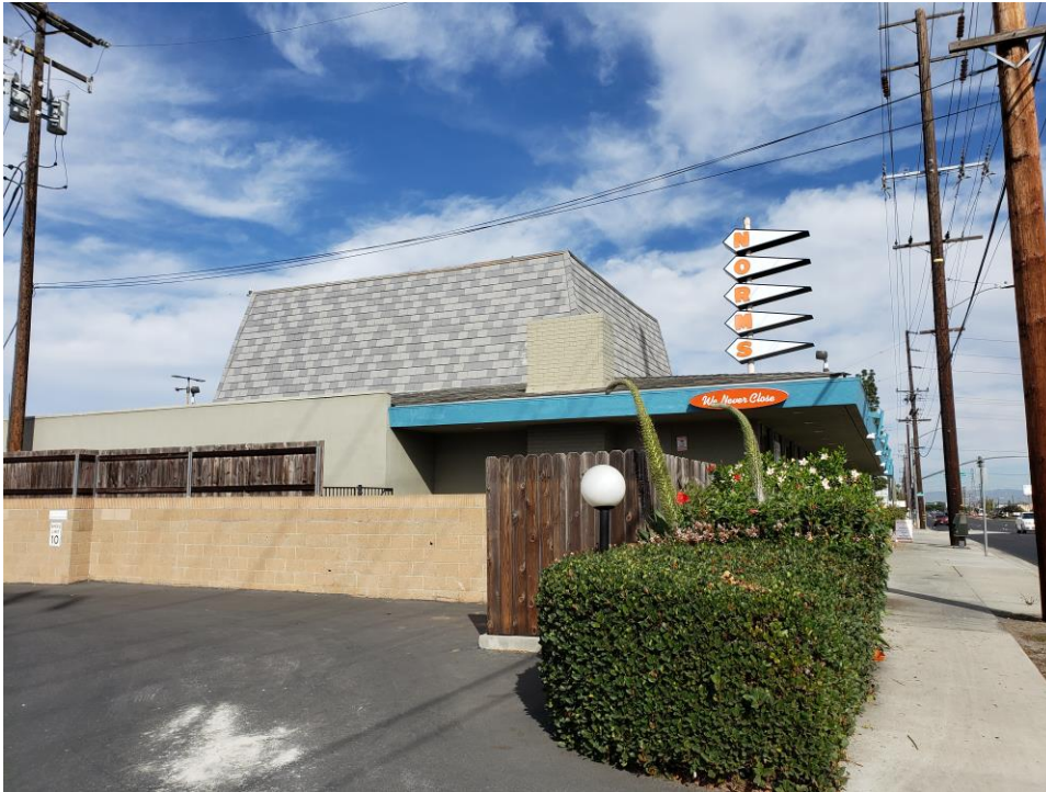
Photograph 2. South elevation rear addition, view to north, November 5, 2020
