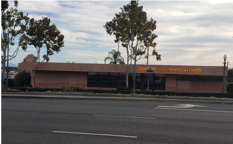
Photograph 2. West elevation, view to east, November 5, 2020
