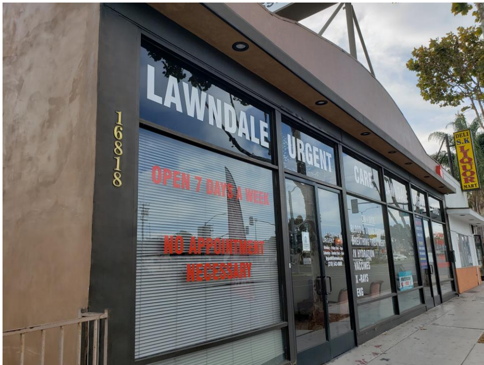
Photograph 2. Detail view of façade, view to east, November 5, 2020
