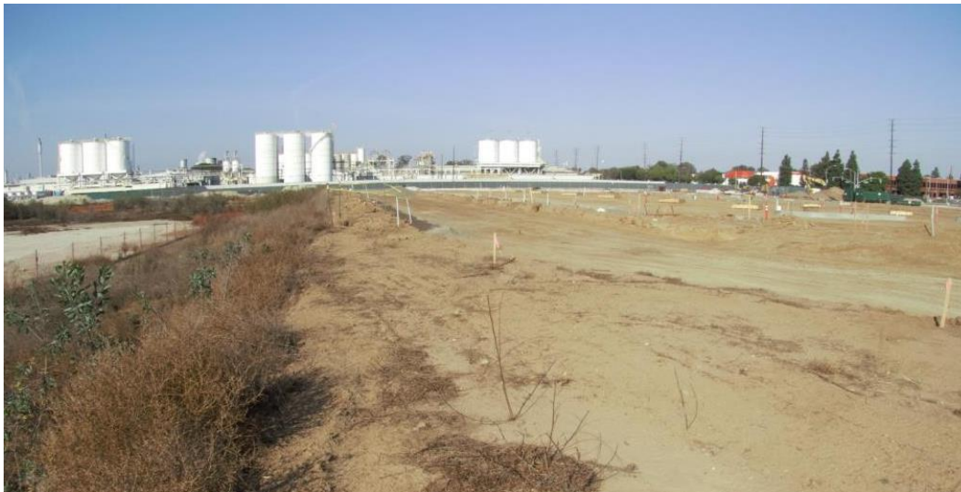
Figure 3.7-13. Proposed laydown area adjacent to the Open Space Preserve (Torrance TC); facing north
