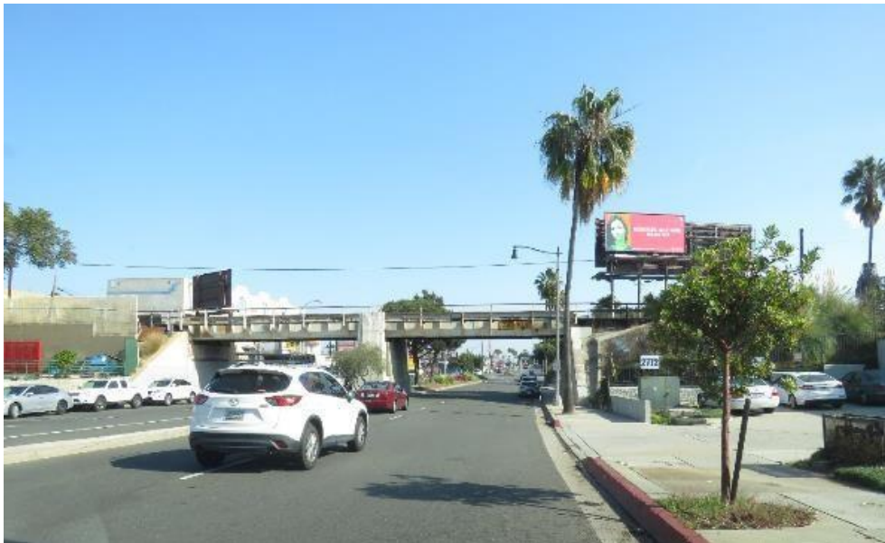
Figure 3.7-11. Existing freight bridge in Metro ROW, crossing over Artesia Boulevard; facing west
