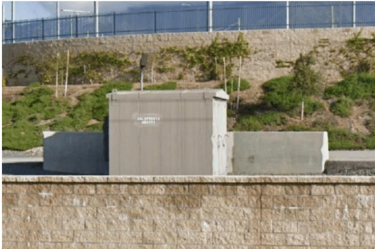
Figure 2.3-35. Typical Train Communications and Signaling Building
