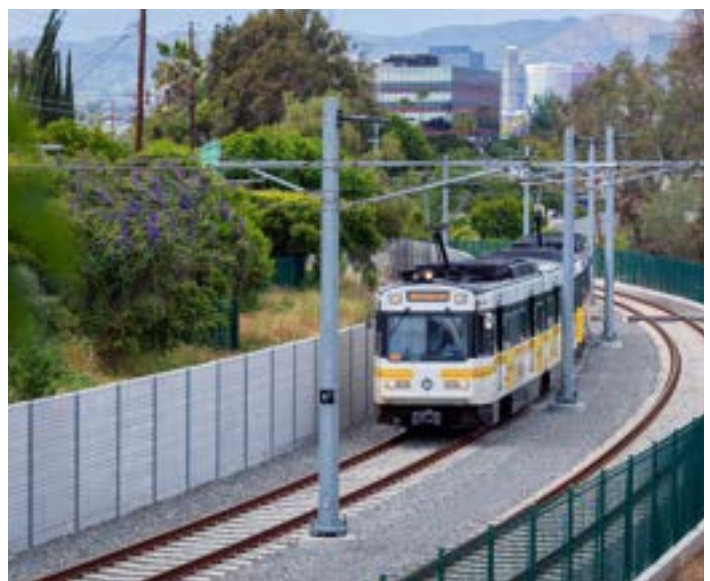
Example of a light rail train (Metro E Line) traveling alongside soundwalls through a neighborhood.
