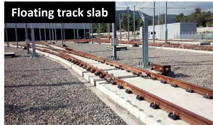
Floating track slab
