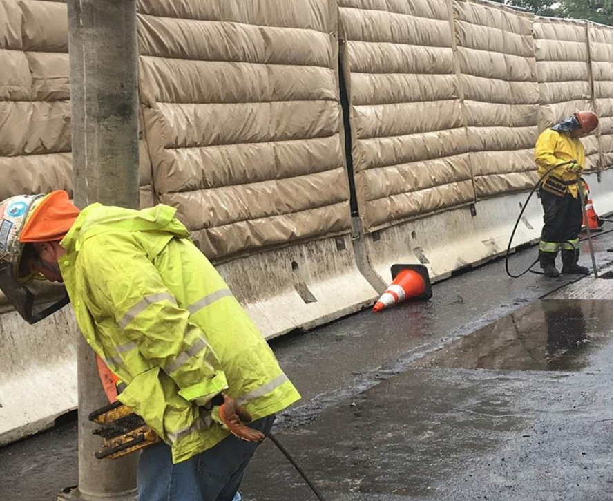
Temporary Noise Barriers
