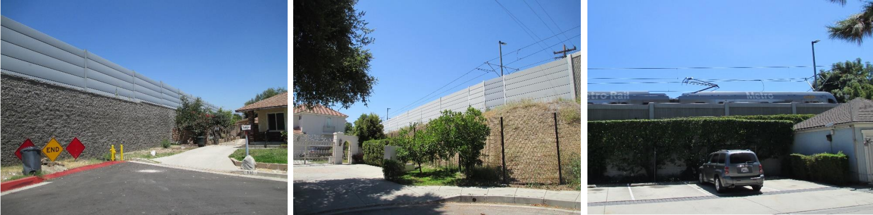
Solid Privacy Panels over soundwall
