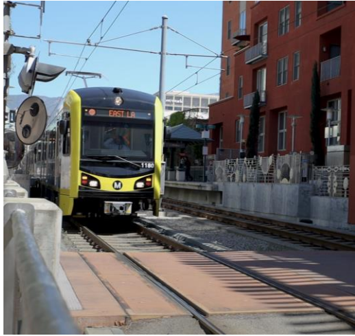
Overhead Catenary System Poles
