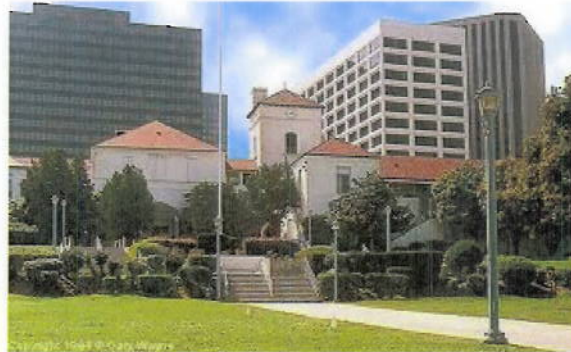
Figure 5 - Stair access to Buildings B from S. Moreno Drive.
