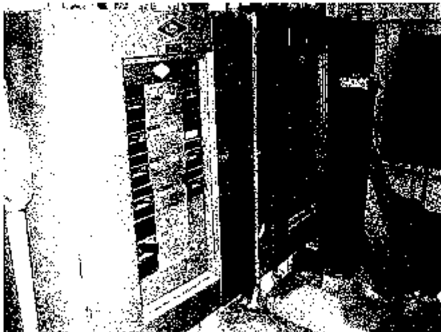
Bldg C, Rm 158: Switch boards "MSP-1" 600A, 240V, 3ph, 3w; "MSA", "MSB", "MSC": 600A, 120/240V, 1ph, 3w.
