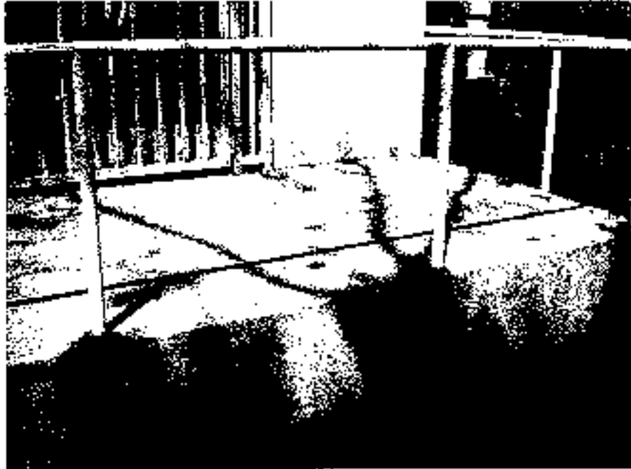
Handrail at entrance along Rexford Drive shows signs of corrosion at base of posts. Repair is required.
