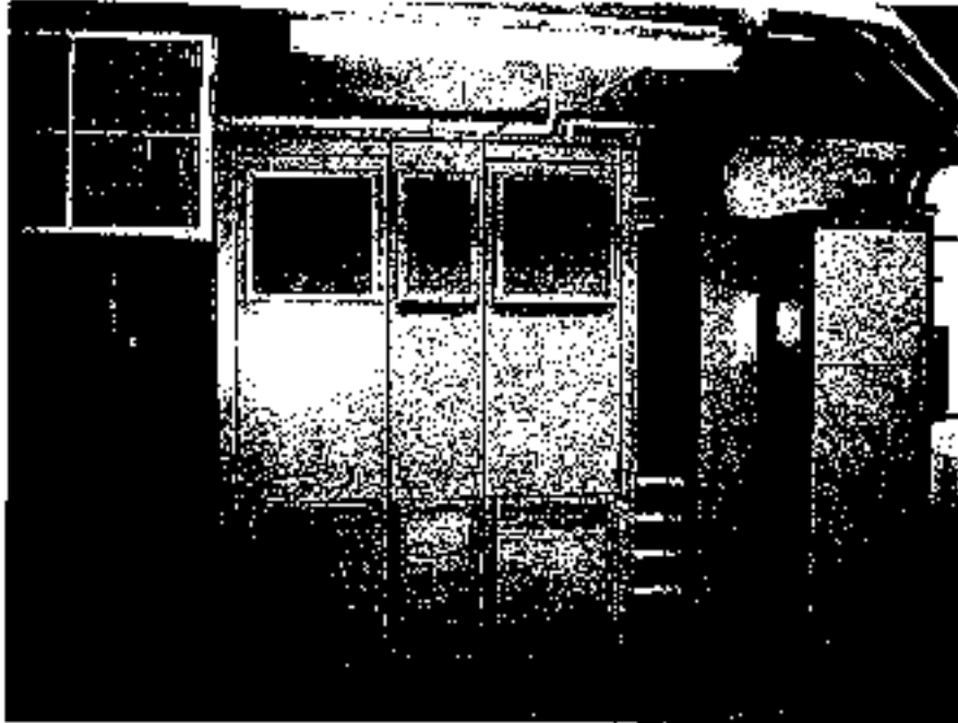
Existing MGM - 1000KVA - 4160V = 277/480V Stepdown Transformer - In Electrical Room Serving Dist. Board "AA"
