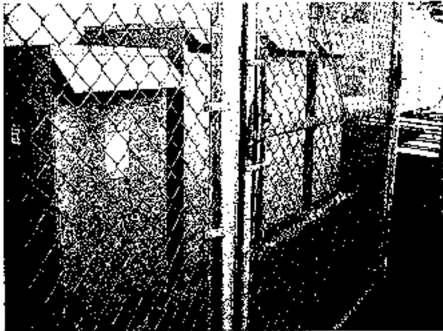
Bldg. C, Rm 158: Distribution board "EMS" 1600A, 240V, 3ph, 3w.
