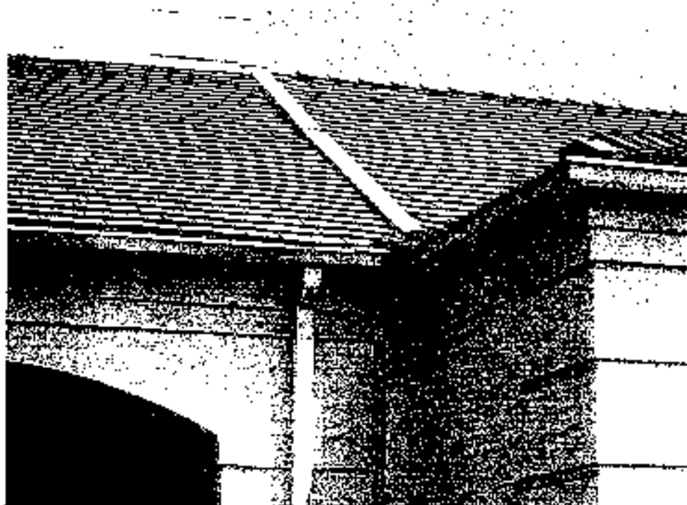
Photo 17: Seismic joint
