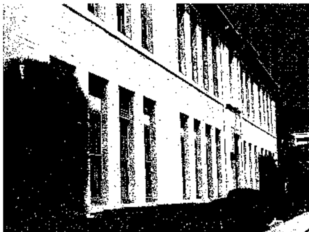
Photo 13: Classroom north elevation
