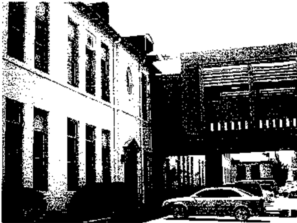
Photo 22: Classroom bridge at south elevation
