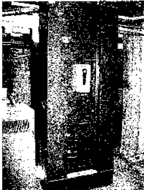
Replace Distribution Board- 1200A, 120/240V, 1ø (E-4A)
