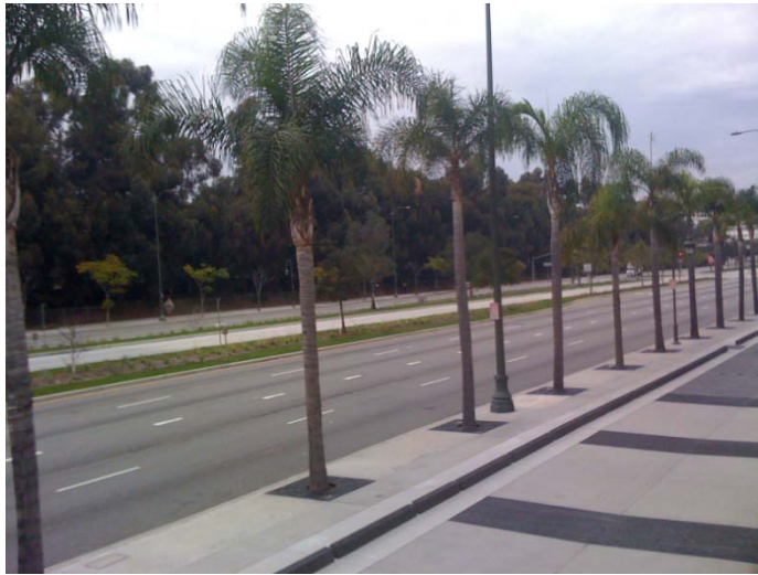
Photograph 3 – Santa Monica Boulevard Busway looking northeast
