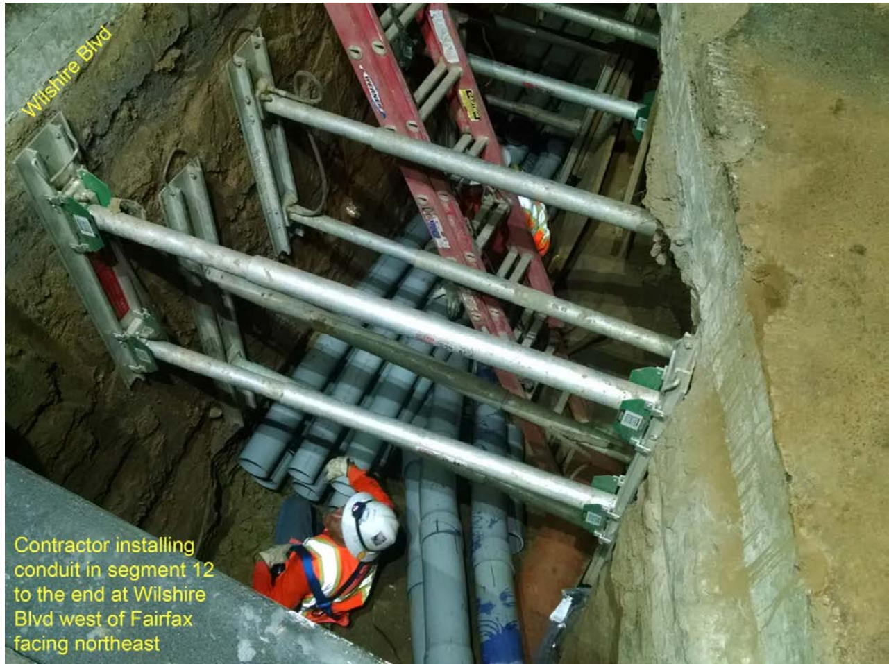
C1055 Contractor Installing Power Conduit near Wilshire/Fairfax Intersection
