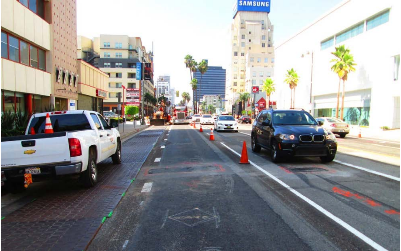
C1055 Contractor Performing Utility Relocations in Eastbound Wilshire Boulevard Traffic Lanes
