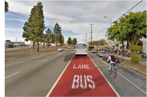
Side Running BRT – south of Gage
