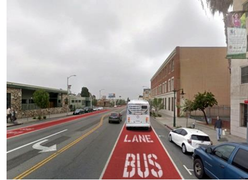
Side Running BRT – north of Gage
