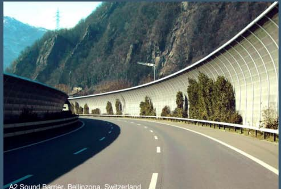
A2 Sound Barrier, Bellinzona, Switzerland
