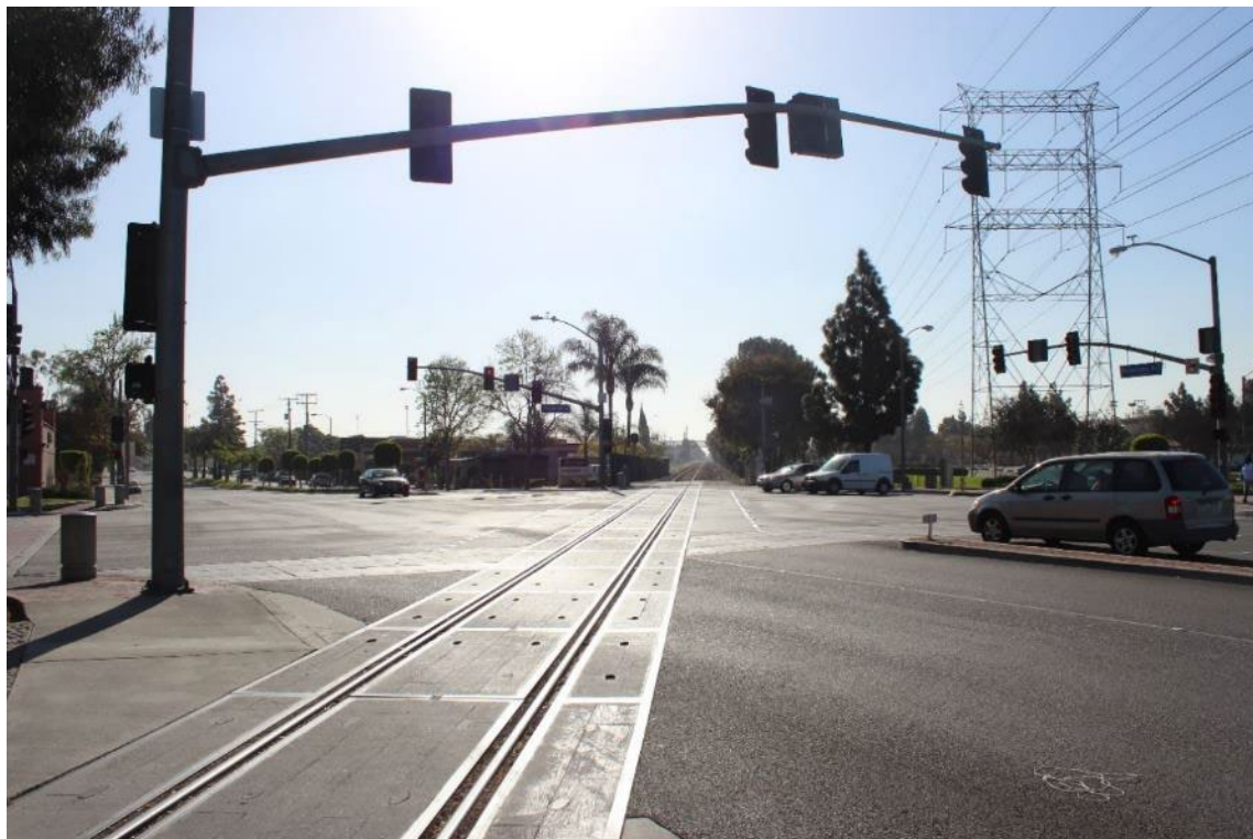
Figure 1-3. Existing Paramount Boulevard and Rosecrans Avenue At-Grade Train Crossing
