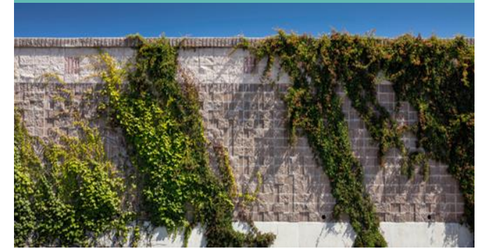
Sound Wall Improvements
