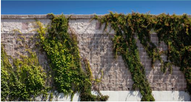
Sound Wall Improvements
