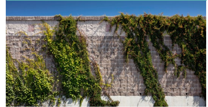
Sound Wall Improvements
