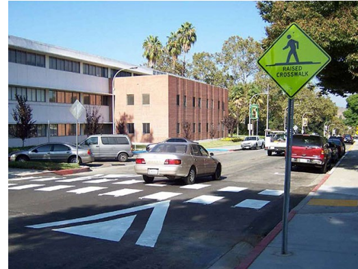
Raised pedestrian crossing
