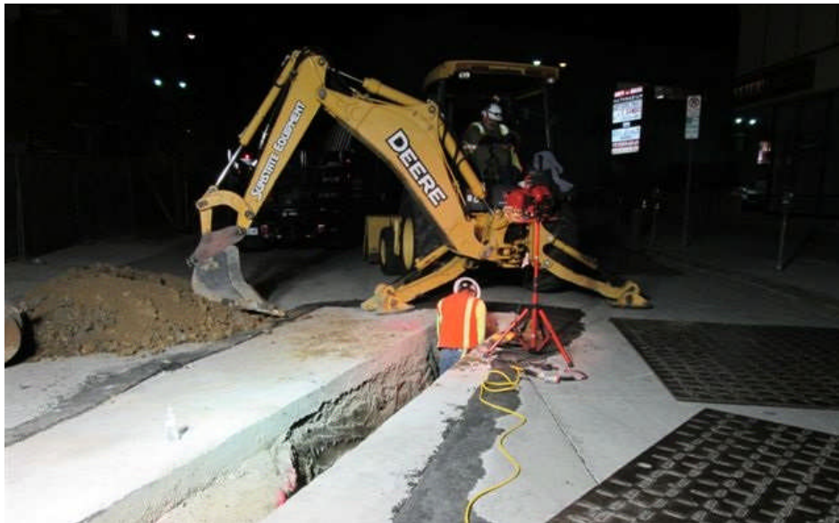
Utility potholing on Sycamore Avenue
