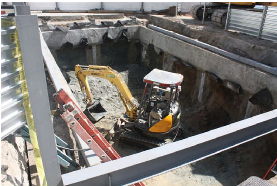
Intrinsically Safe Excavator inside the Exploratory Shaft
