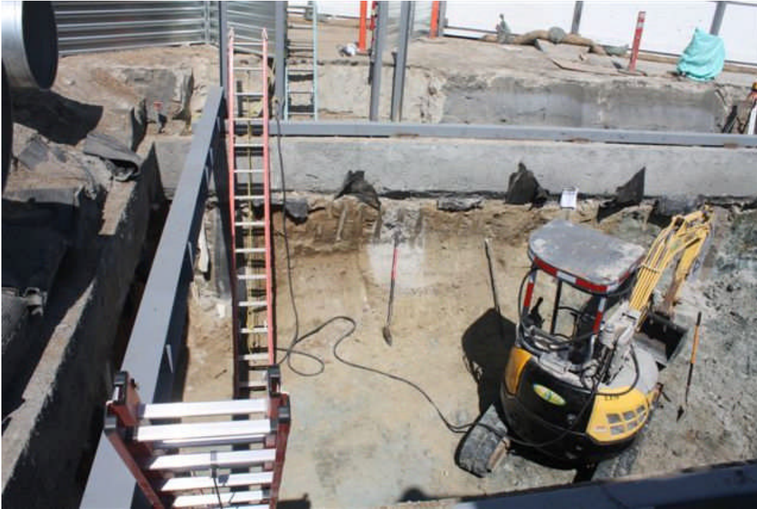
Shotcrete on West and North Walls of the Exploratory Shaft
