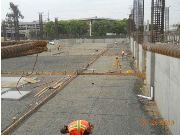
Slab on grade rebar installation on Parking Building.
