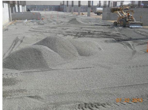
Gravel base for slab on grade on Parking Building.
