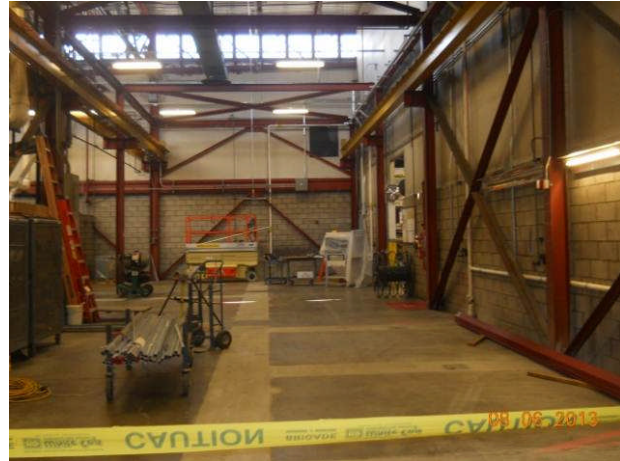
SOG refill and electrical work at new Radiator Shop
