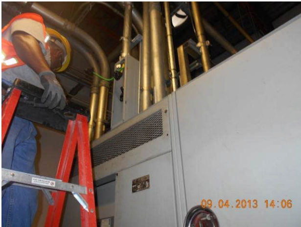
Connecting to main electrical control panel at Radiator Shop.
