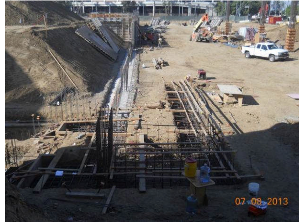
Concrete on wall foundation on Maintenance Building.
