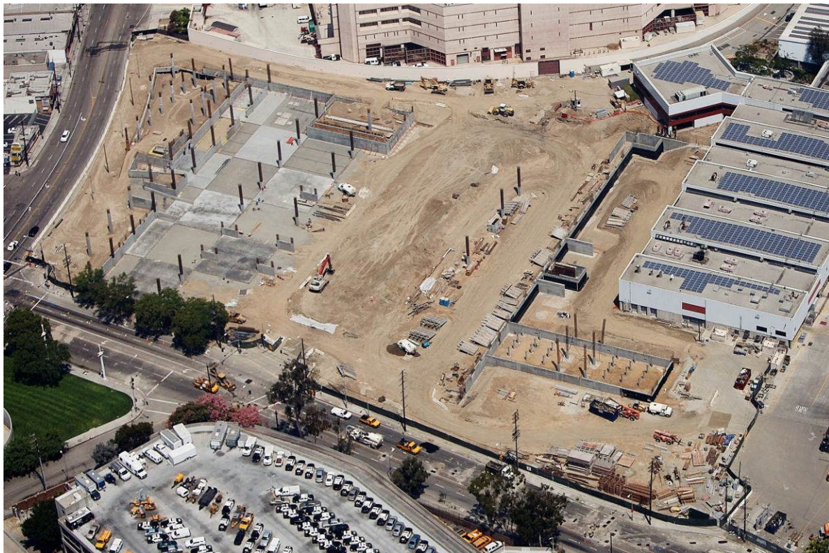
Transportation Building, Parking Garage and Maintenance Building in construction; at the bottom side Cesar Chavez Avenue and at the left side Vignes Street – August 2013.
