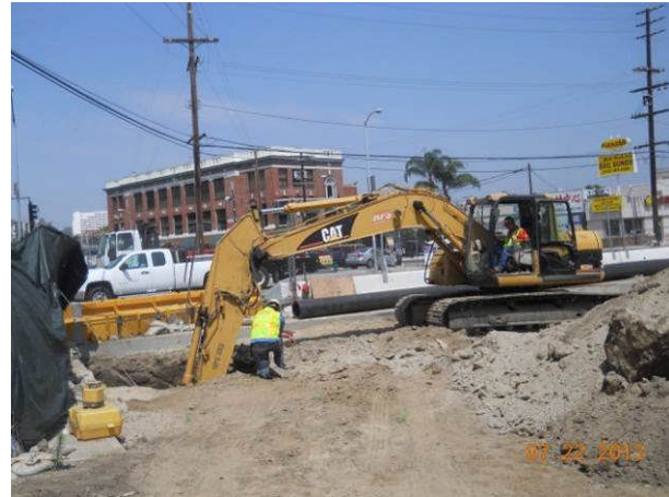
MH excavation on Vignes and Cesar Chavez intersection.
