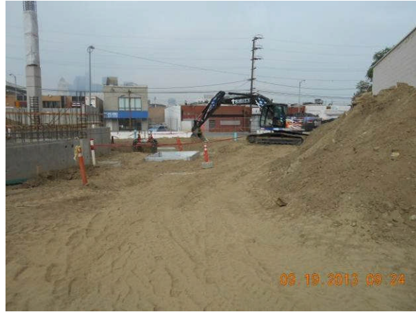
Storm water jellyfish excavation on Metro Driveway.
