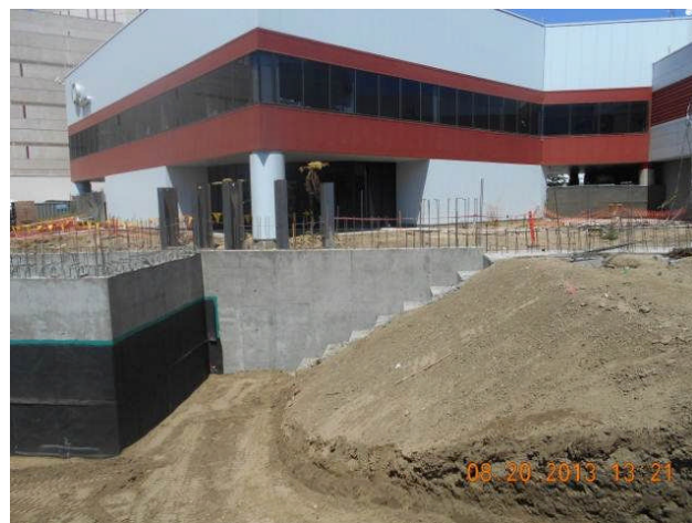
Outside wall waterproofing at Maintenance Building
