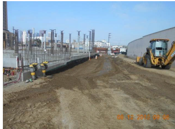
Filling and backfilling on Metro Driveway.
