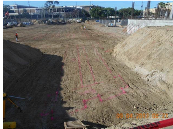
Foundations lay out on Area 5, 6 and 7 at Parking Garage.
