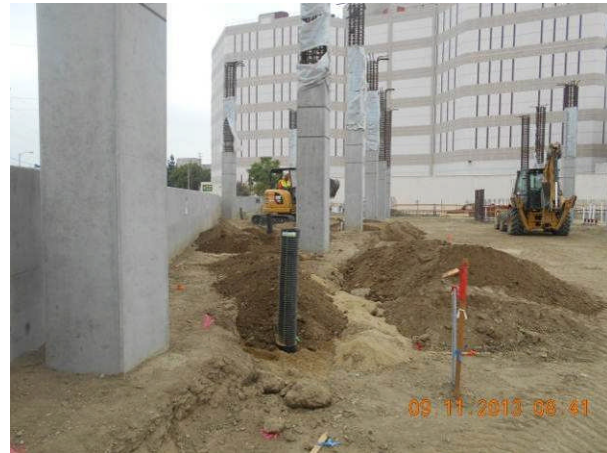
Storm drainage pipe installation at Transportation Bldg.
