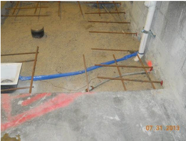
Rebar anchorage for SOG refill at new Radiator Shop.
