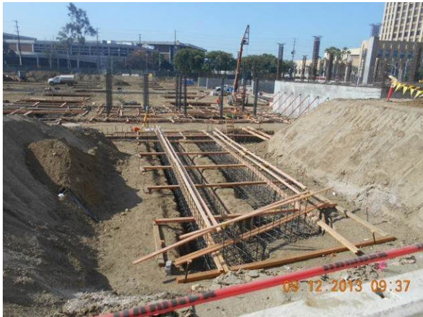
Tunnel and Area 5, 6 and 7 rebar installation at Building 2.
