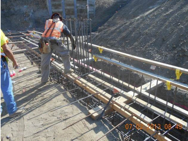
Wall foundation rebar on Maintenance Building.
