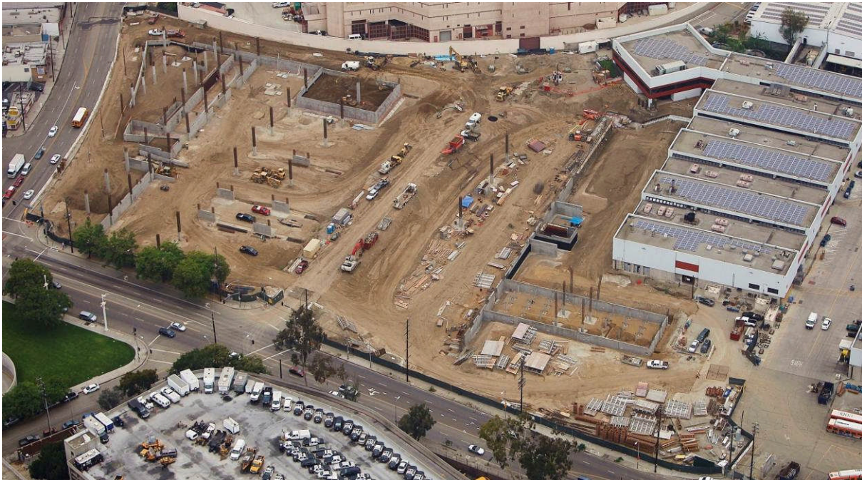
Transportation Building, Parking Garage and Maintenance Building in construction; at the bottom side Cesar Chavez Avenue and at the left side Vignes Street – July 2013.
