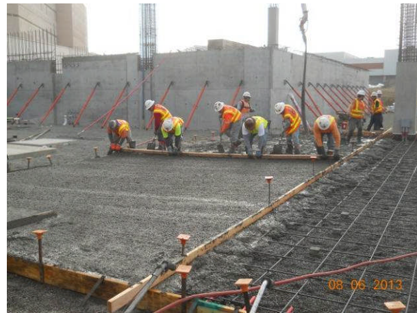
Slab on grade concrete placement on Parking Garage.
