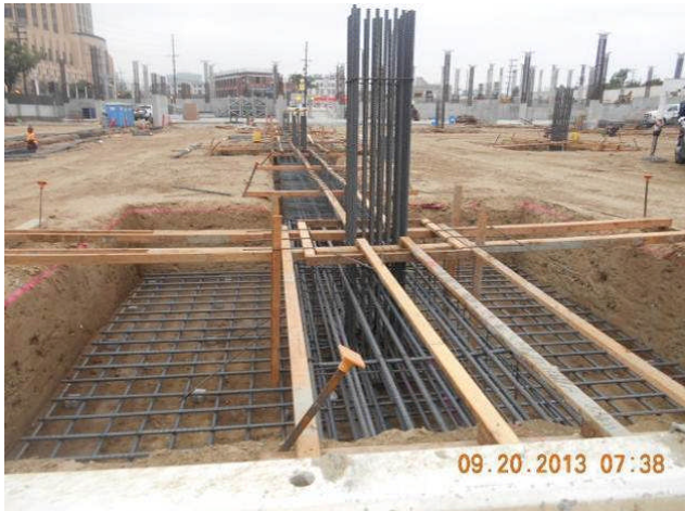
Area 5 and 8 columns and walls rebar installation at Park G
