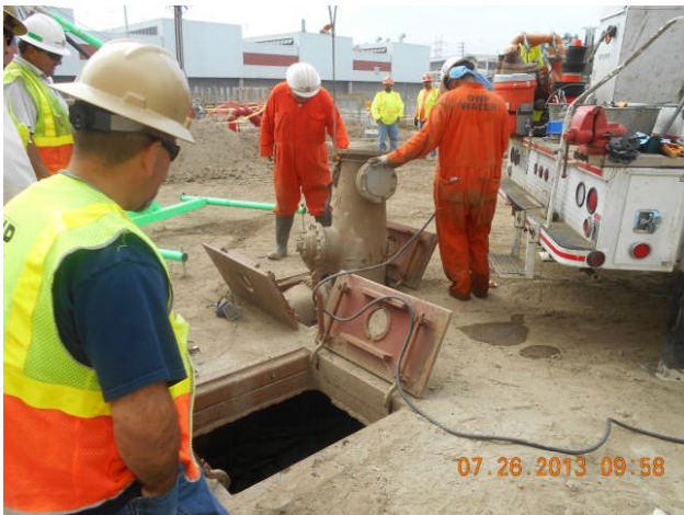
LADWP removing existing water pipe valve/meter on Metro Driveway.
