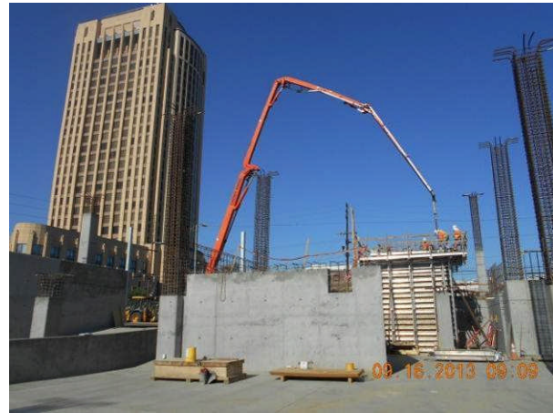
Elevator 1 concrete placement operation at Building 1.
