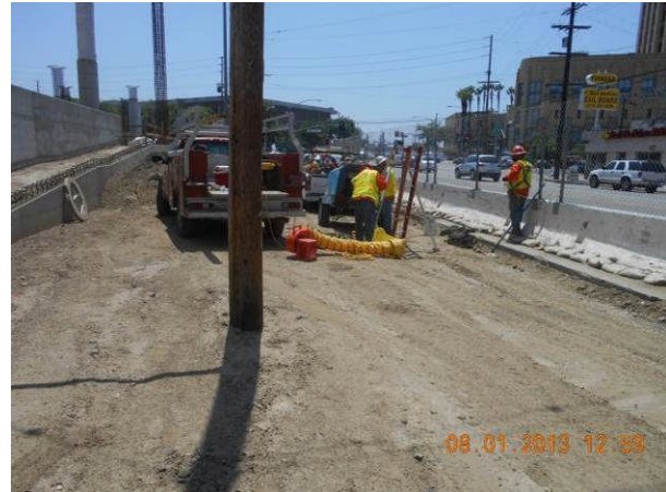
Contractor working on water meter vault at Vignes.
