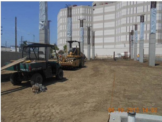
First level compacting and grading at Transportation Bldg.
