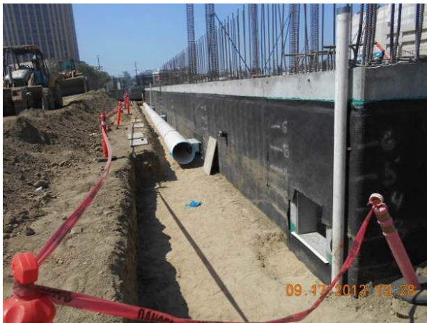
Underground mechanical ducts installation Maintenance Bldg.
