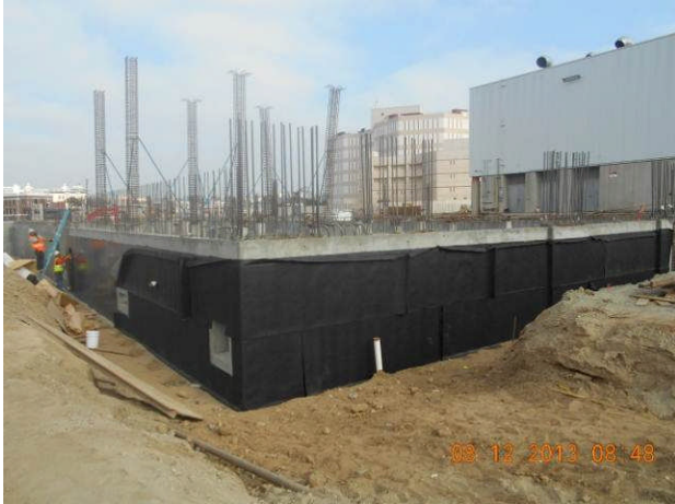
New waterproofing installation on Maintenance Building.
