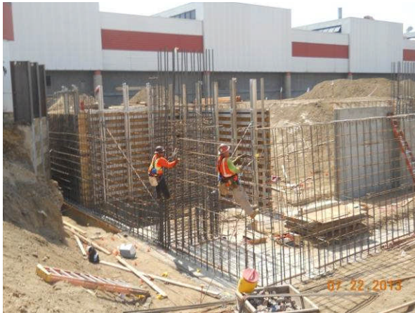
Wall rebar installation on Maintenance Building.
