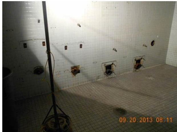
Existing rest rooms demolition/ removal at Radiator Shop
