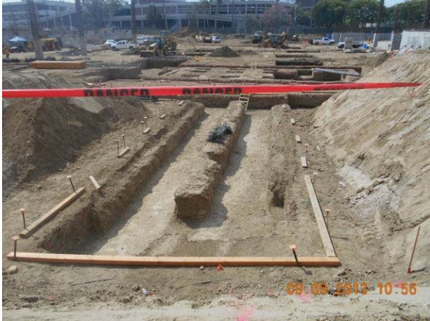
Foundation excavation Area 5, 6 and 7 at Parking Garage.
