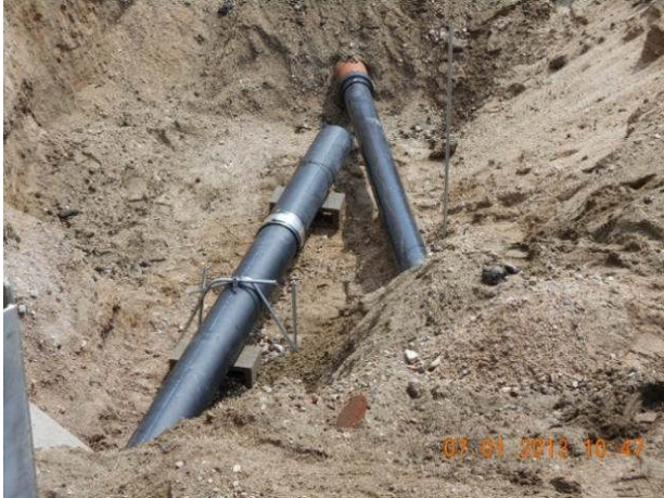
Provisional sanitary sewer piping.
