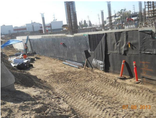
New waterproofing outside Parking Building walls.
