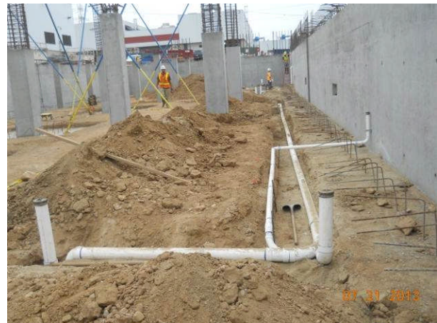
Drain pipe installation inside Parking Building.
