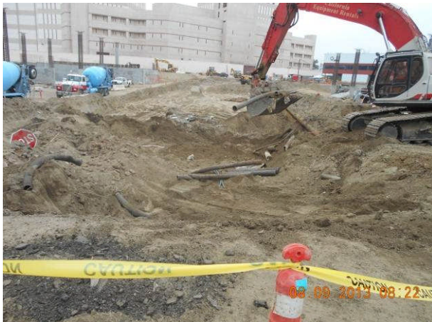
Existing pipes demolition and removal at Lyon Street.
