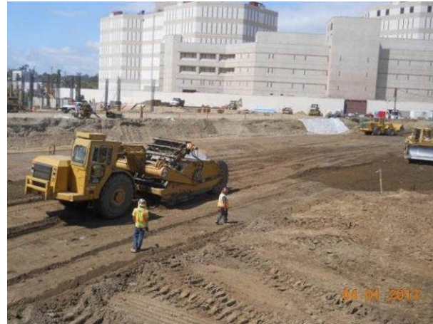
New storm drain pipe and existing pipe connection .
