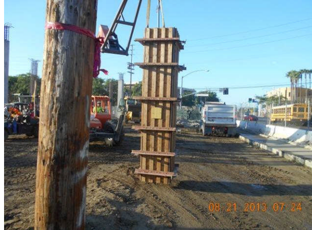
Moving columns forms to Transportation Building..
