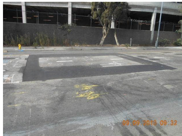
DWP electrical inspection vault on Cesar Chavez.
