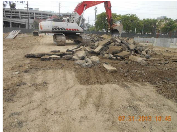
Pavement demolition and removal on Lyon Street.
