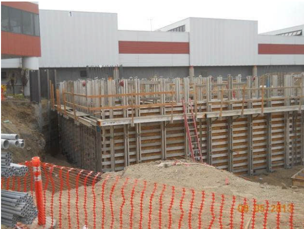
Gridline H shear wall form on Maintenance Building.
