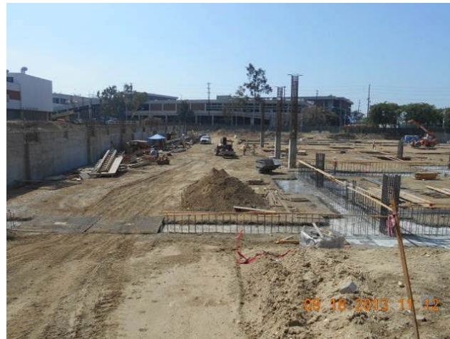
Foundations for columns and walls at Parking Garage.
