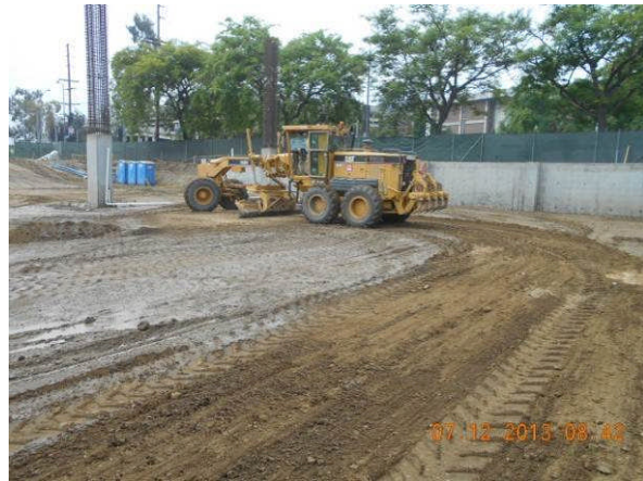
SOG fine grading operation on Parking Building.
