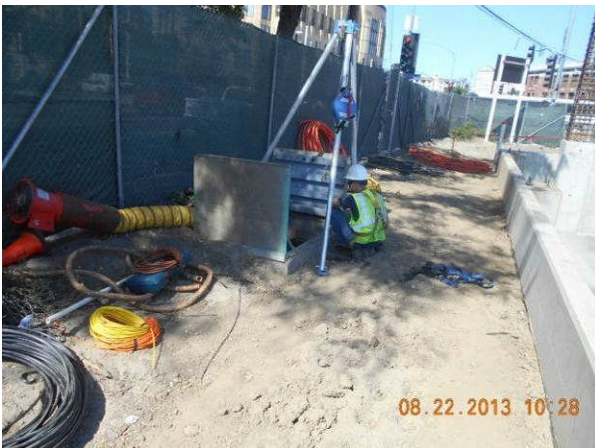
Fiber optic duct installation near Cesar Chavez Avenue.
