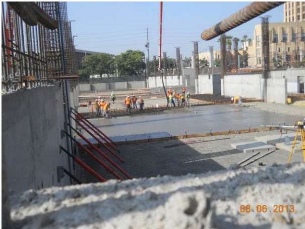
Slab on grade floating finish surface on Parking Garage.
