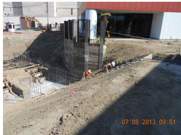
Wall foundation concrete placement on Maintenance Bldg.
