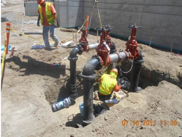
Water pipe RPP Devices installation on Metro Driveway.
