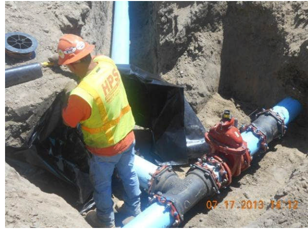
Water pipe valves installation on Metro Driveway.
