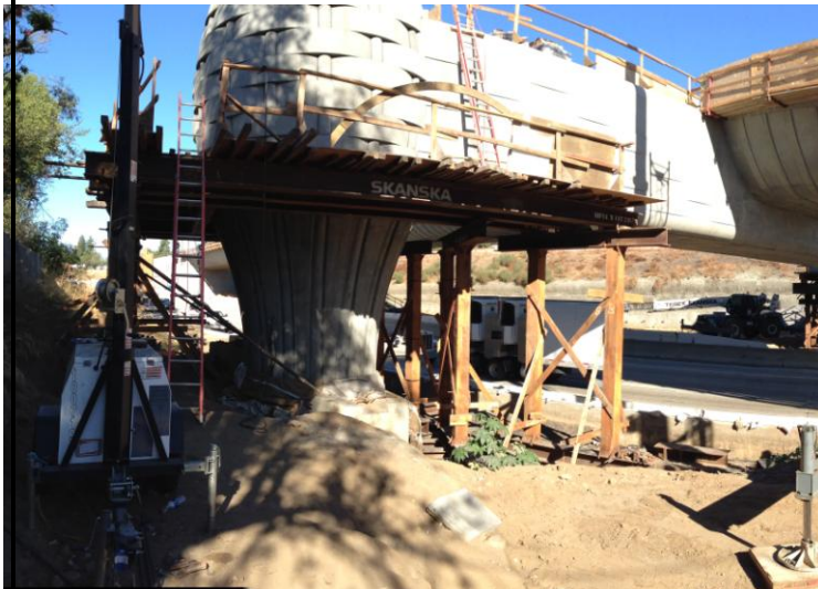
Median basket installation
