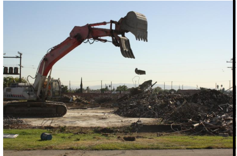
M&O Facility demolition
