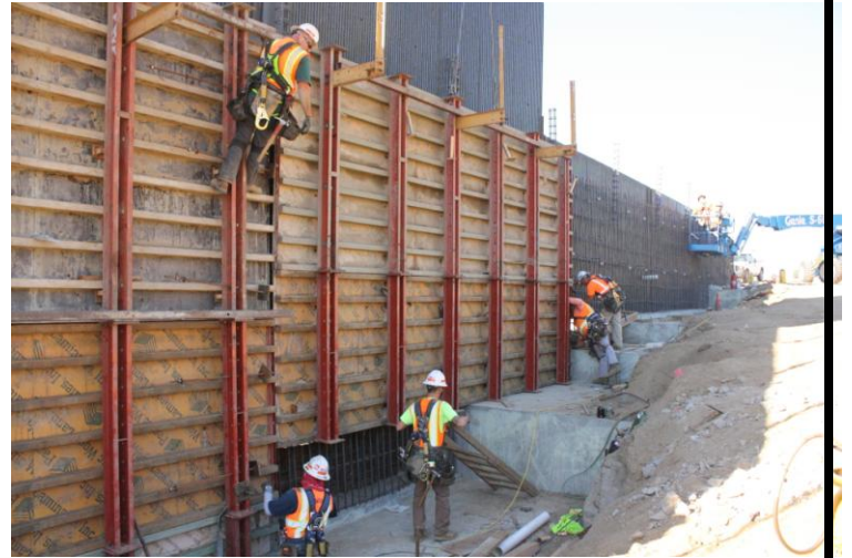
Construction of retaining walls
